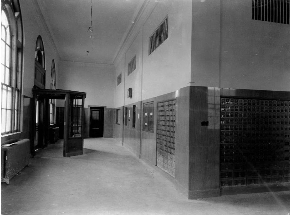
Figure 5: Bryan Federal Building and Post Office and Post Office, November 1939. Lobby interior looking east towards Postmaster office. Source: Property Owner.
