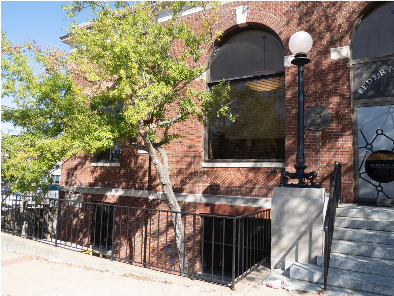
Photo 10: Primary (South) Elevation, View Northwest.
