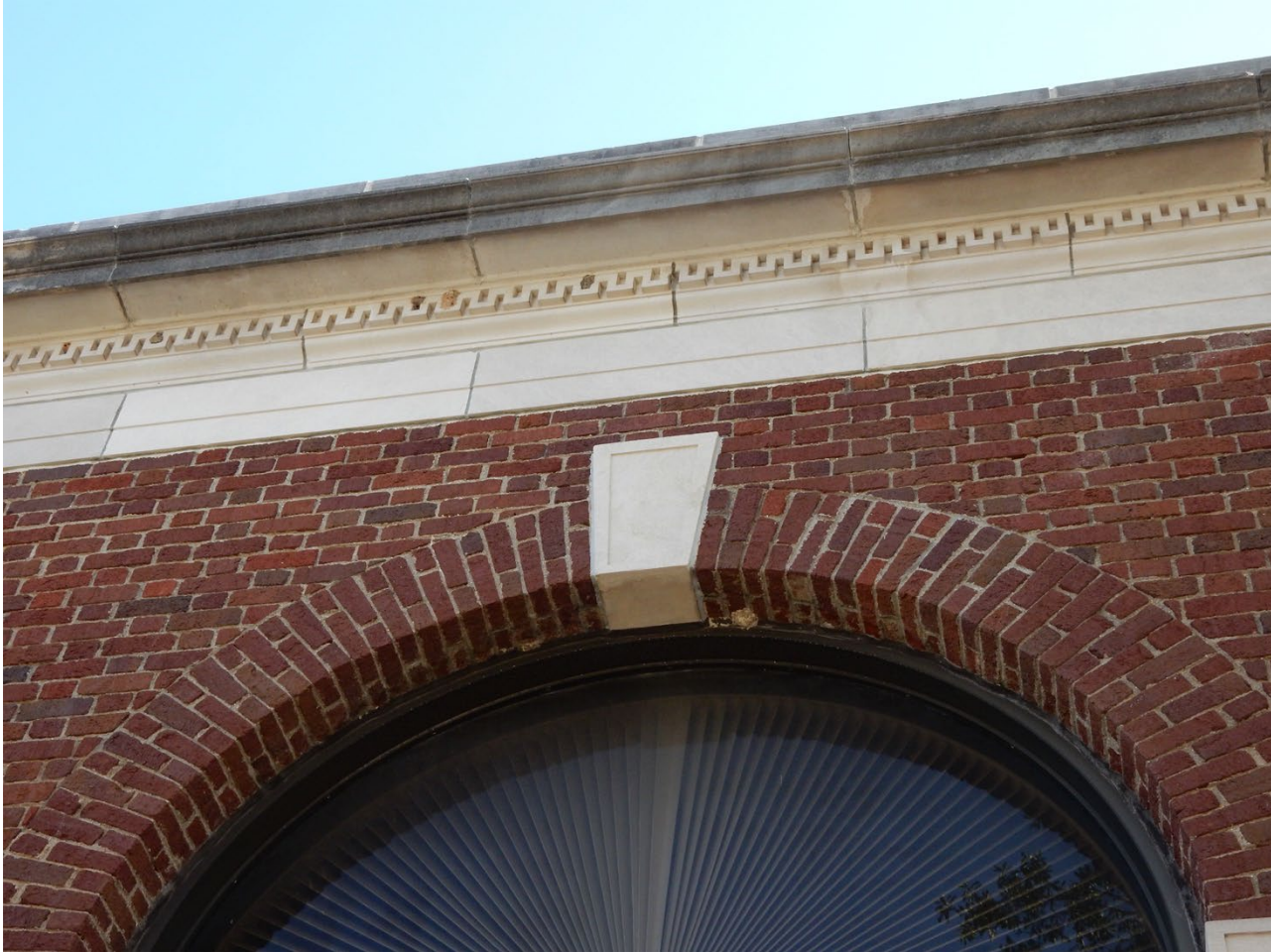
Photo 11: Primary (South) Elevation Masonry and Cornice Detail, View North.
