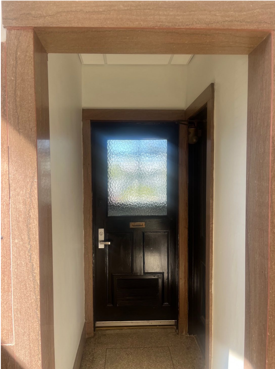
Photo 14: Main Level, Postmaster Office Entrance, View West.
