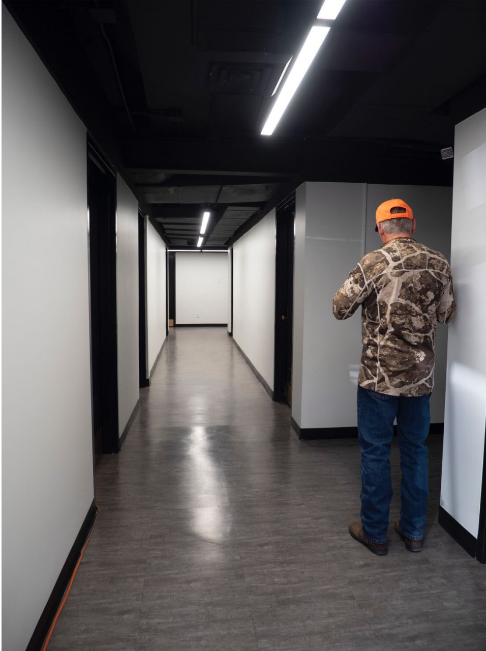
Photo 20: Lower Level, Central Corridor, View West.
