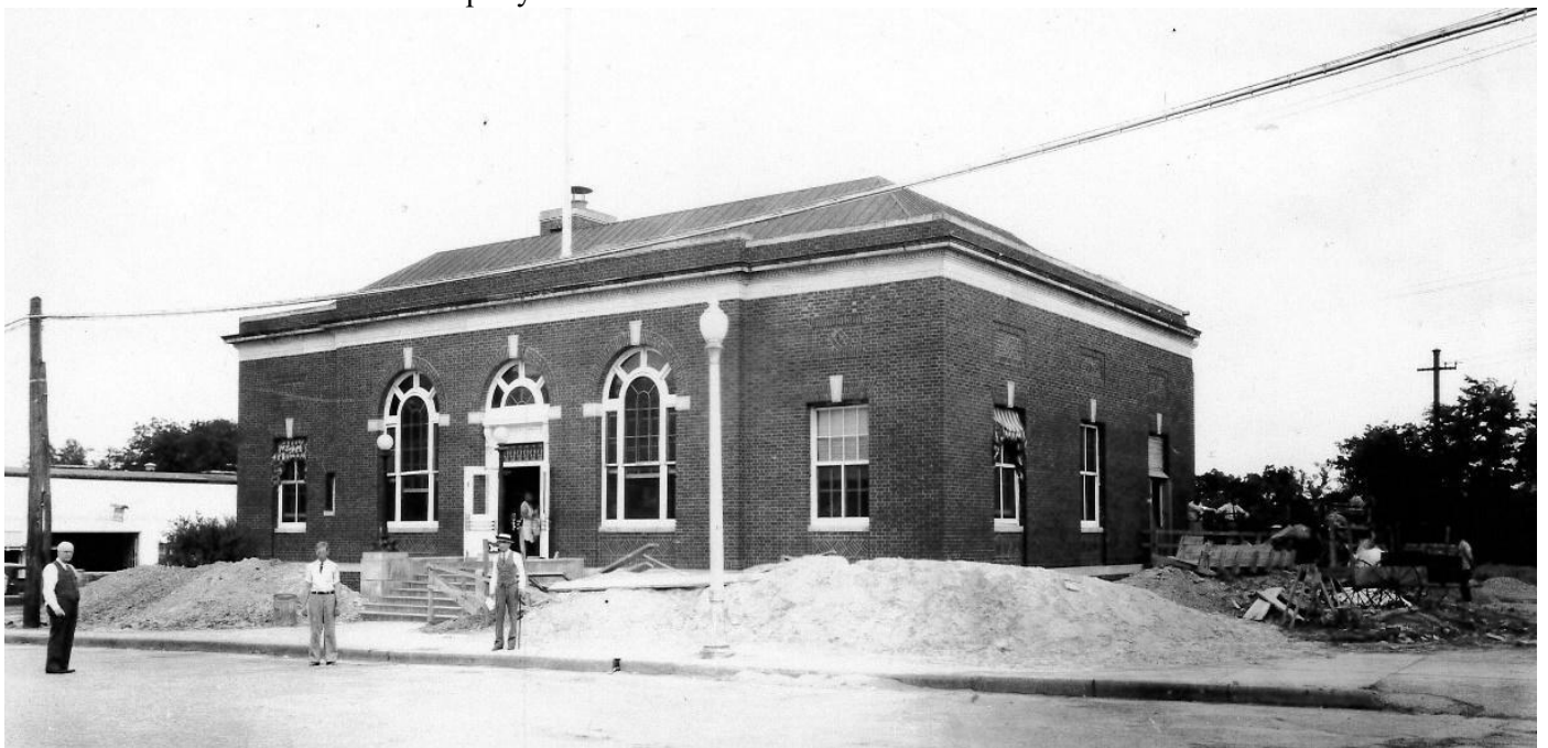
Figure 2: Bryan Federal Building and Post Office and Post Office, April 1939 front (south) elevation Beginning construction in addition. Source: Property Owner.
