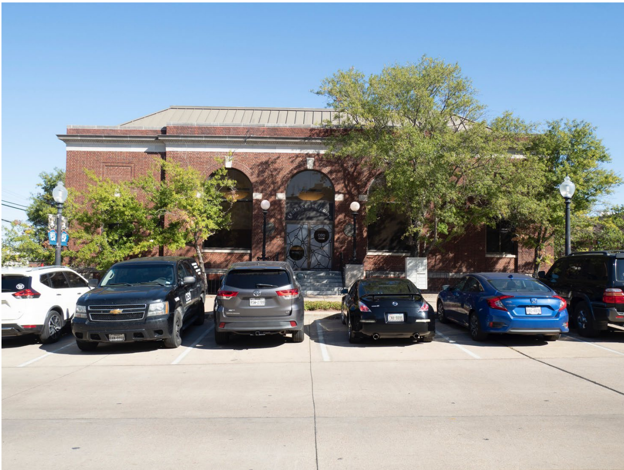
Photo 1: Primary (South) Elevation, View North.
