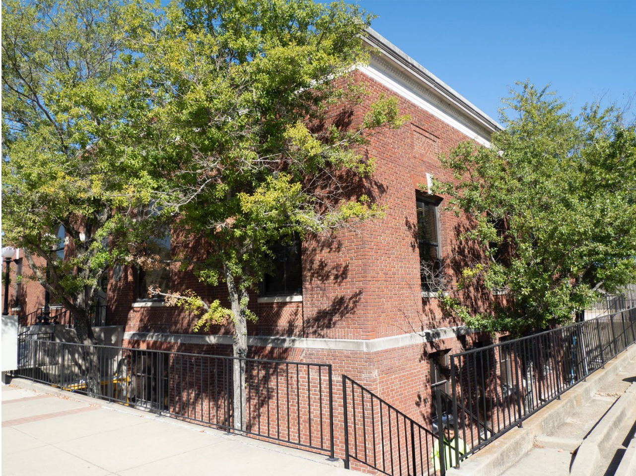
Photo 8: Oblique Showing Primary (South) and East Elevations, View Northwest.
