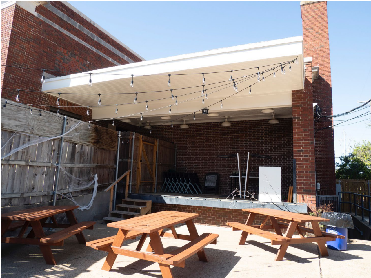
Photo 6: Northeast Corner Showing Mailing Platform, View Southwest.
