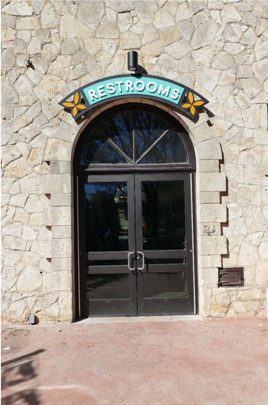
Photo 9: entrance on south elevation. View north.
