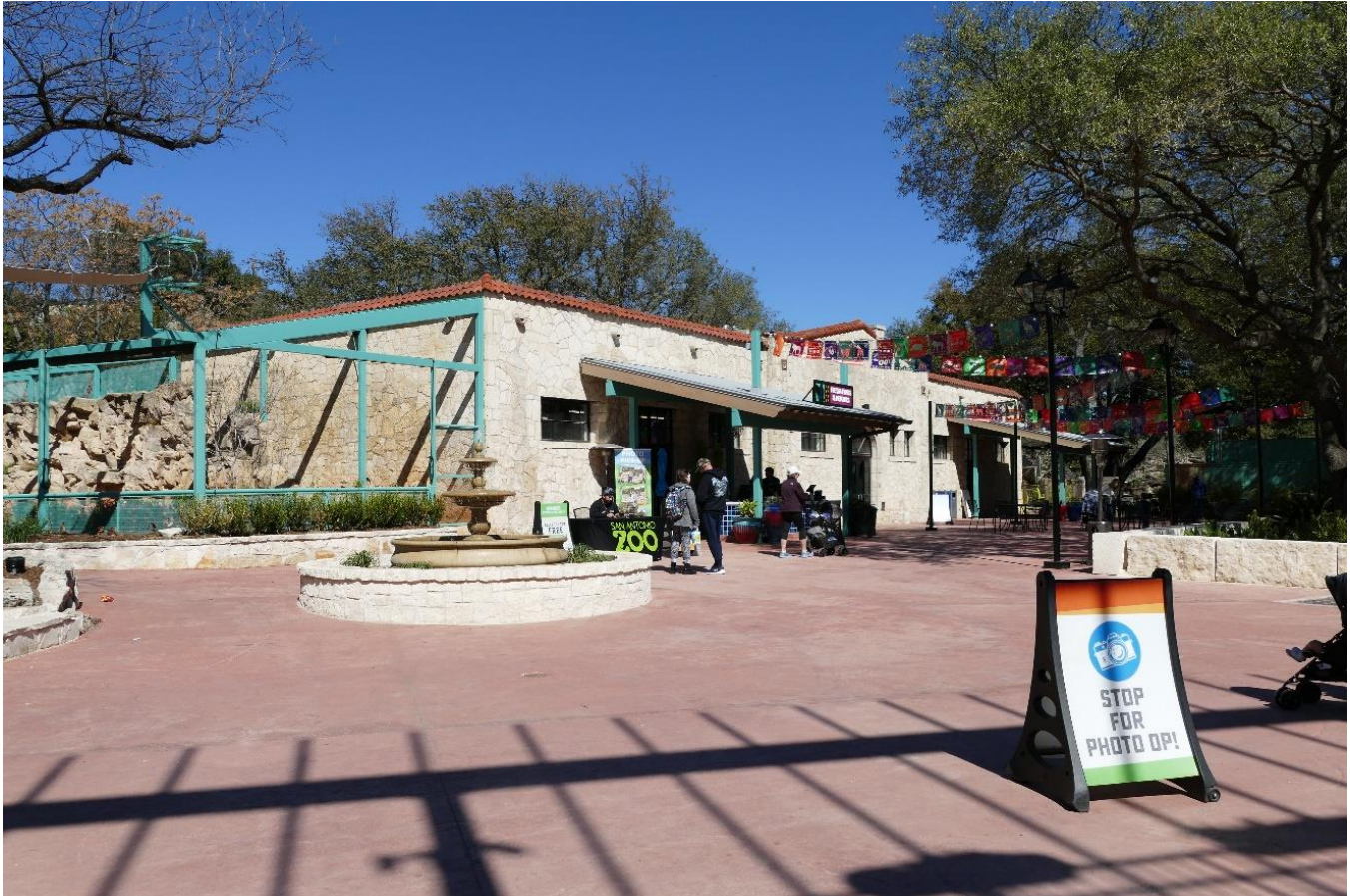
Photo 21: View of south and east elevations from zoo entrance. View northwest.
