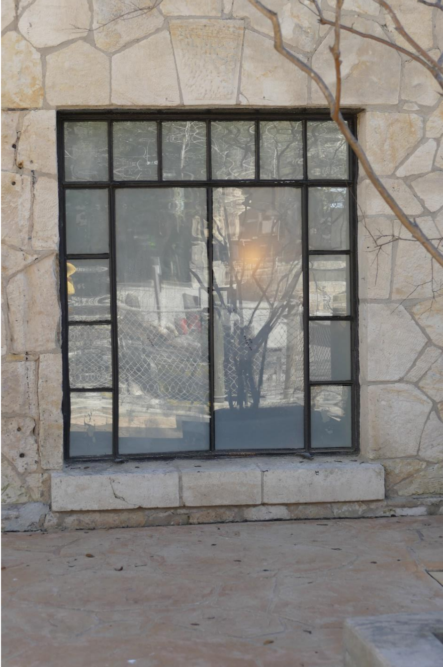
Photo 3: Restored window on north elevation. View south.
