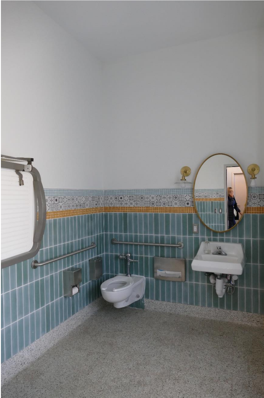
Photo 13: former office, now family restroom. View east.
