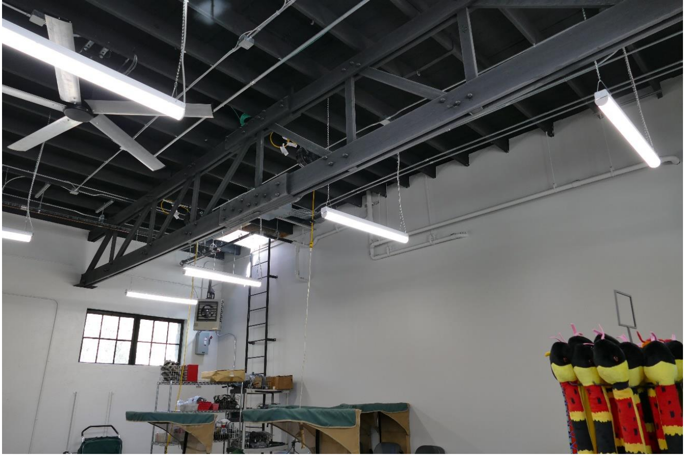
Photo 16: roof truss. View southwest.
