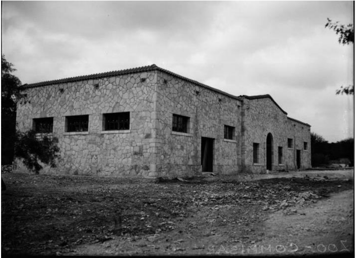
Figure 1. Monkey House/Commissary under construction, c. 1936. University of Texas at San Antonio Special Collections.
