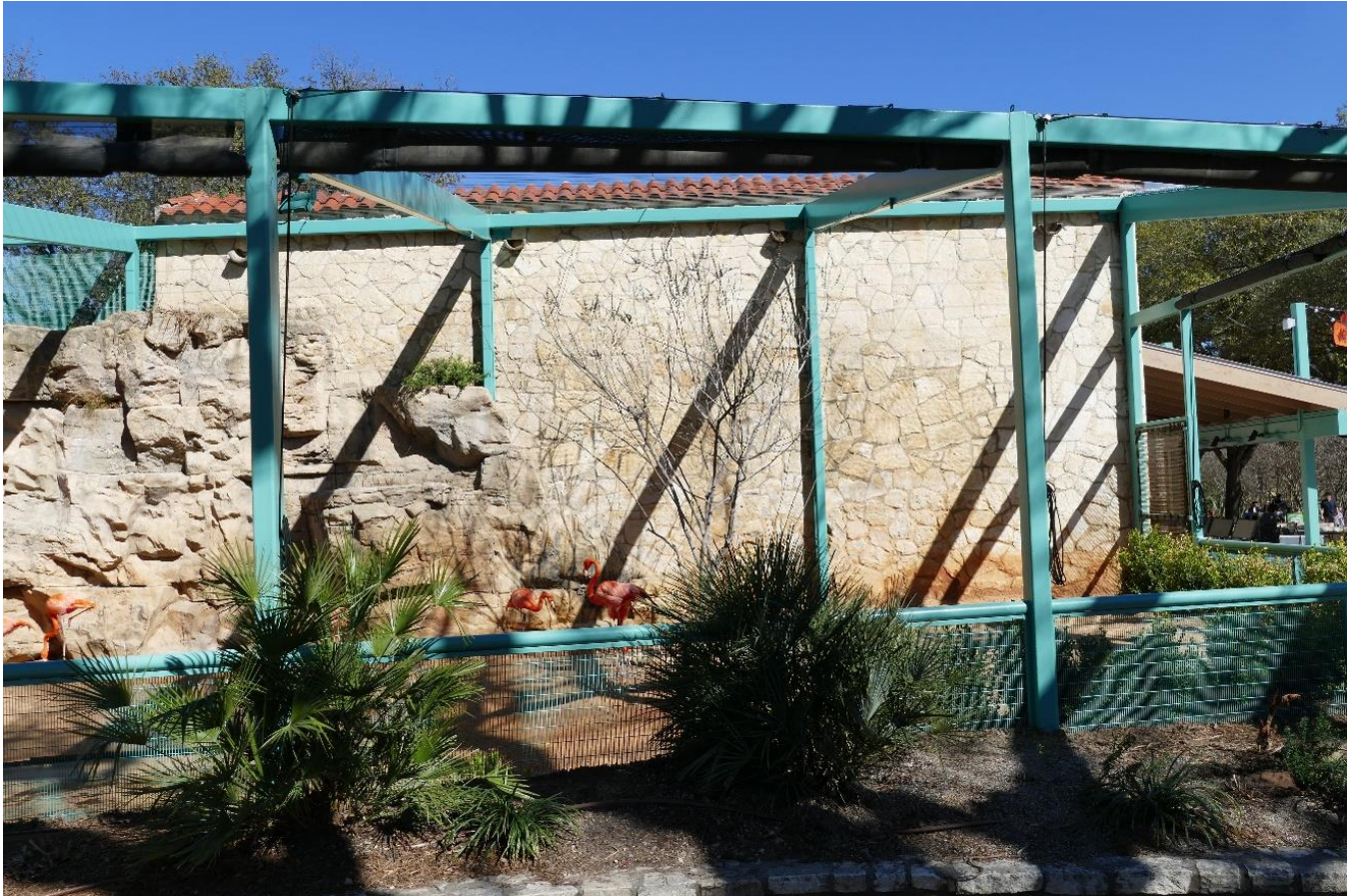
Photo 11: west elevation. View east.
