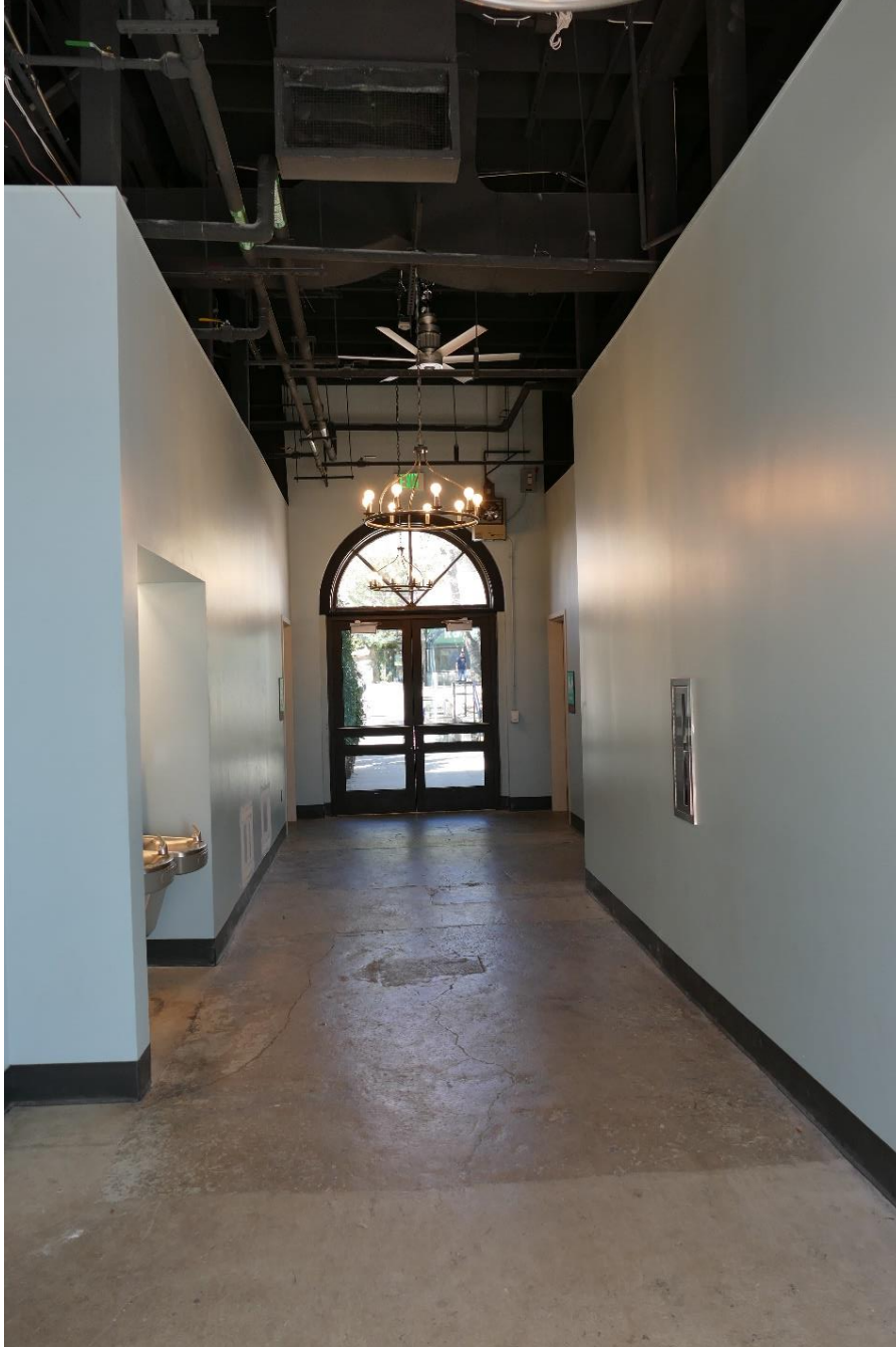
Photo 12: interior north elevation entrance and corridor. View north.
