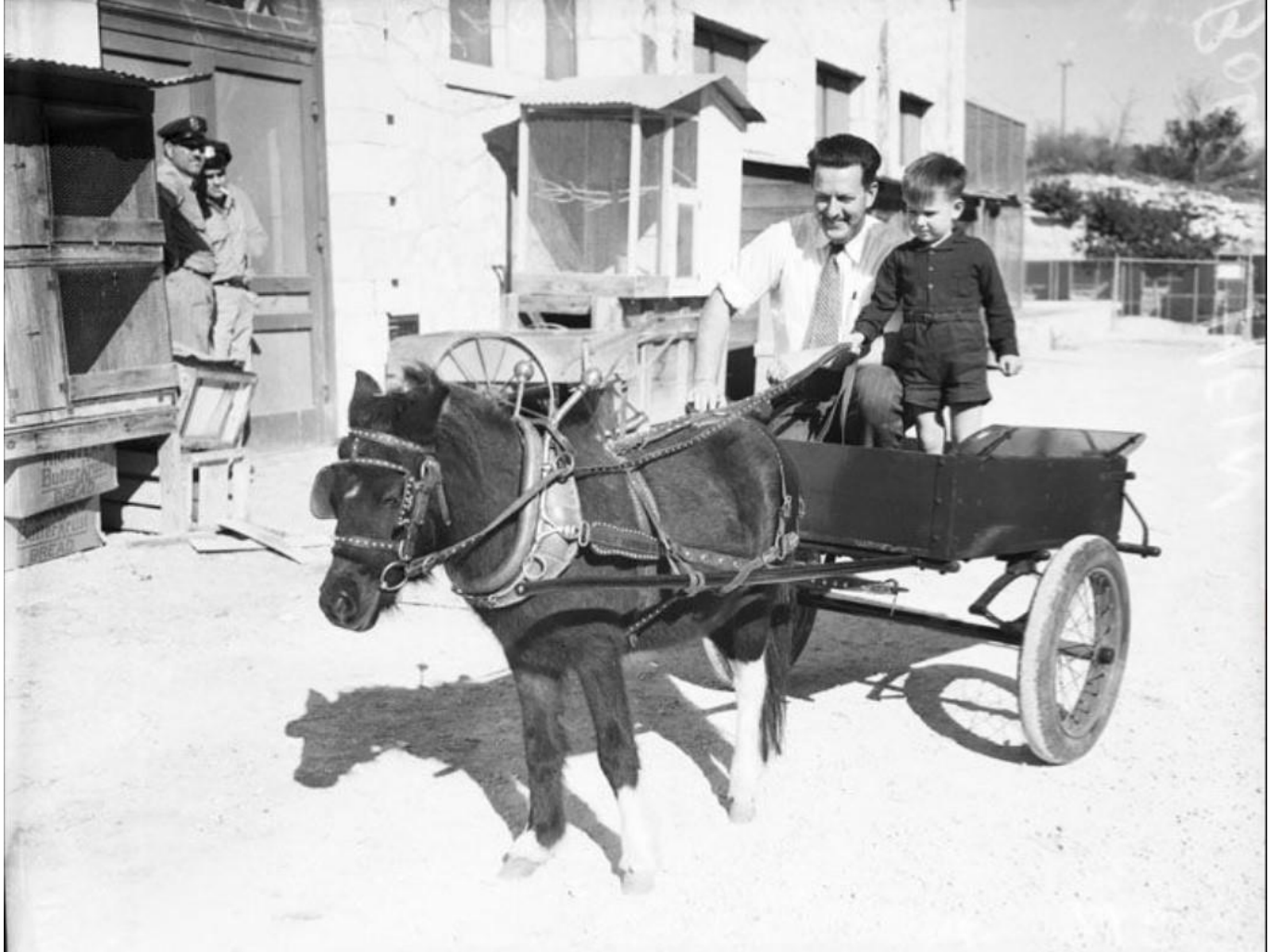
Figure 2. Monkey House/Commissary, c. 1939. University of Texas at San Antonio Special Collections. Note original metal animal enclosures at far right of photograph.
