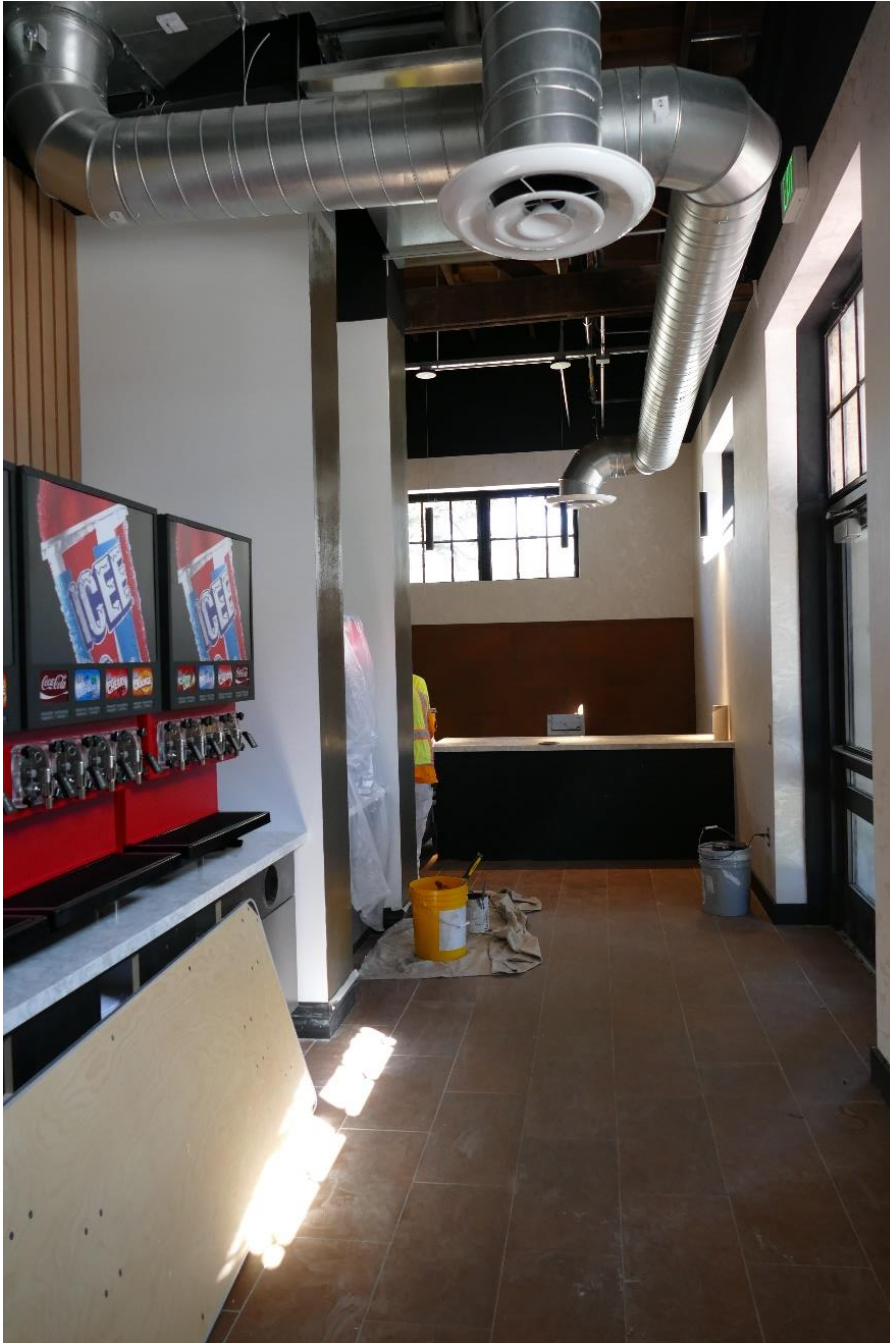
Photo 17: former east end, now restaurant food preparation area. View east.
