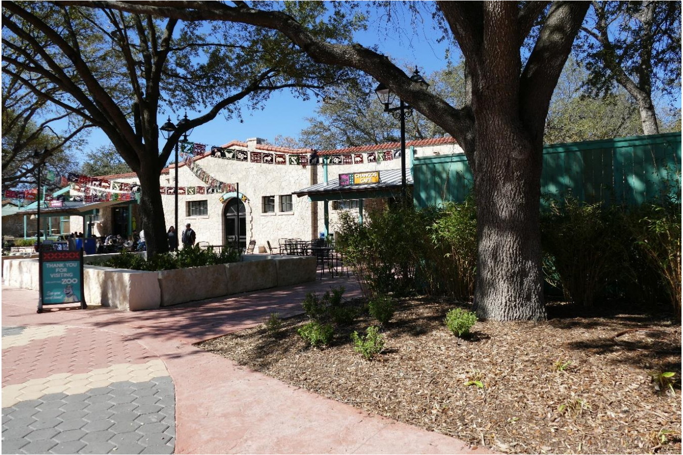
Photo 10: plaza located south of the building. View southwest.
