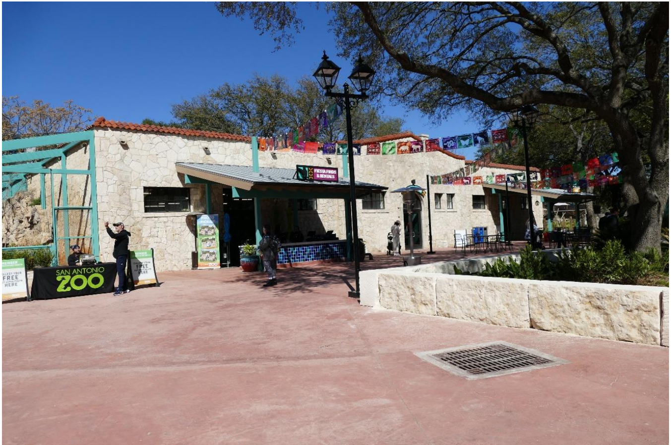
Photo 8: South elevation. View northeast.
