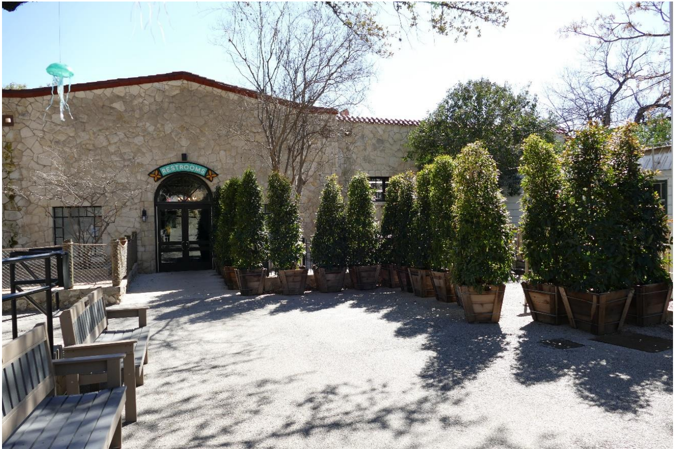
Photo 2: primary entrance on north elevation. View south.
