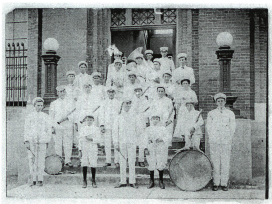
Early photograph of Courthouse Annex entrance
