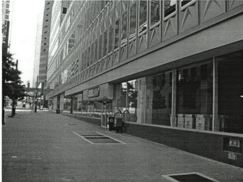
Ground floor, along Bryan Street (facing southeast)
