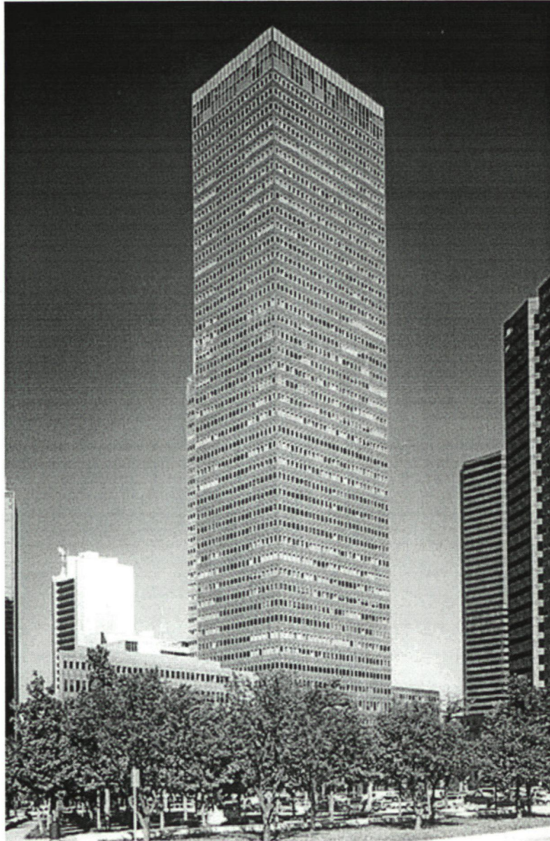
Tower II (facing west)
