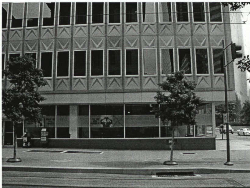
Ground floor at Bryan & Ervay (facing southeast)
