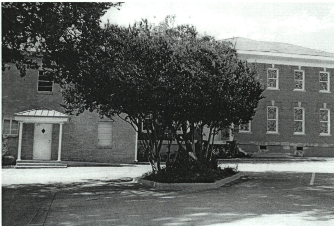
North elevation, showing addition on left, original structure on right
