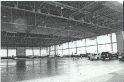
Interior of Hangar, Looking Southeast
