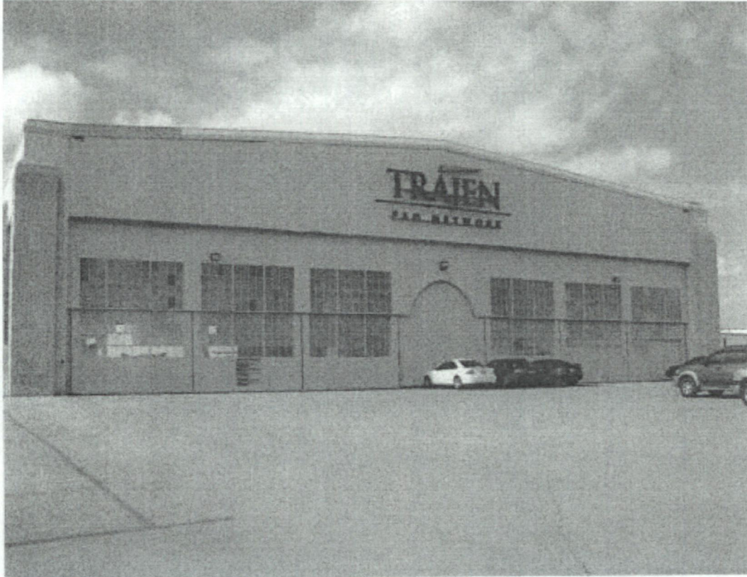
East Elevation, Camera Facing West
