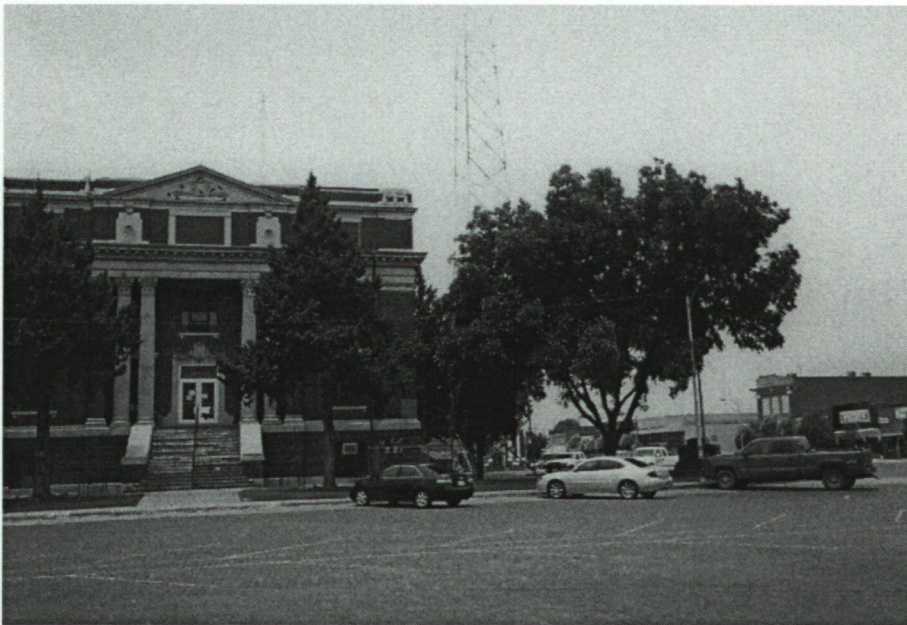
East elevation; radio tower to right of courthouse
