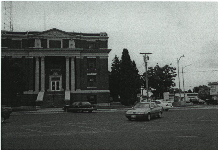
West elevation; another non-contributing monument on right at edge of courthouse lawn
