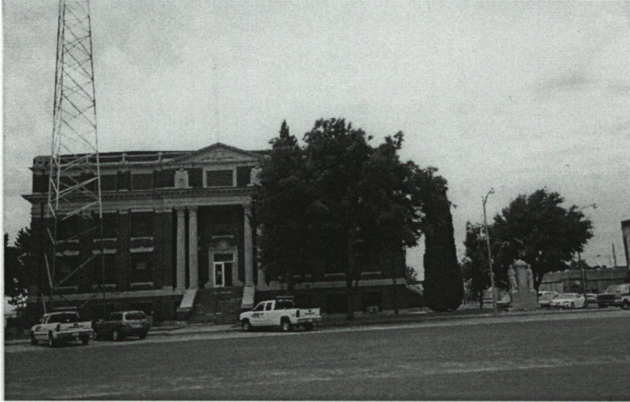
North elevation with radio tower on right and a non-contributing monument on right at edge of courthouse lawn
