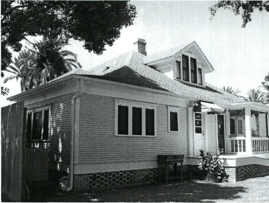
Rear (north) and east elevations
