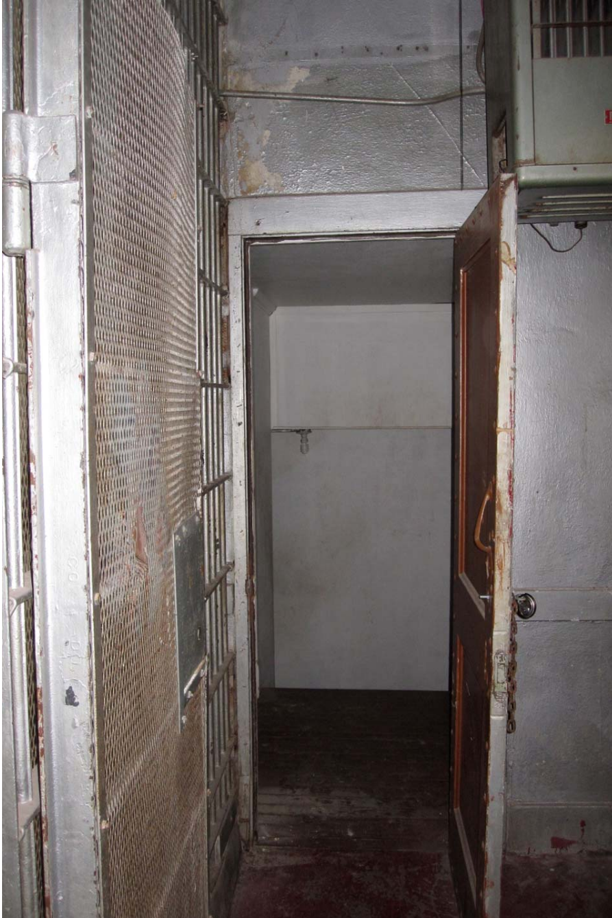
Photo 11: Third floor corridor
