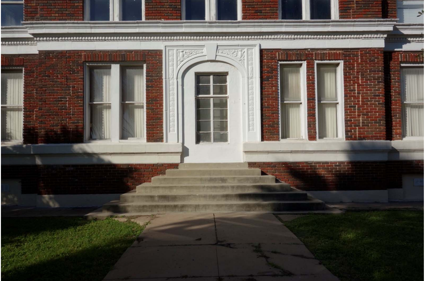
Photo 4: East Elevation, entry detail
