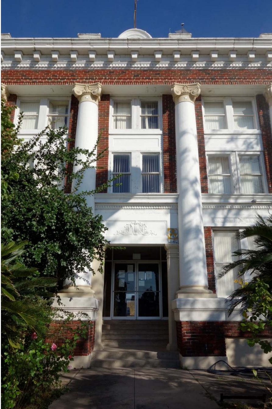
Photo 2: South Elevation, entry detail
