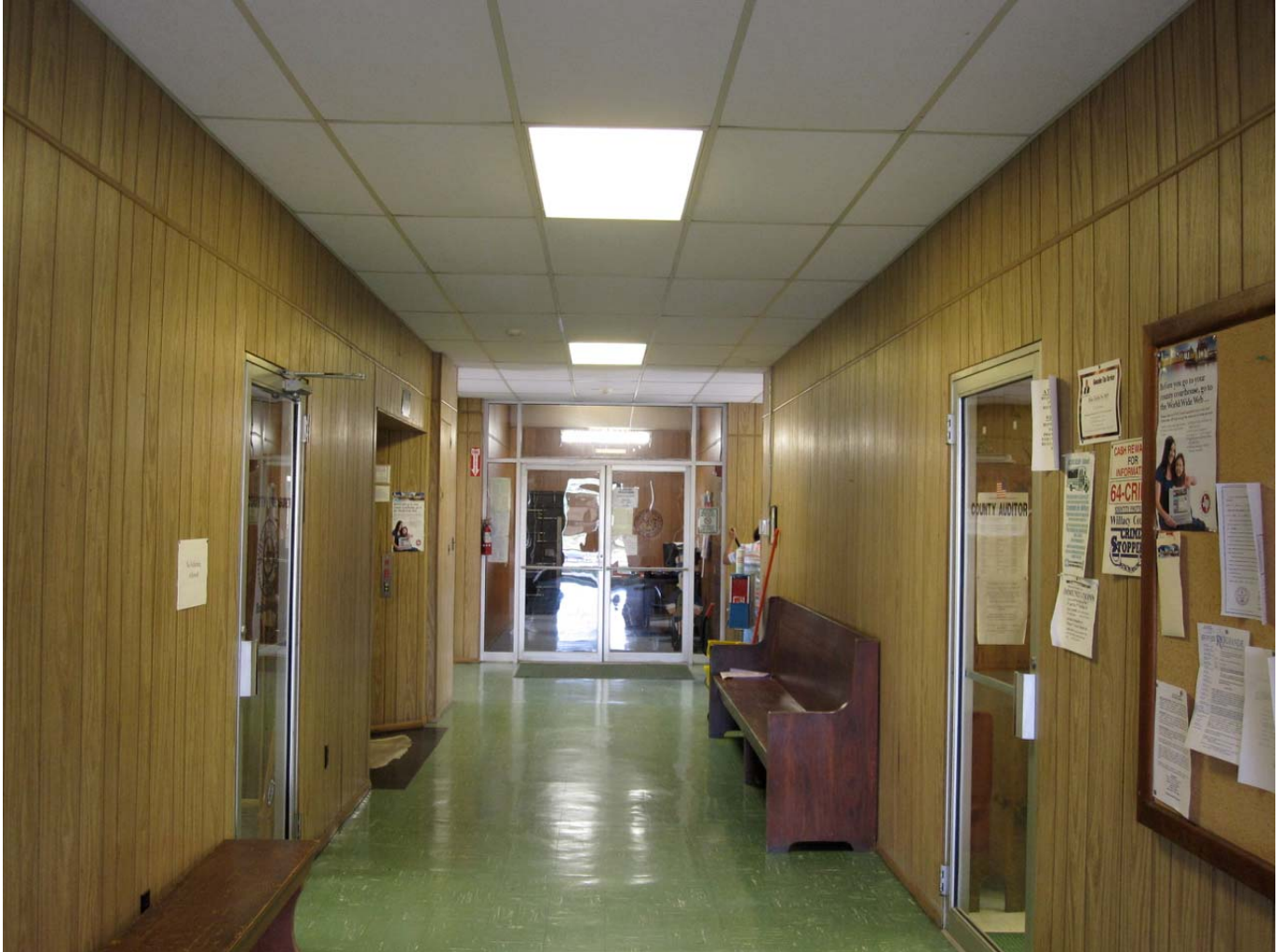
Photo 9: First floor corridor
