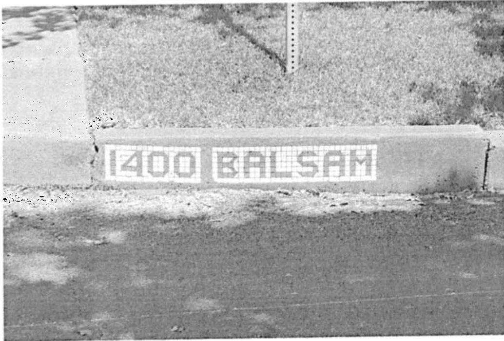
Photo #13 Example of ceramic curb tiles
