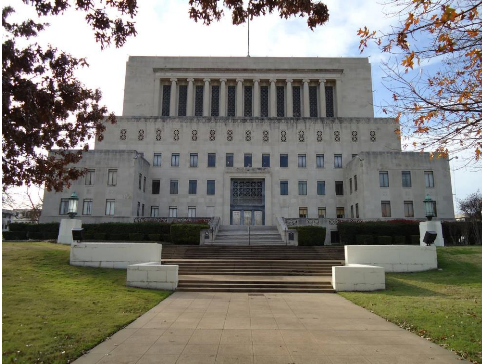
Photo 1: Façade (east) elevation and two lanterns, January 8, 2016, looking west.
