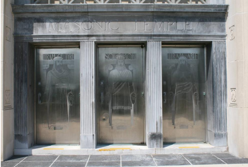
Photo 3: East entrance, August 30, 2016, looking west.
