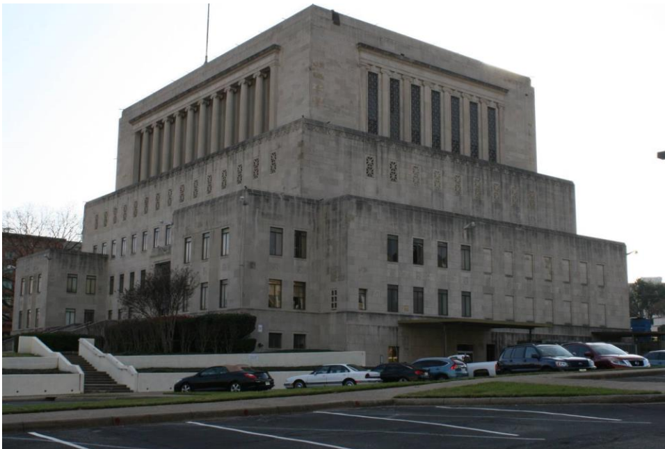
Photo 2: Façade and north elevation, January 8, 2016, looking southwest.
