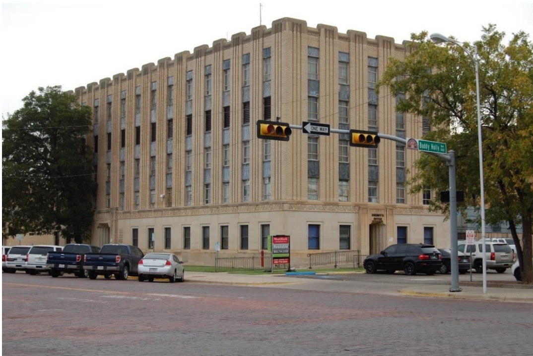
Photo 2: North and West Elevations
