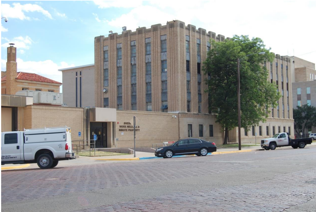
Photo 5: North and East Elevations
