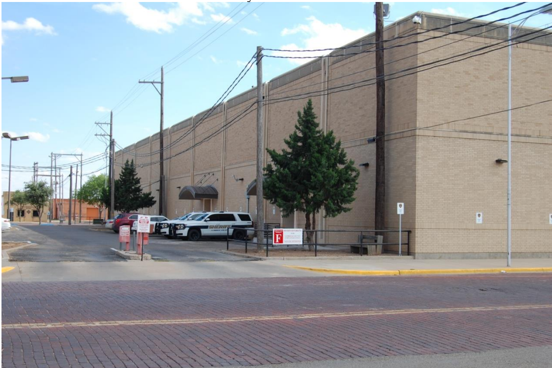
Photo 8: East Elevation of Lubbock County Detention Center
