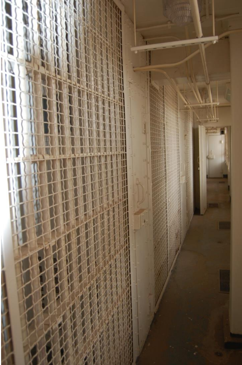
Photo 20: Inspection Corridor about Fifth Floor Cell Block
