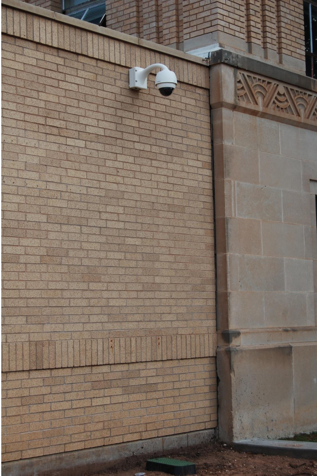
Photo 12: North Elevation where the Lubbock County Detention Facility meets the Lubbock County Jail
