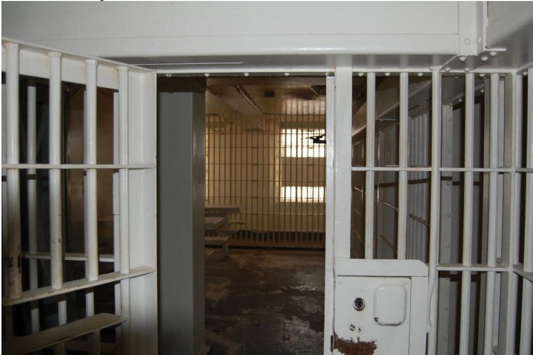
Photo 19: Security Entrance into Fifth Floor Cell Block
