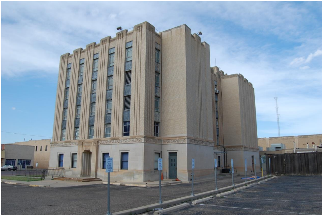
Photo 4: South and West Elevations
