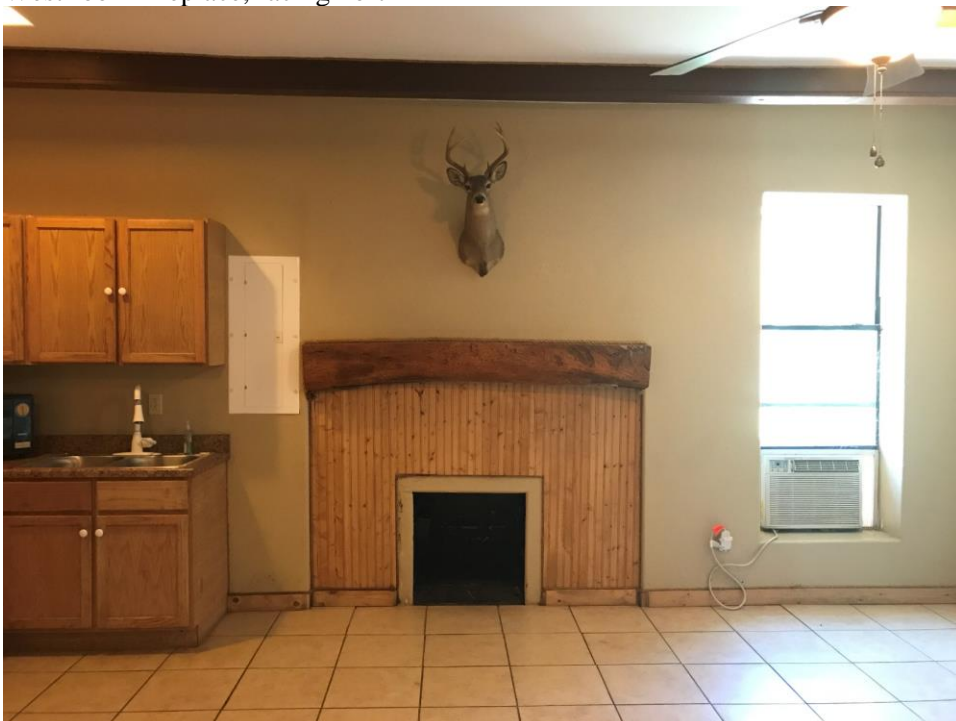
Photo 16 West room fireplace, facing north
