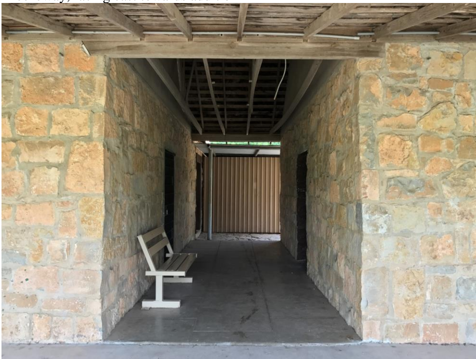
Photo 10 Breezeway, facing east towards addition
