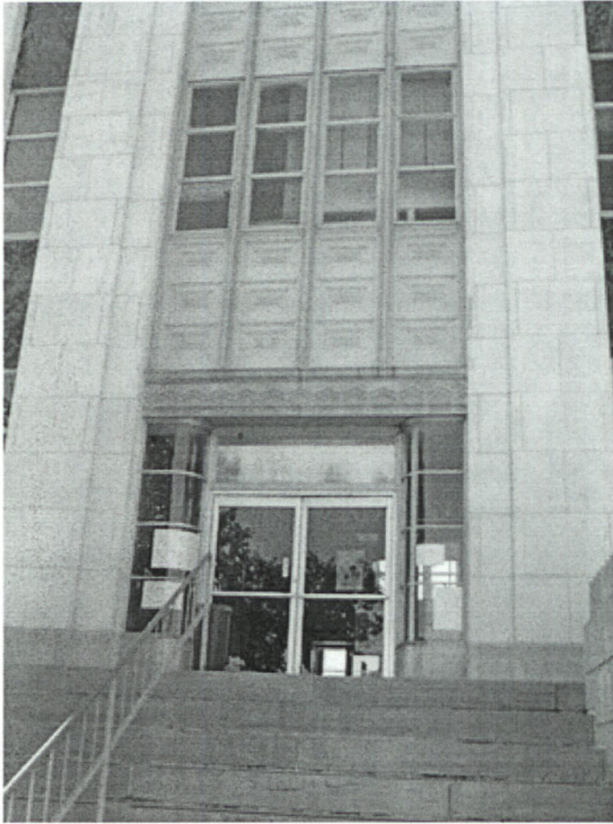
Photo 2. Current exterior details. A major entrance, left, features curved glass sidelights and metal spandrel panels of an incised grid of squares. The grand staircase features fluted balusters and urns for plantings.
