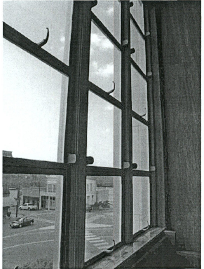
Photo 4. Current details. Steel windows and exterior marble spandrels.
