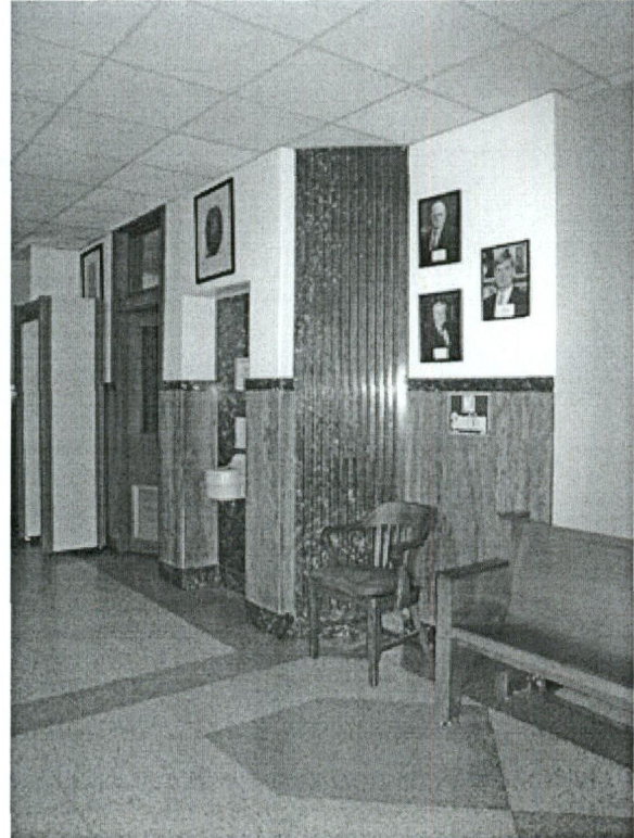
Photo 7. Current interior details. Moderne zig-zag aluminum screens at hallways transoms and sidelights, terrazzo floors, and marble wall coverings, including fluted pilasters and wainscoting on second floor.
