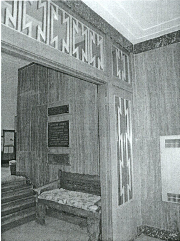
Photo 7. Current interior details. Moderne zig-zag aluminum screens at hallways transoms and sidelights, terrazzo floors, and marble wall coverings, including fluted pilasters and wainscoting on second floor.
