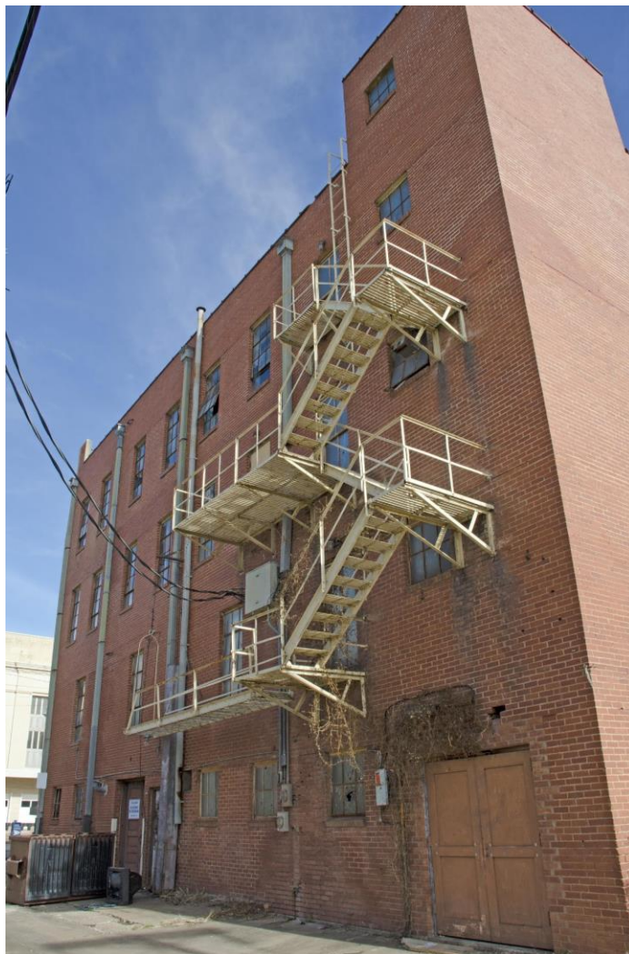
Photo 5 - Southwest (Rear) Elevation, view north.
