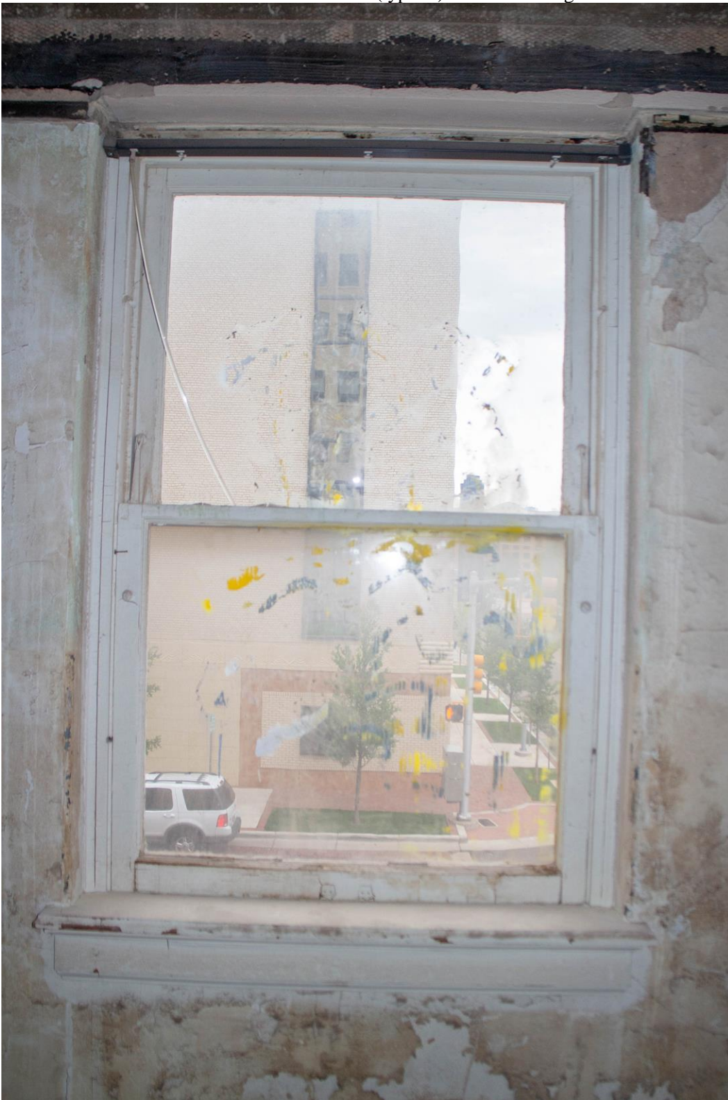
Photo 21: Second floor wood astral window (typical). Camera facing north.
