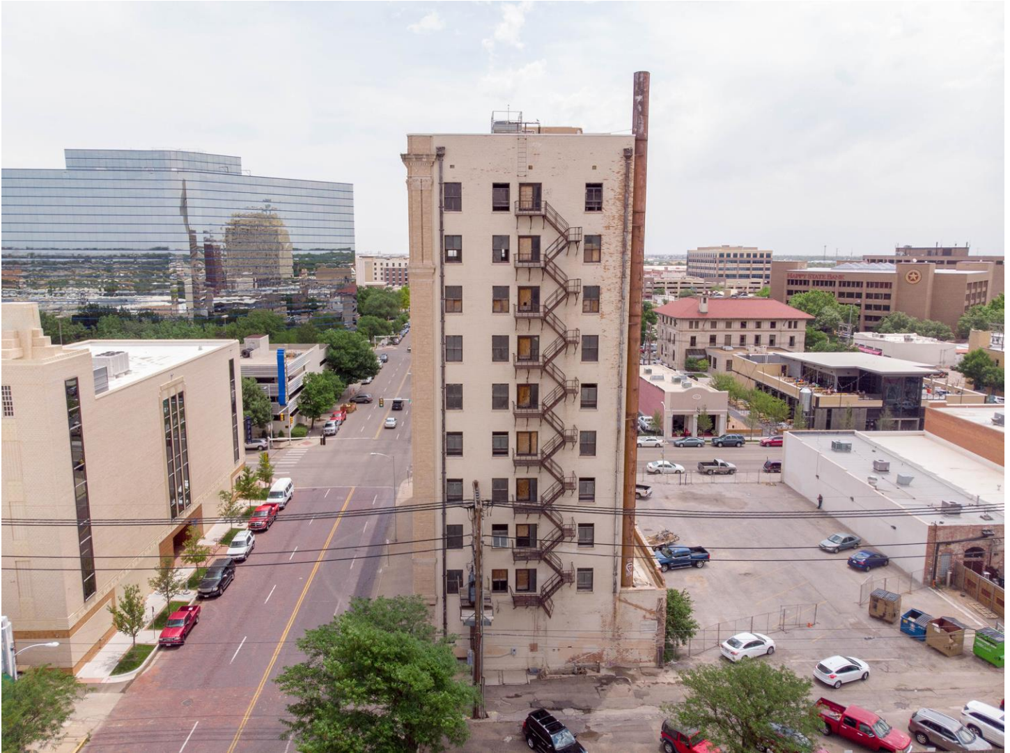
Photo 9: West (rear) elevation. Camera facing east.
