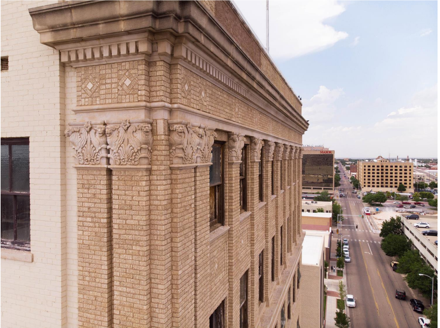
Photo 11: Detail of cornice and parapet. Camera facing northwest.
