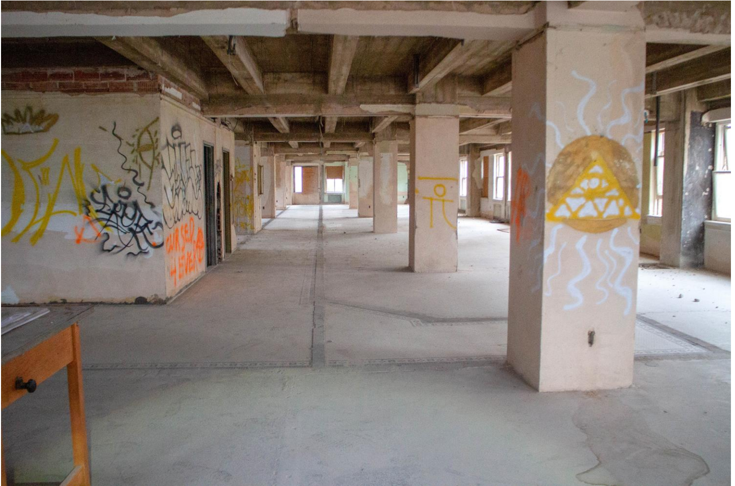
Photo 19: Second floor general view. Camera facing west.
