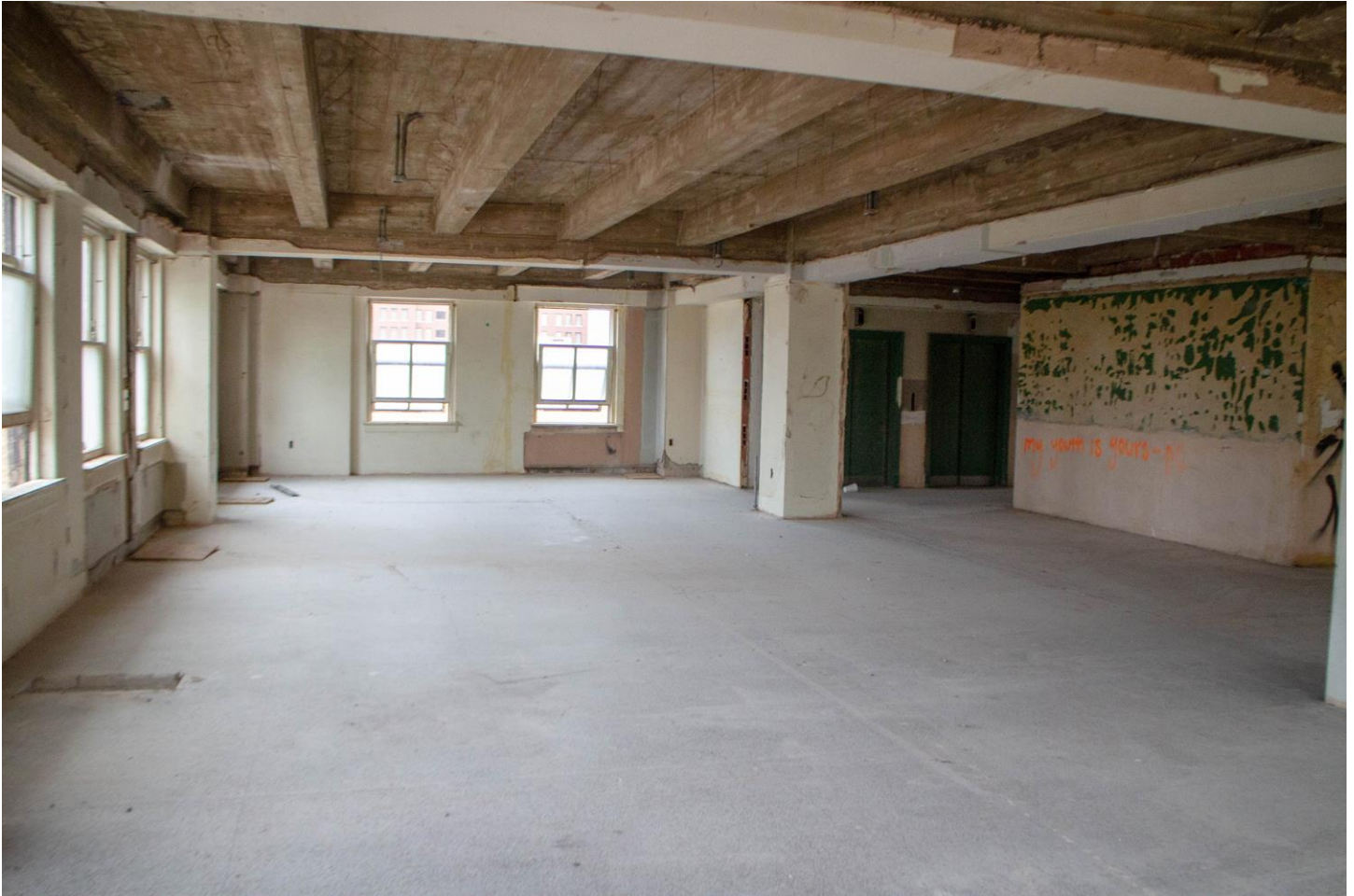
Photo 24: Third floor general view (typical). Camera facing south.
