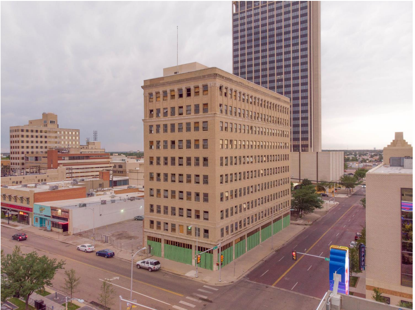
Photo 5: Northeast (primary) oblique. Camera facing southwest.
