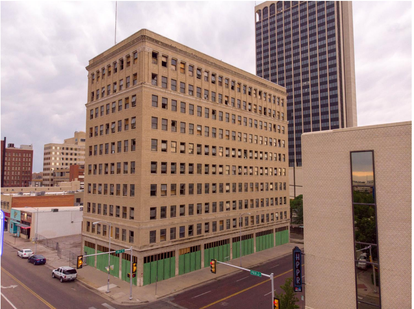
Photo 8: Northeast (primary) oblique. Camera facing southwest.
