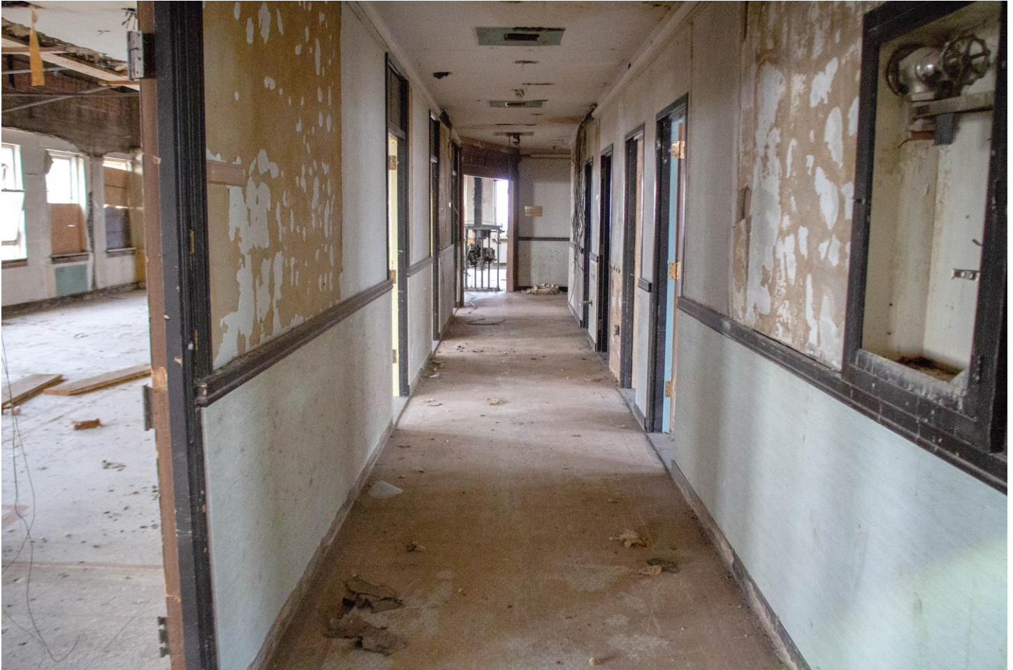
Photo 27: Tenth floor corridor. Camera facing east.
