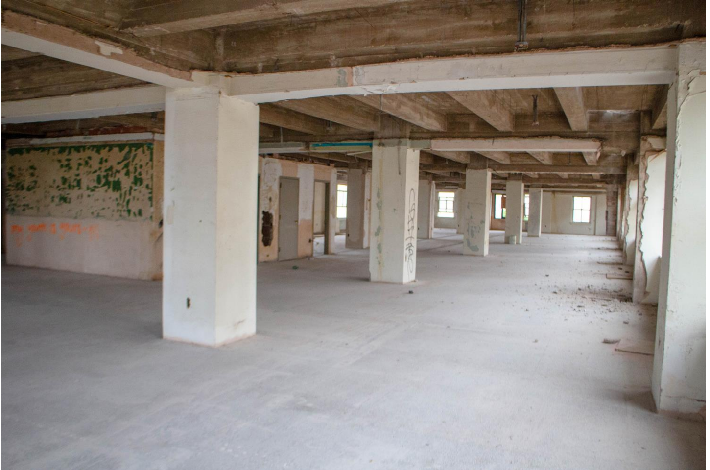
Photo 23: Third floor general view (typical). Camera facing west.
