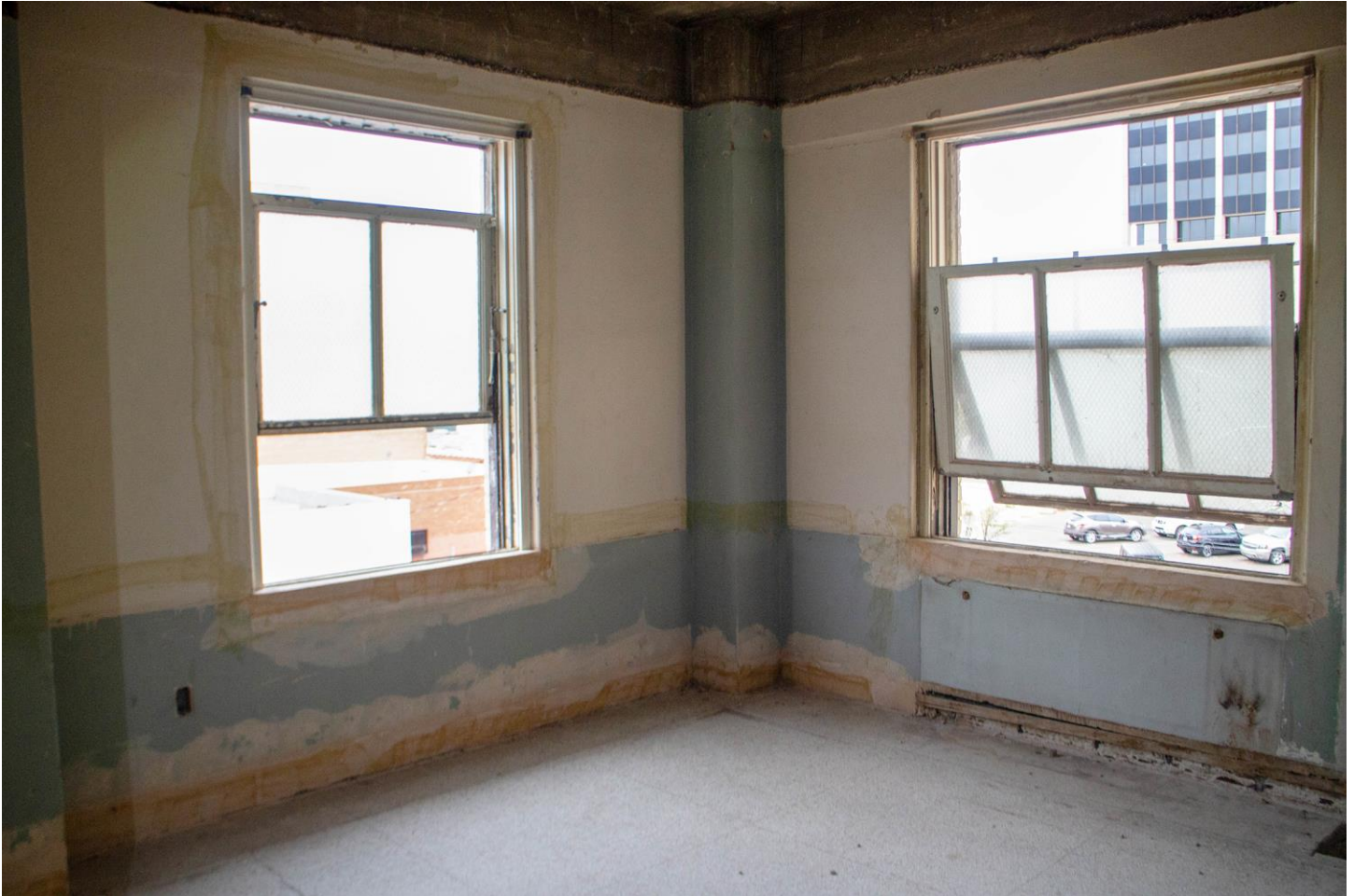
Photo 22: Second floor steel austral windows (typical). Camera facing southwest.
