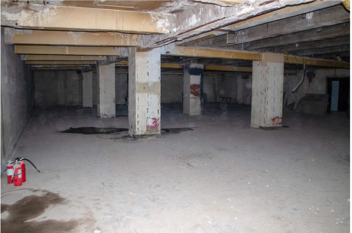
Photo 13: General view in basement (typical). Camera facing east.
