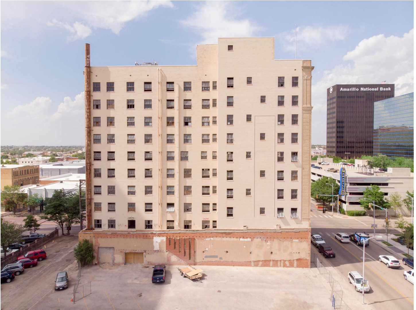
Photo 10: South elevation. Camera facing north.
