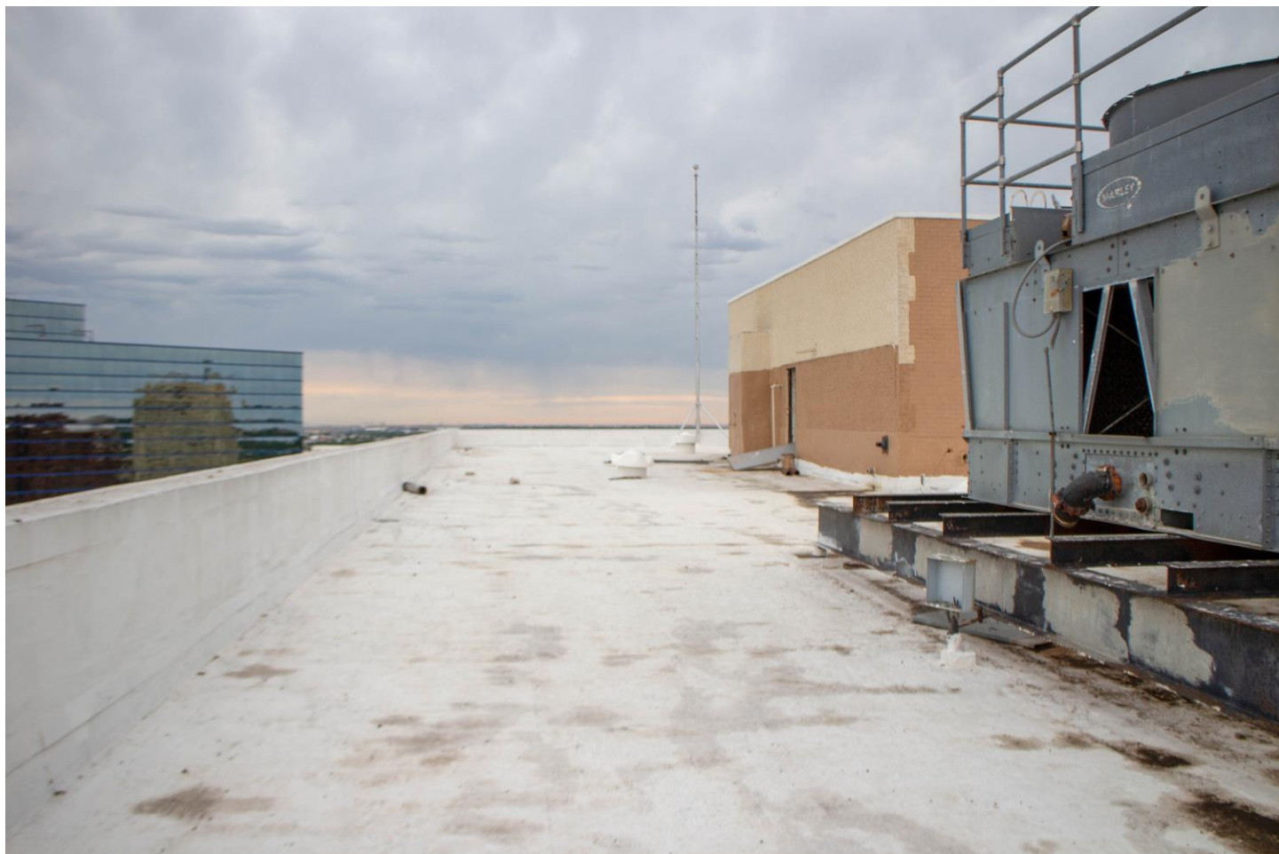
Photo 29: General view of roof. Camera facing west.
