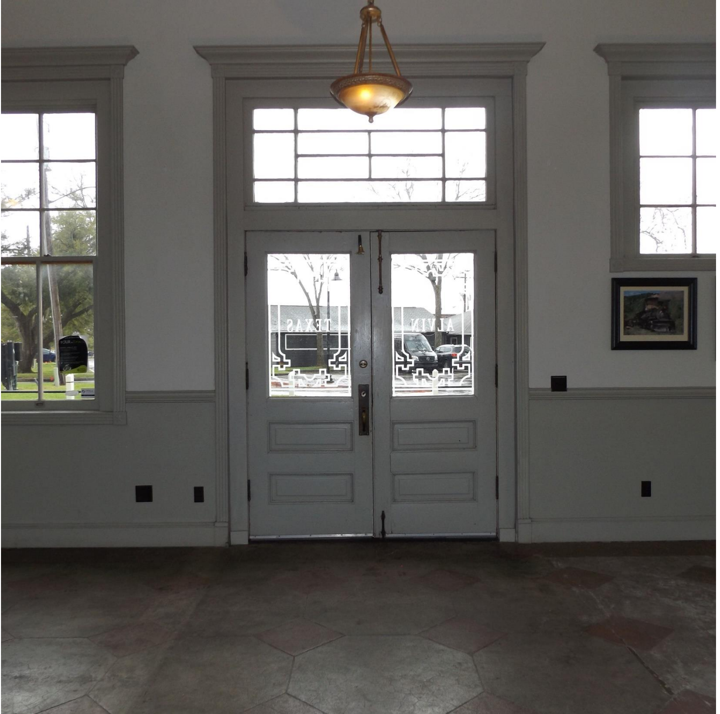
Photo 9 Detail of south entrance to Main Waiting Room, facing south.
