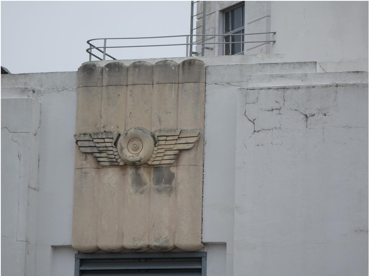
Photo 7 Winged wheel motif, south elevation Photo by Gregory Smith, December 2016
