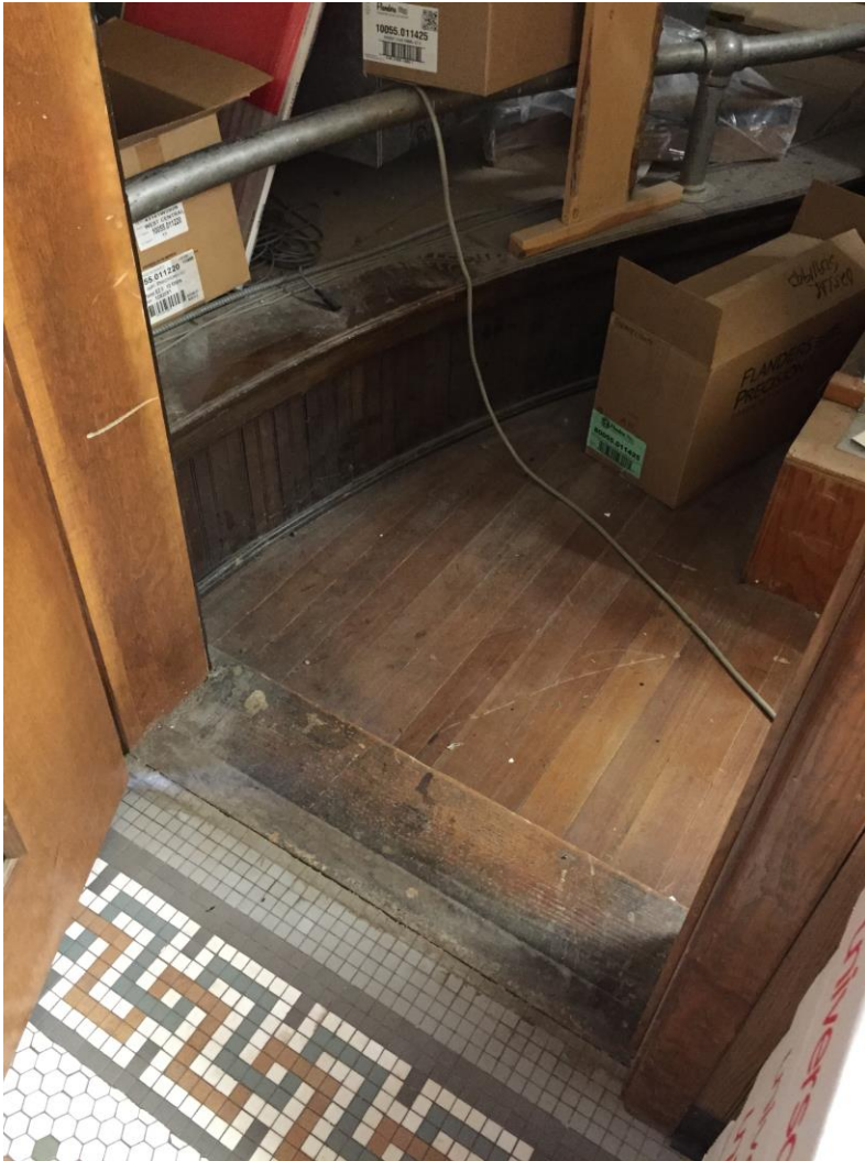
Photo 21 Third floor mezzanine level.
