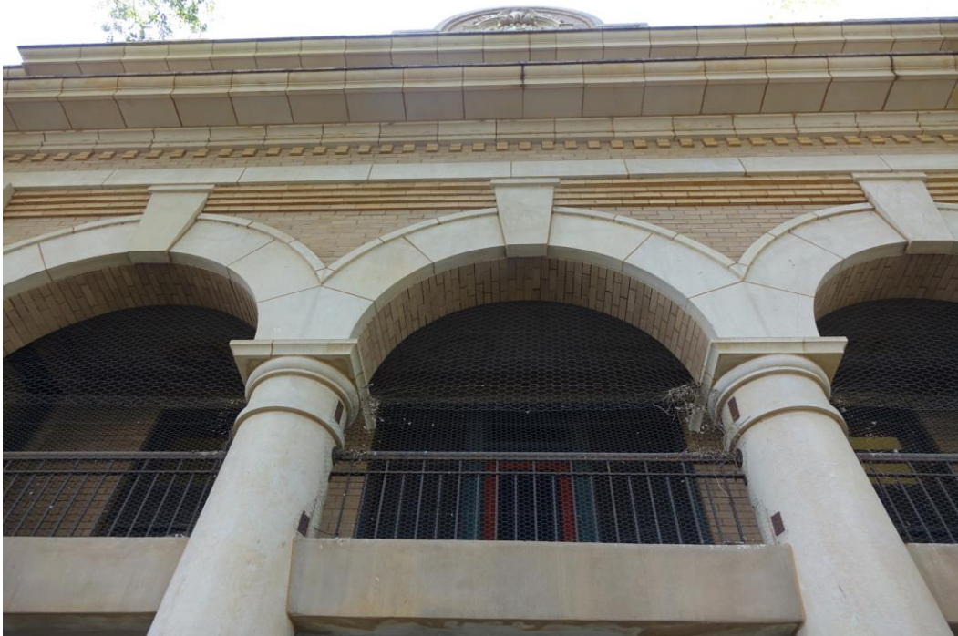
Photo 6 Second floor balcony, west side.
