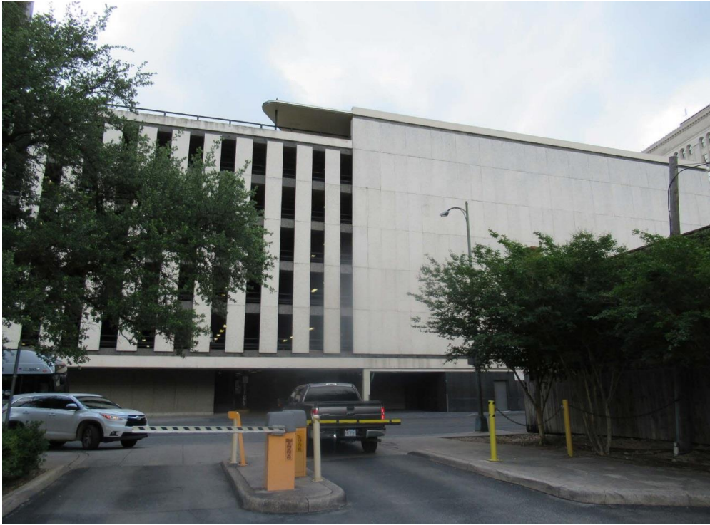
Photo #17: Frost Bank Parking Garage, 109 N. Main, 117 W. Commerce Street, West façade, camera facing east
