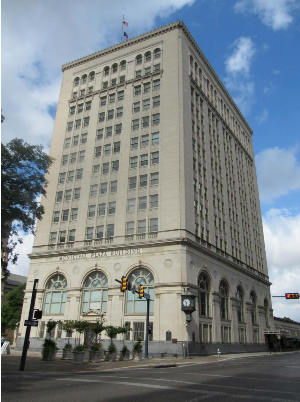
Photo #4: Municipal Building, 103 or 114 S. Main, Northeast oblique, camera facing southwest
