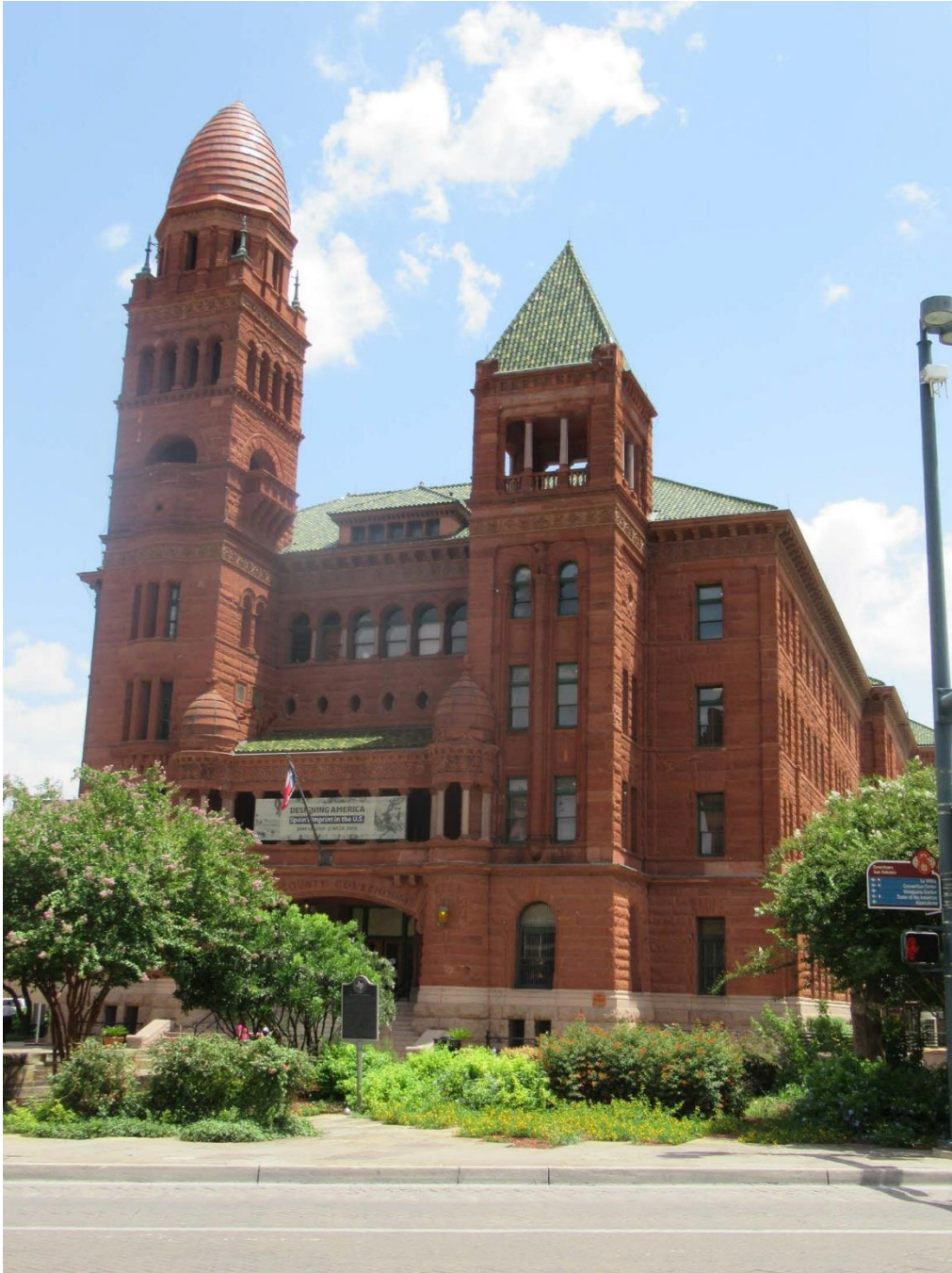
Photo #3: Bexar County Courthouse, 100 Main Plaza, North façade, camera facing south
