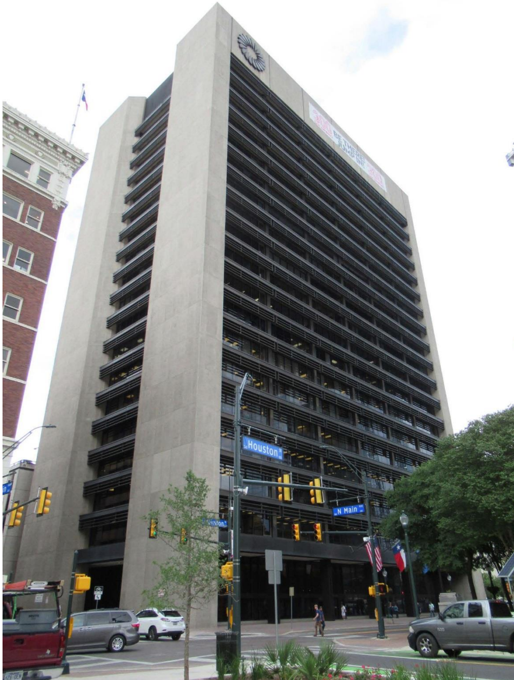
Photo #16: Frost Tower, 100 Houston Street, North façade, camera facing southeast
