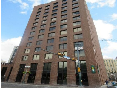
ID# 21 River View Tower 111/ 115 Commerce Street/ Soledad Street Non-Contributing
