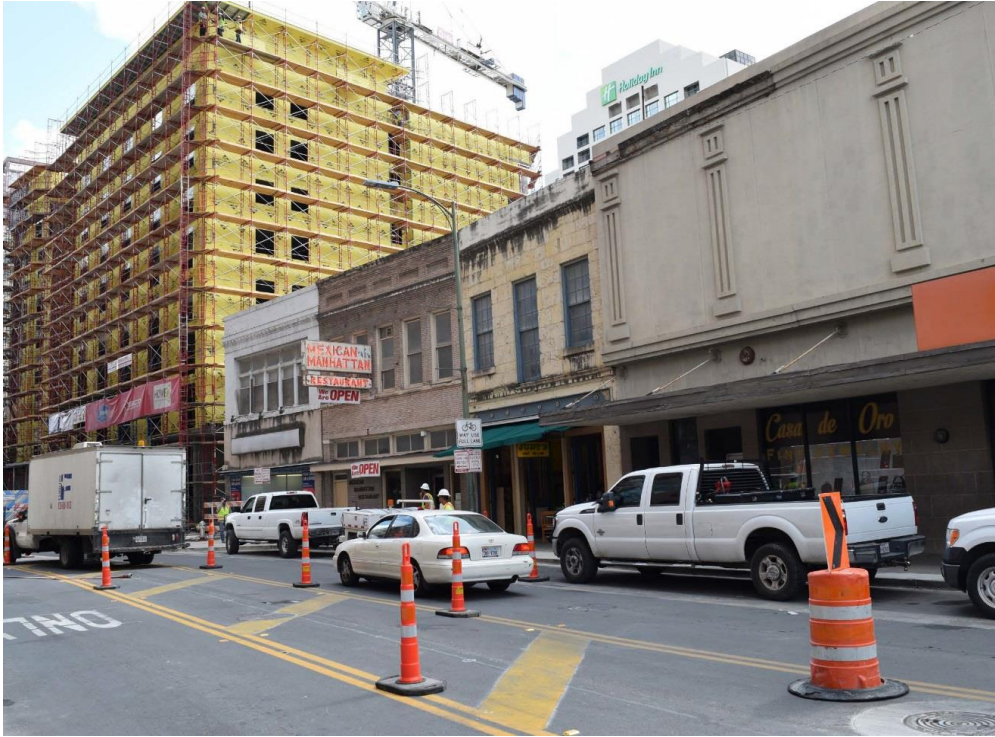
Photo #21: Soledad Block, 102-118 Soledad Street, southwest oblique, camera facing northeast
