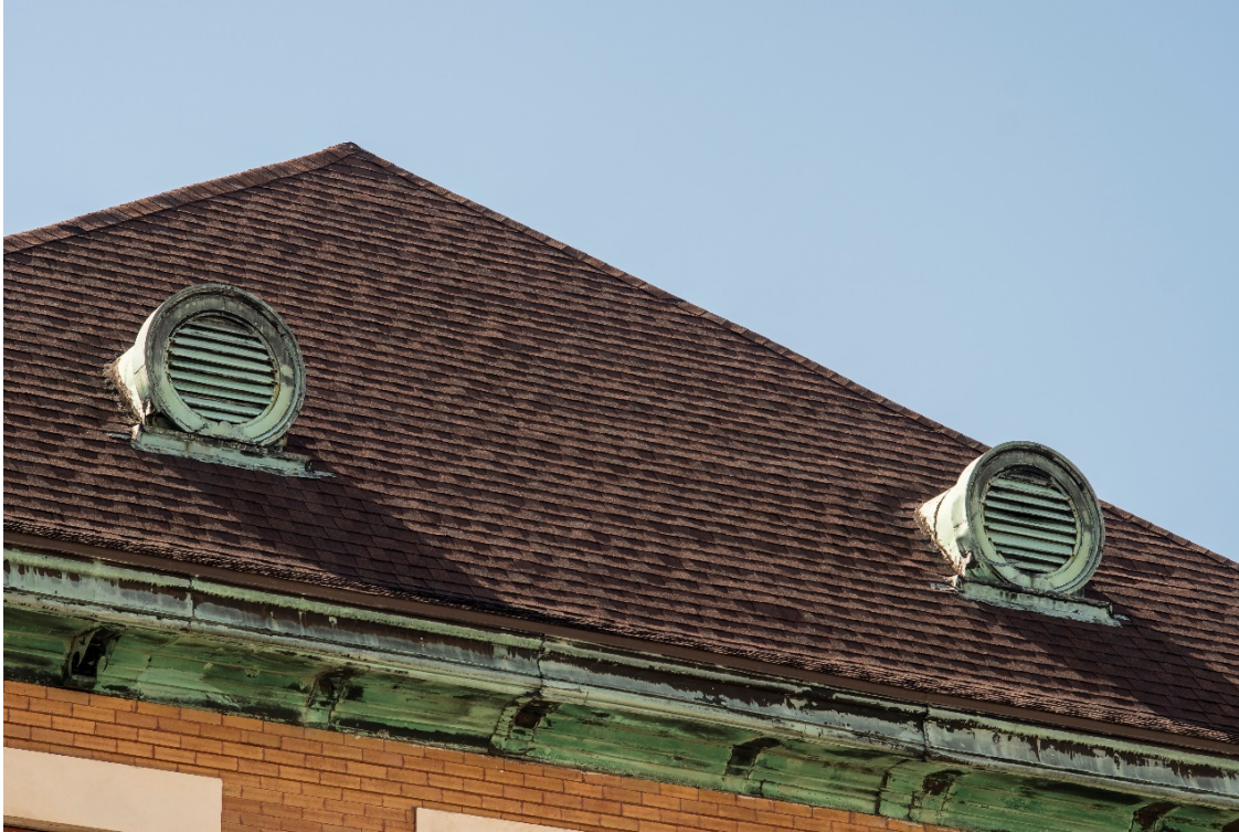
Photo 10: Roof detail. Looking south.
