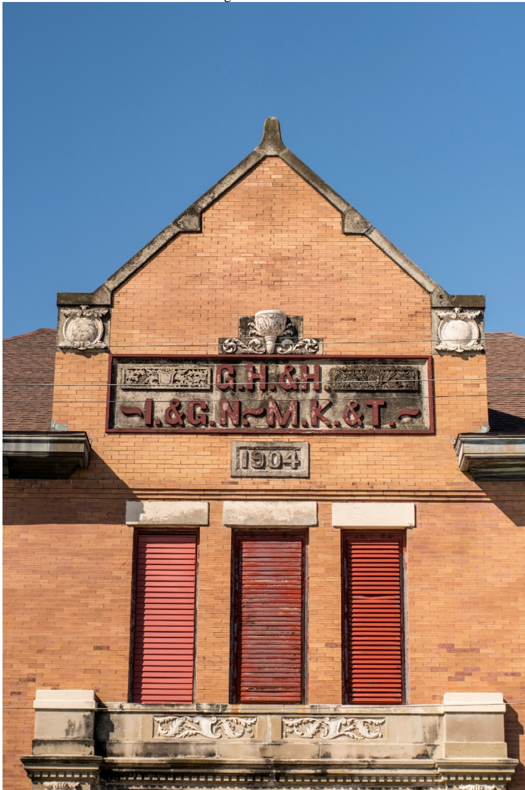
Photo 6: East elevation detail. Looking west.
