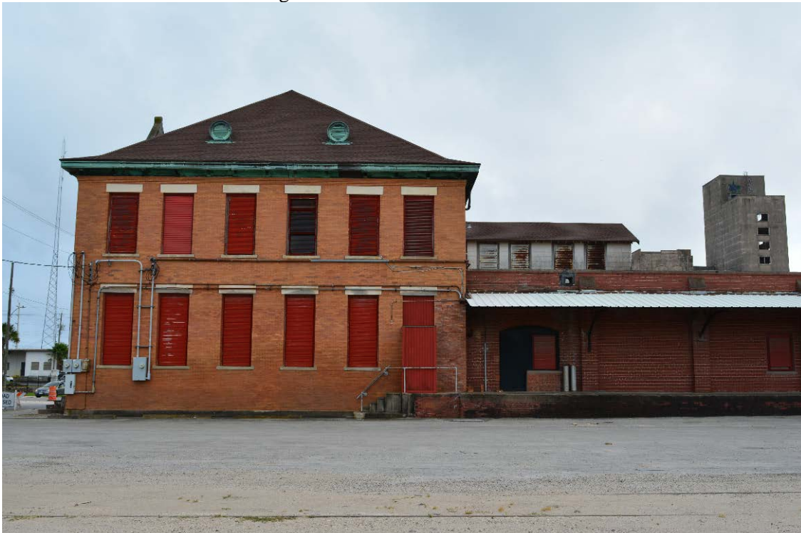
Photo 3: North elevation. Looking south.
