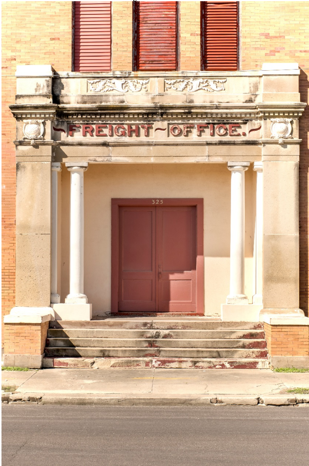
Photo 7: East elevation detail. Looking west.
