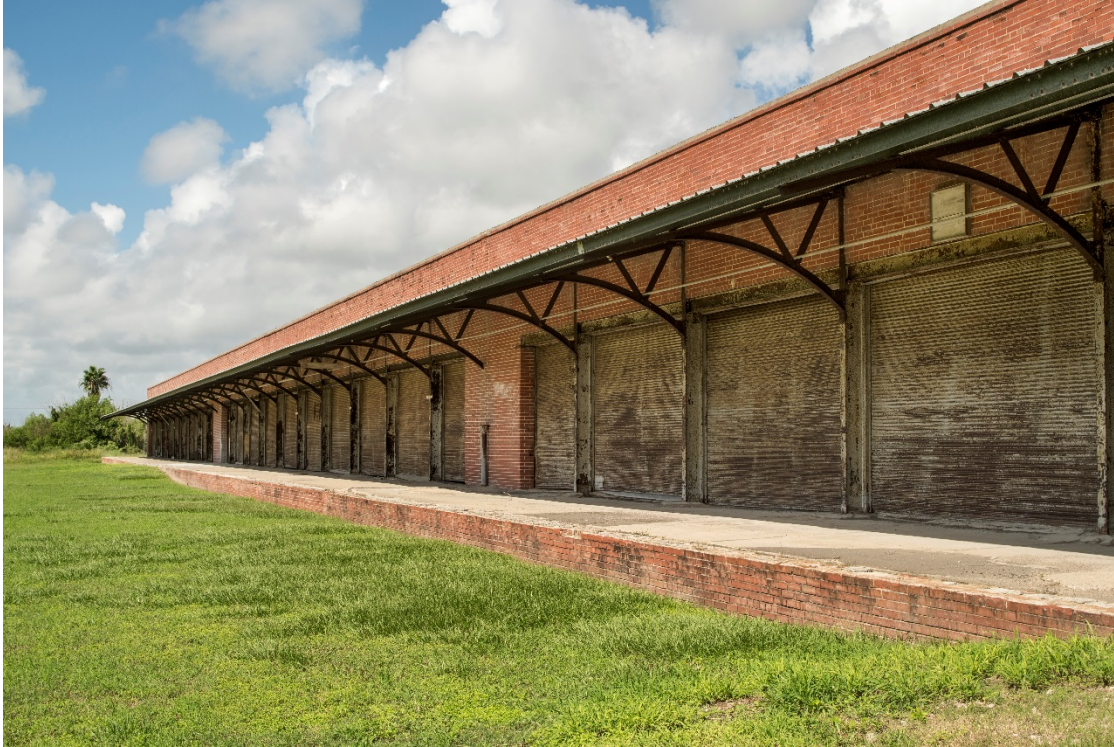
Photo 8: South elevation warehouse. Looking northwest.
