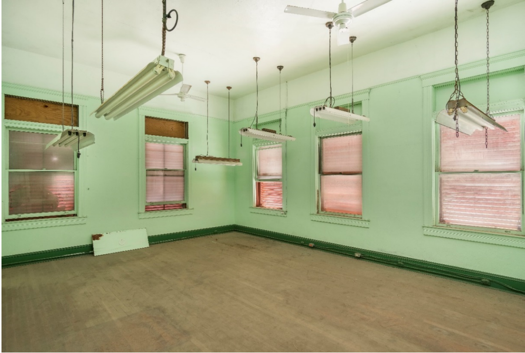
Photo 14: Second story north office. Looking northeast.
