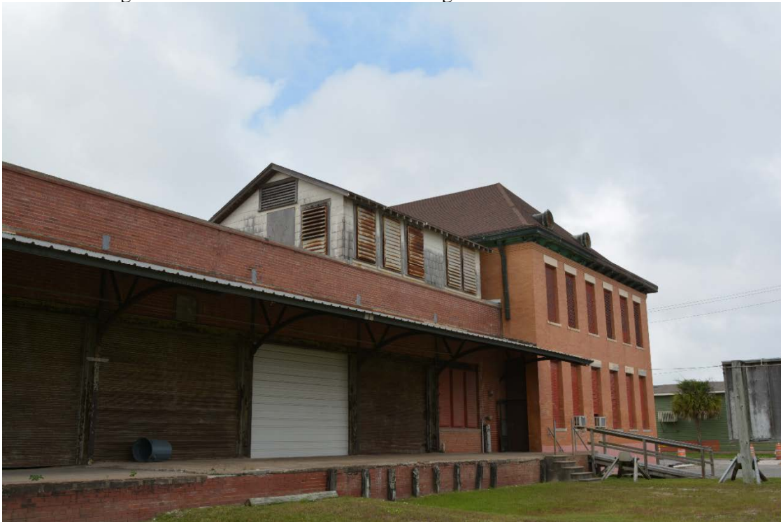
Photo 5: Cottage and west elevation of office. Looking northeast.
