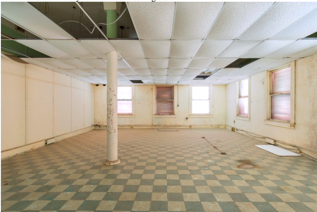
Photo 13: Second story south office. Looking east.
