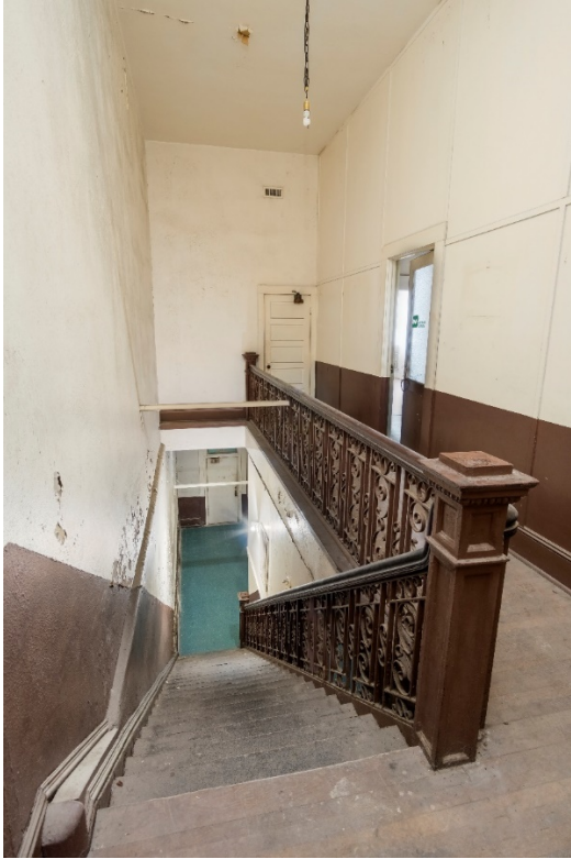
Photo 12: Office interior stairway second story. Looking north.
