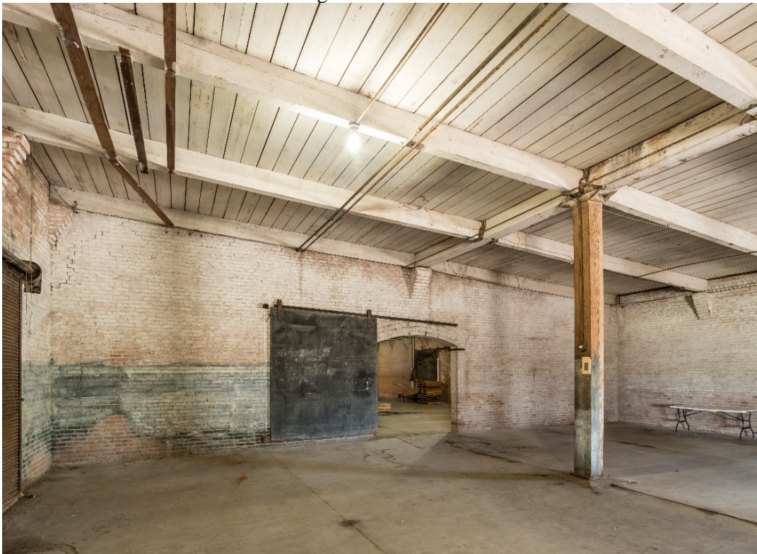
Photo 15: Warehouse interior. Looking west.
