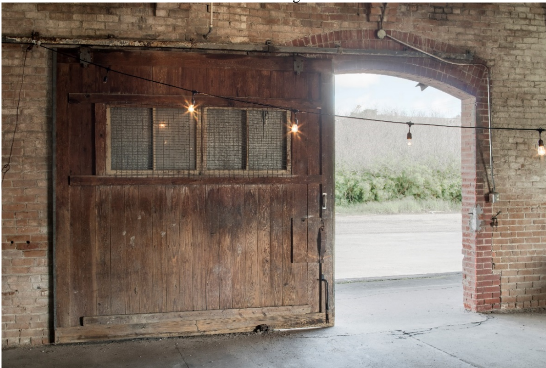
Photo 17: Warehouse north exterior door. Looking north.
