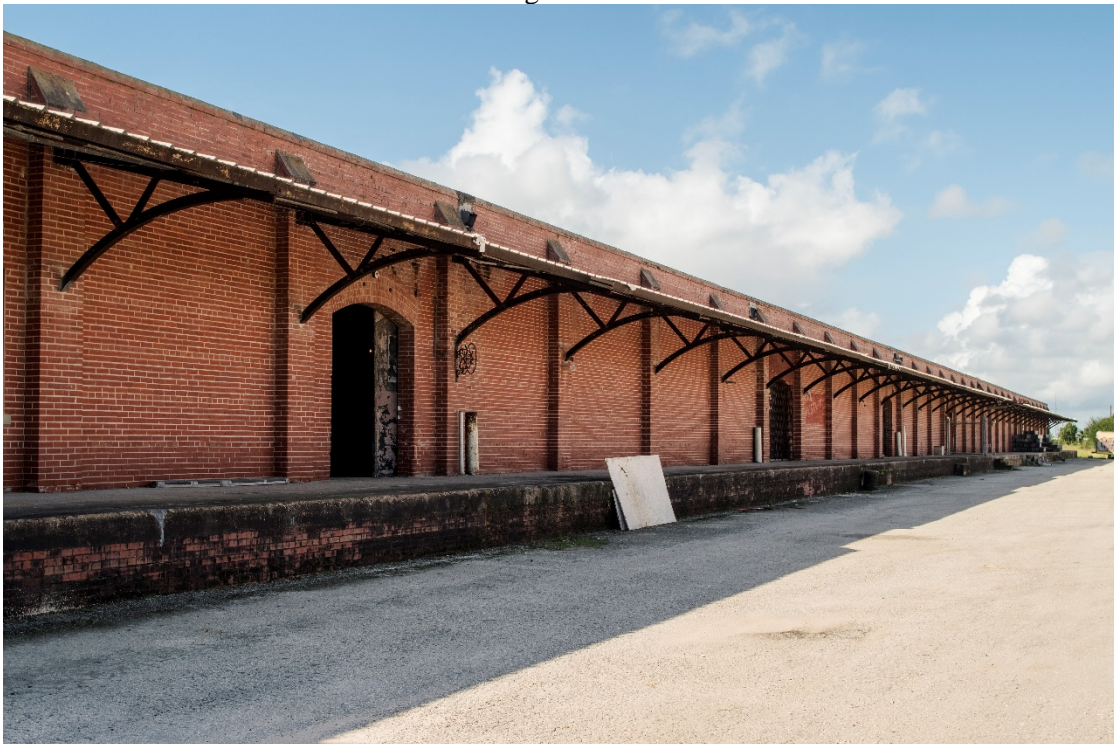
Photo 9: North elevation warehouse. Looking southwest.
