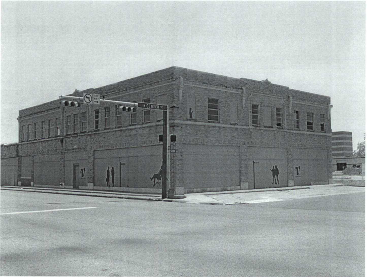
Figure 5. The Vandergriff Building before rehabilitation, ca. 2003.
