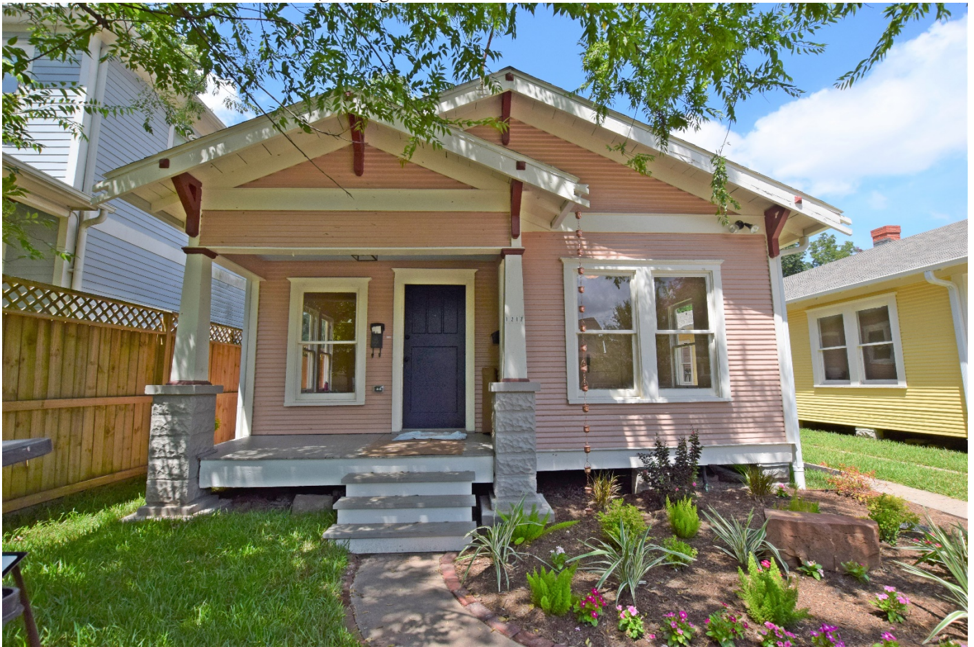
Photo 3: East elevation of 1217 Tulane, looking west.
