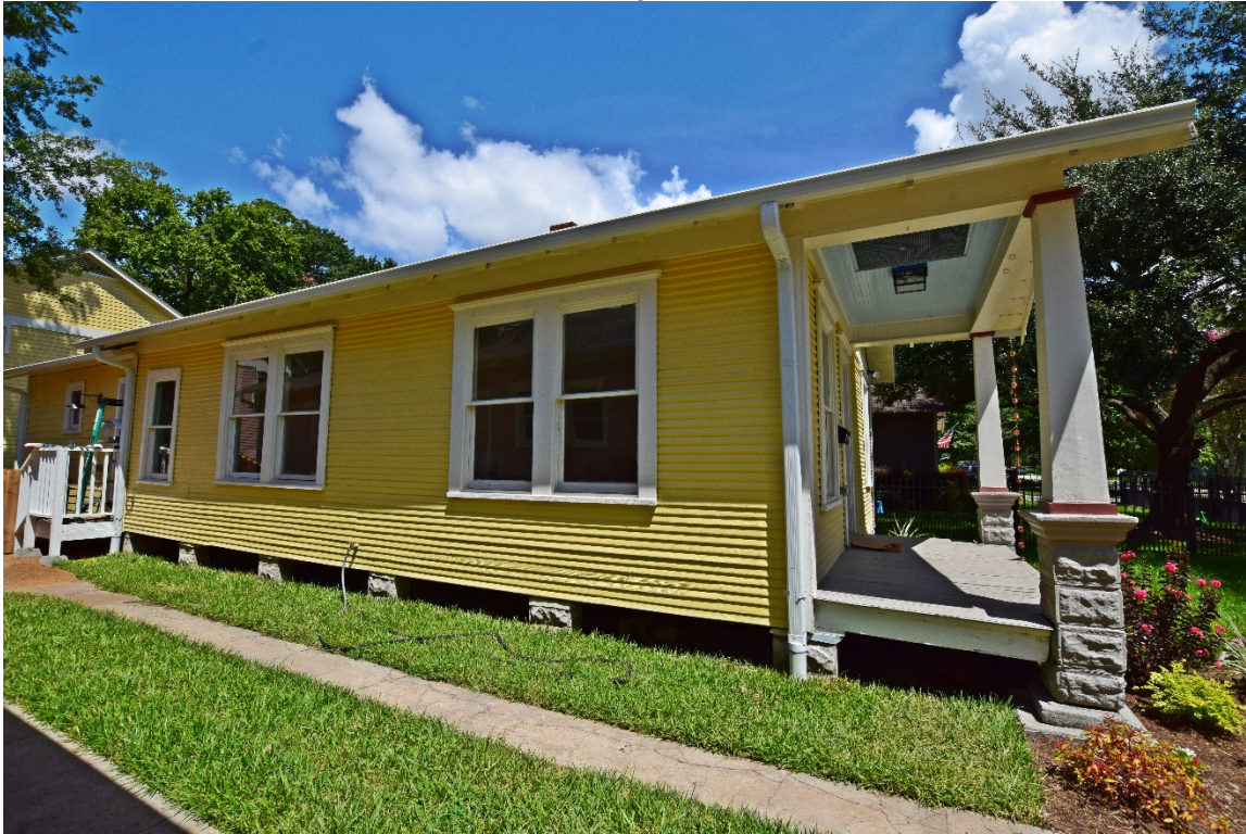
Photo 12: South elevation of 1219 Tulane, looking north.
