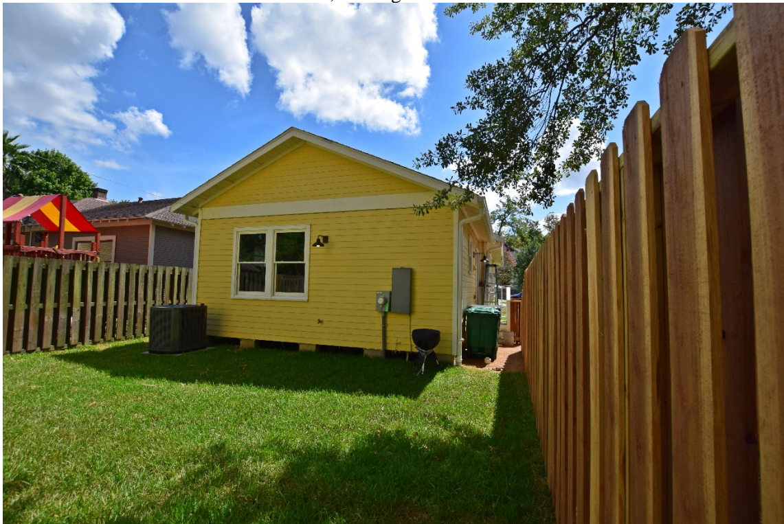
Photo 14: North elevation of 1219 Tulane, looking west.
