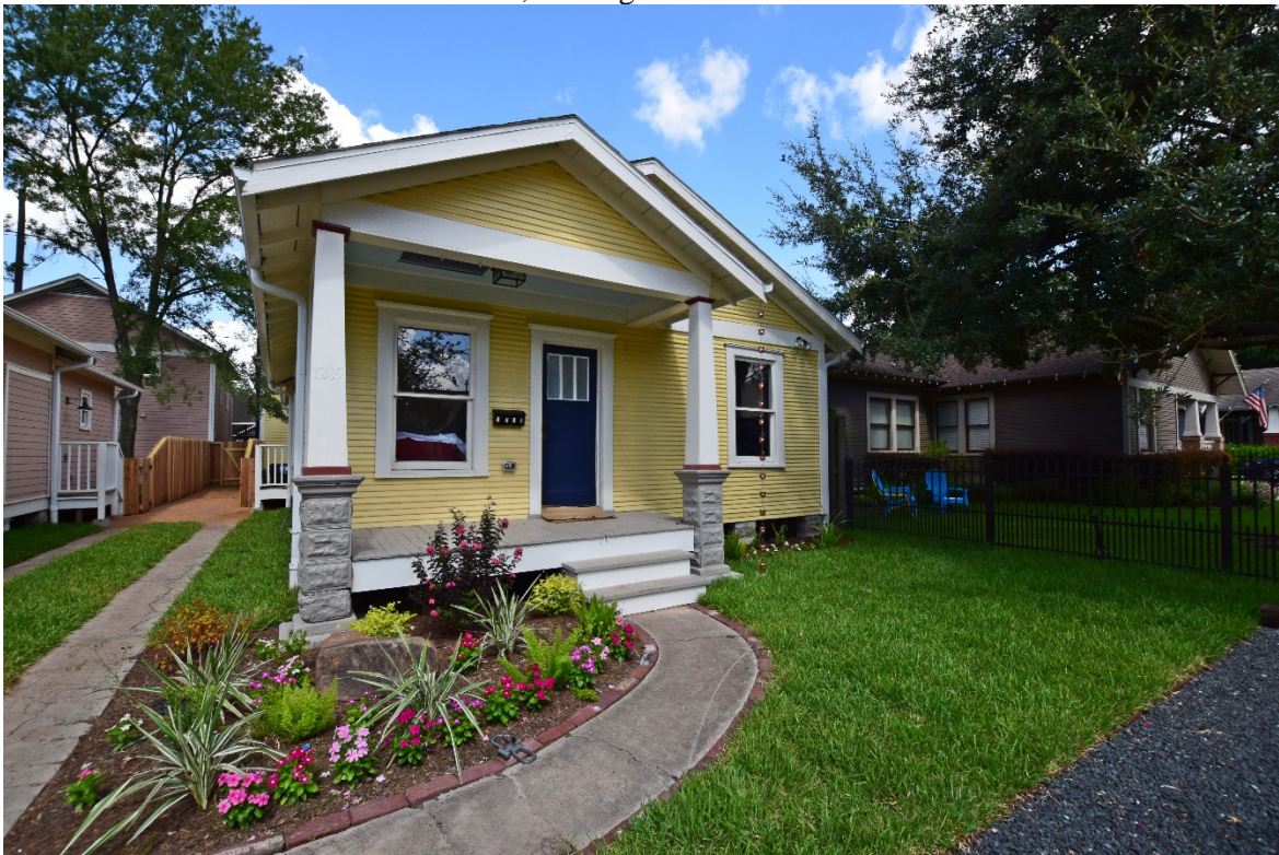
Photo 11: East elevation of 1219 Tulane, looking west.
