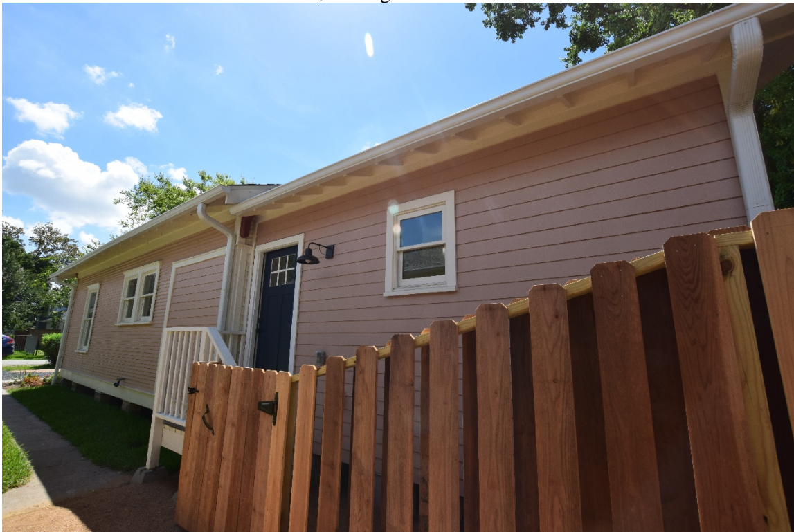
Photo 6: West elevation of 1217 Tulane, looking east.
