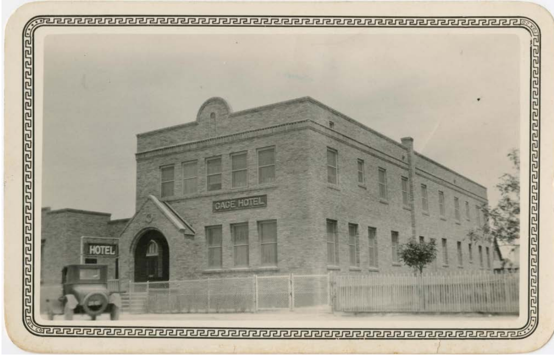
Figure 12. Historic photograph depicting south and east elevations, c. 1930. Source: Recorded Texas Historic Landmark file, Texas Historical Commission.
