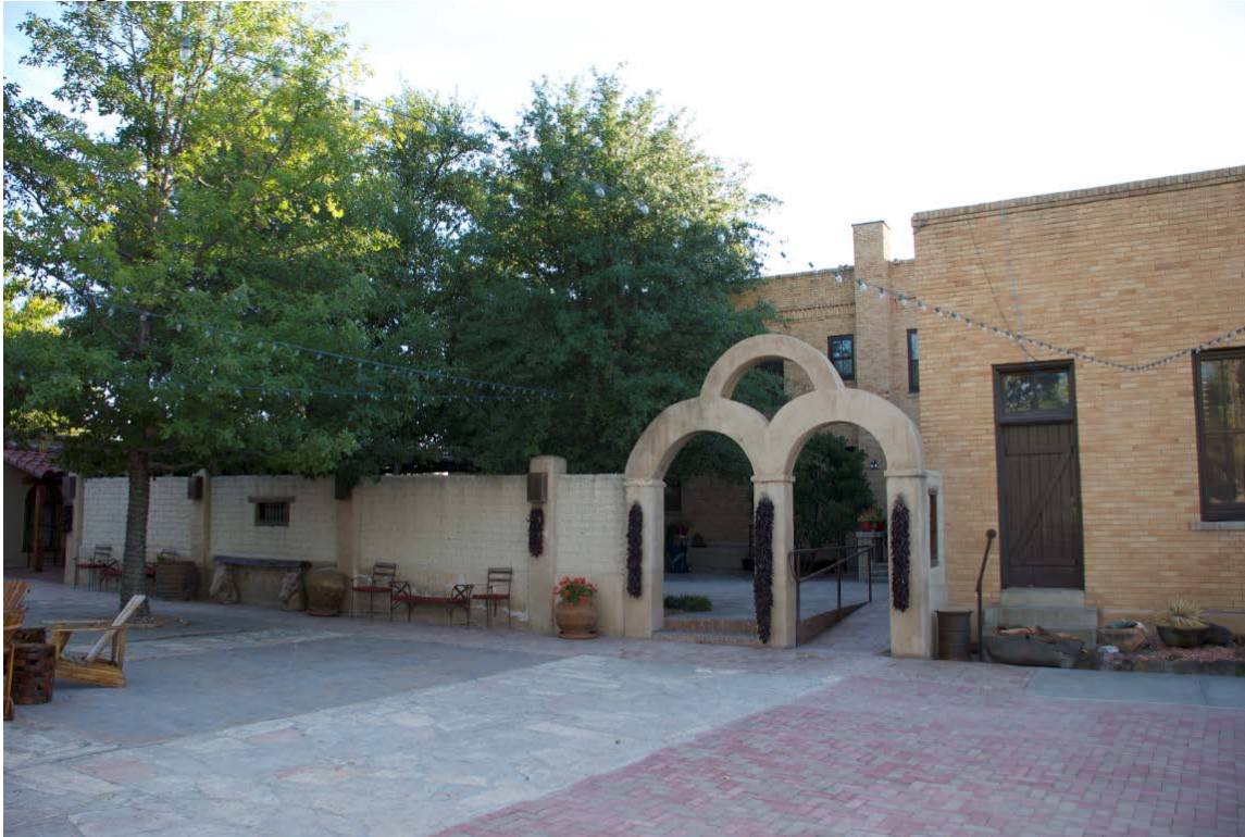
Photo 4. West elevation, camera facing east. The stucco wall and gate on the west elevation separate the historic hotel building from modern additions.
