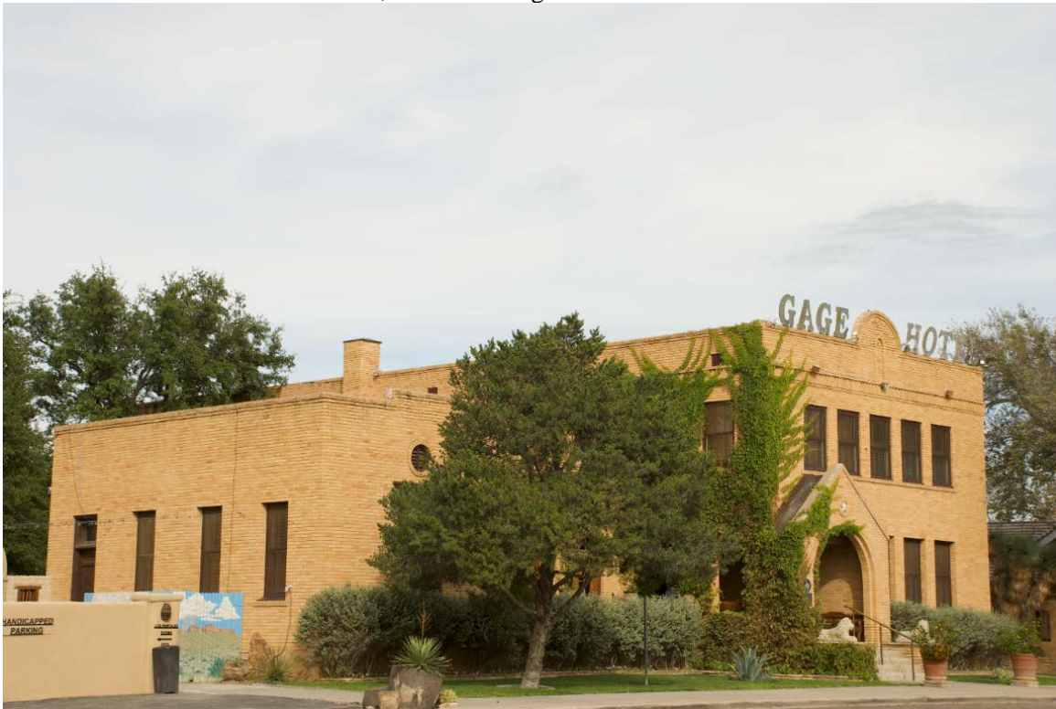
Photo 3. West and south elevations, camera facing northeast.
