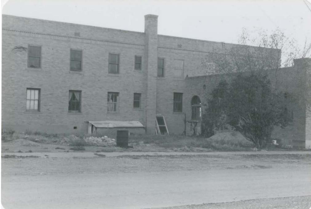
Figure 19. Photo of hotel, during rehabilitation, c. 1980. Source: Recorded Texas Historic Landmark file, Texas Historical Commission.
