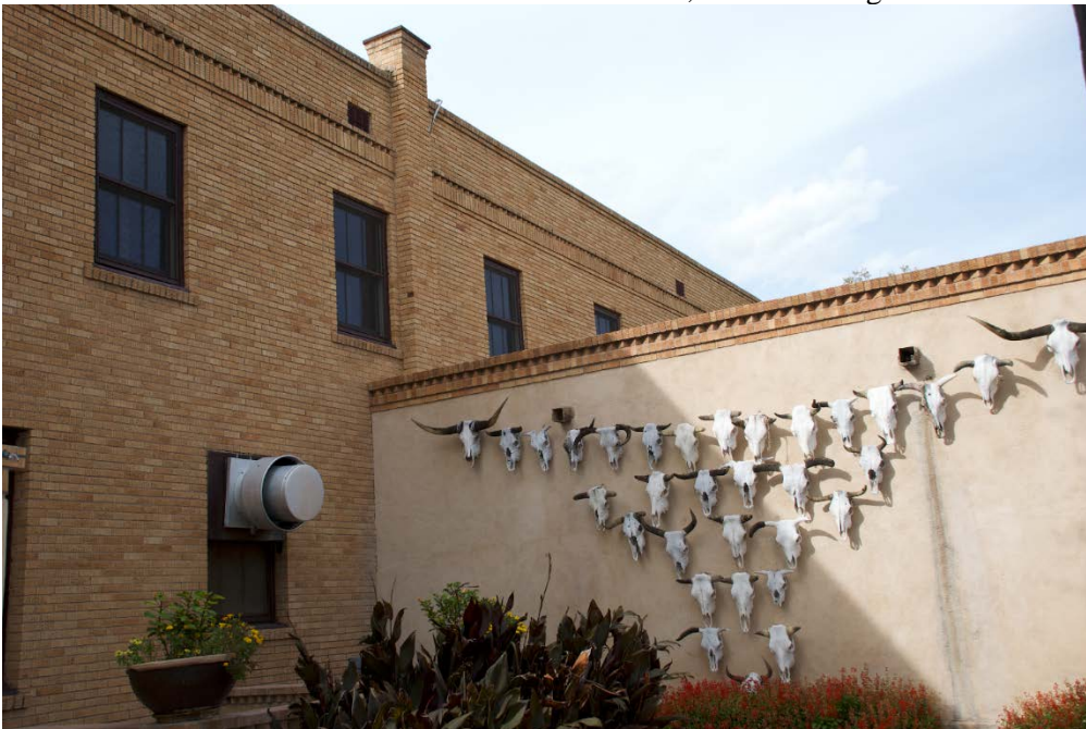
Photo 9. Junction of historic hotel and 1990s addition, camera facing northwest.
