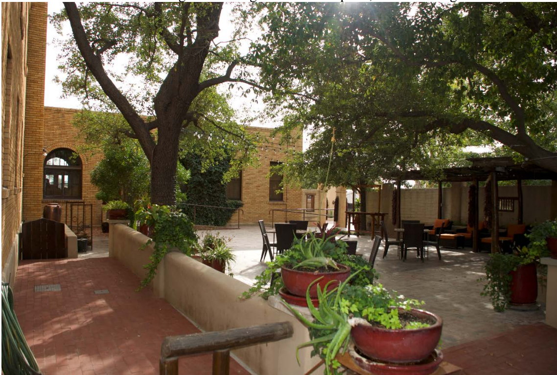
Photo 5. North elevation of Gage hotel wing inside walled patio, camera facing south.
