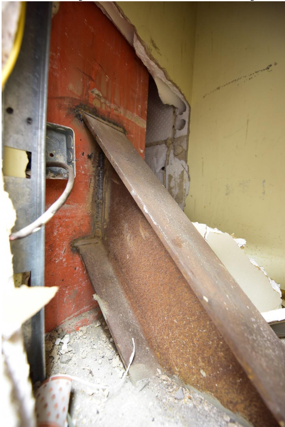
Photo 15. Reinforcing steel added after 1970 tornado. Camera facing southeast.
