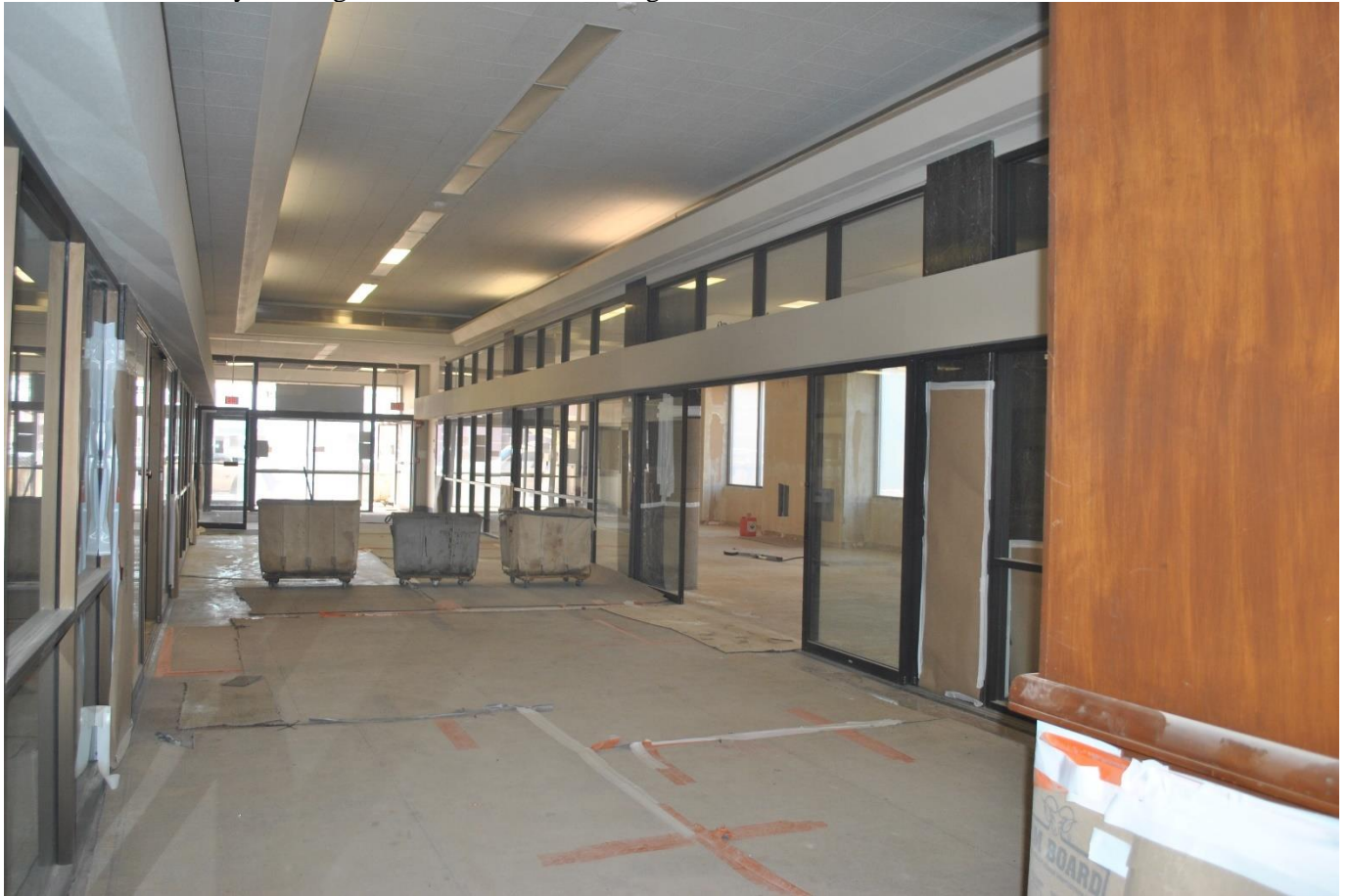
Photo 8. Main lobby on the ground floor. Camera facing south
