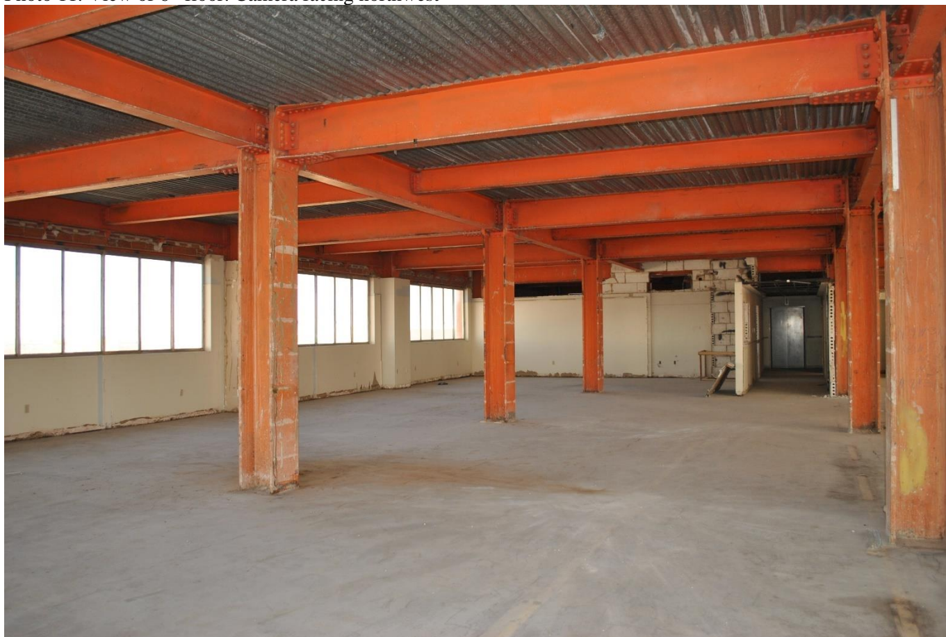
Photo 11. View of 6 th floor. Camera facing northwest
