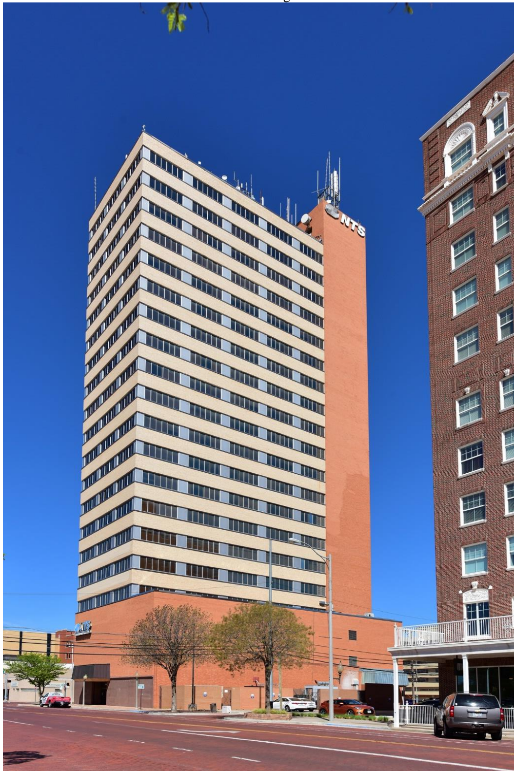
Photo 4. South and east elevations. Camera facing northwest.
