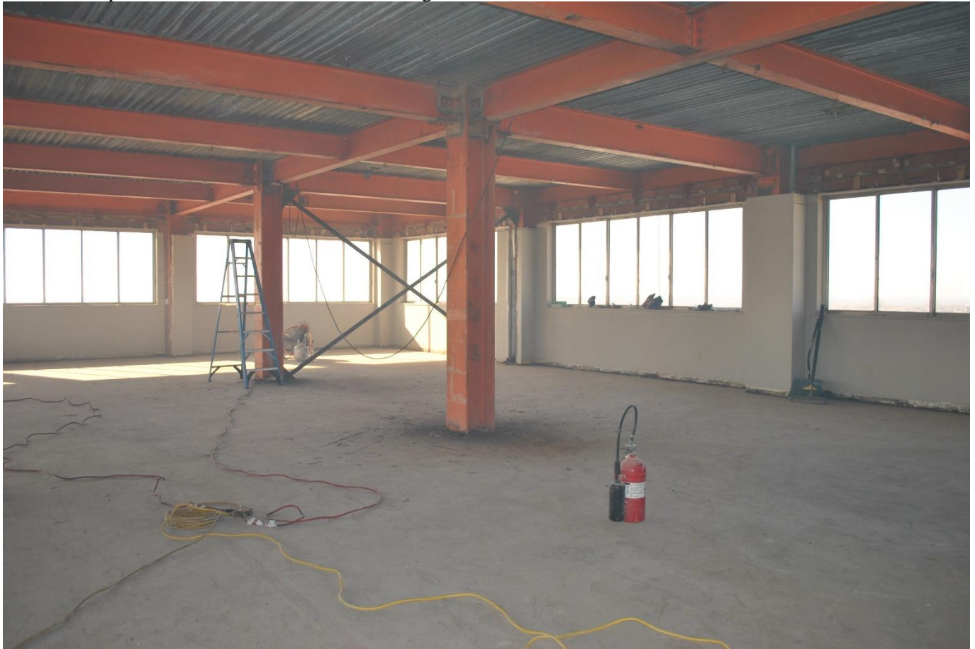
Photo 13. Open office on 14 th floor. Camera facing southwest.
