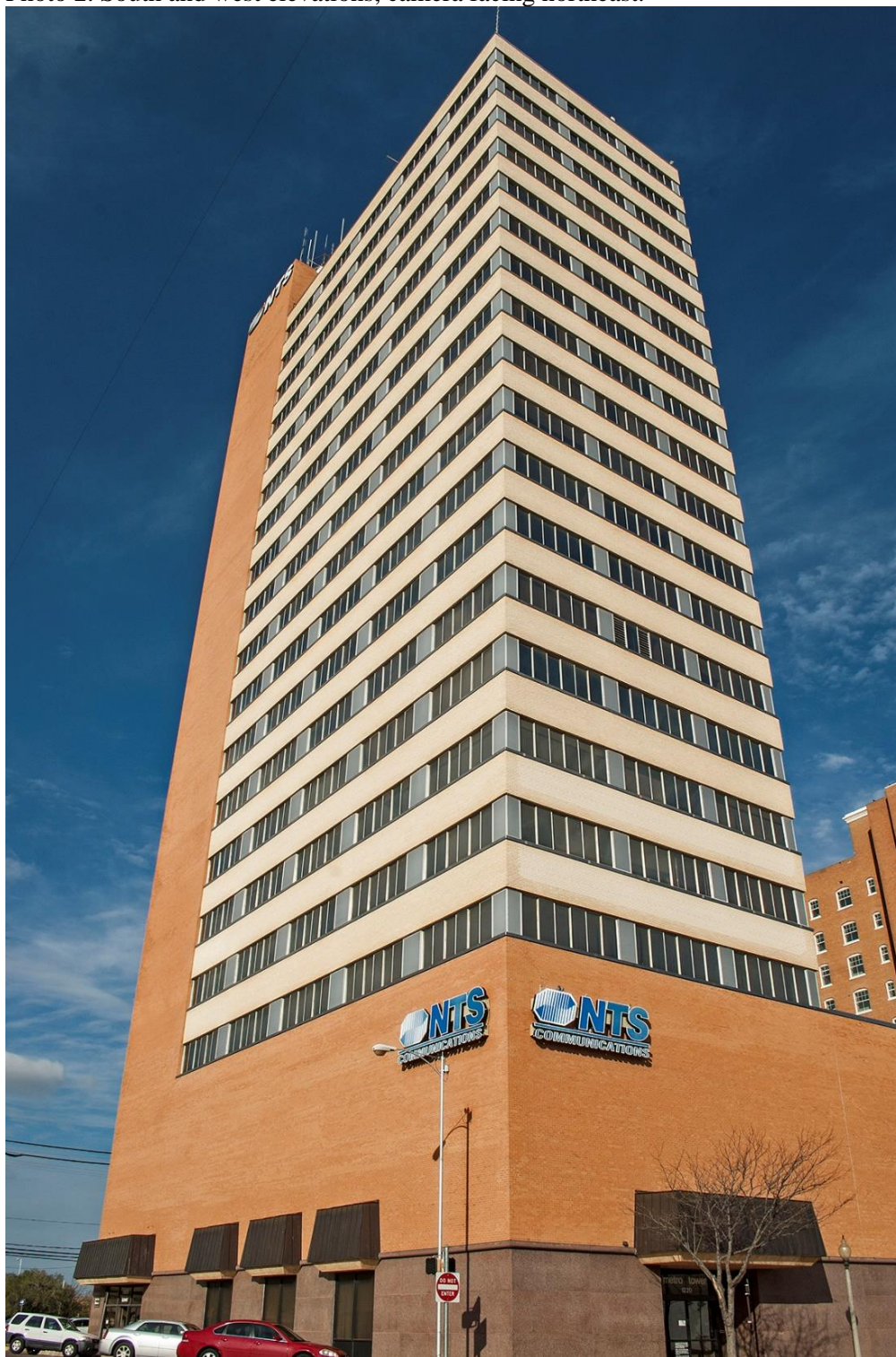
Photo 2. South and west elevations, camera facing northeast.
