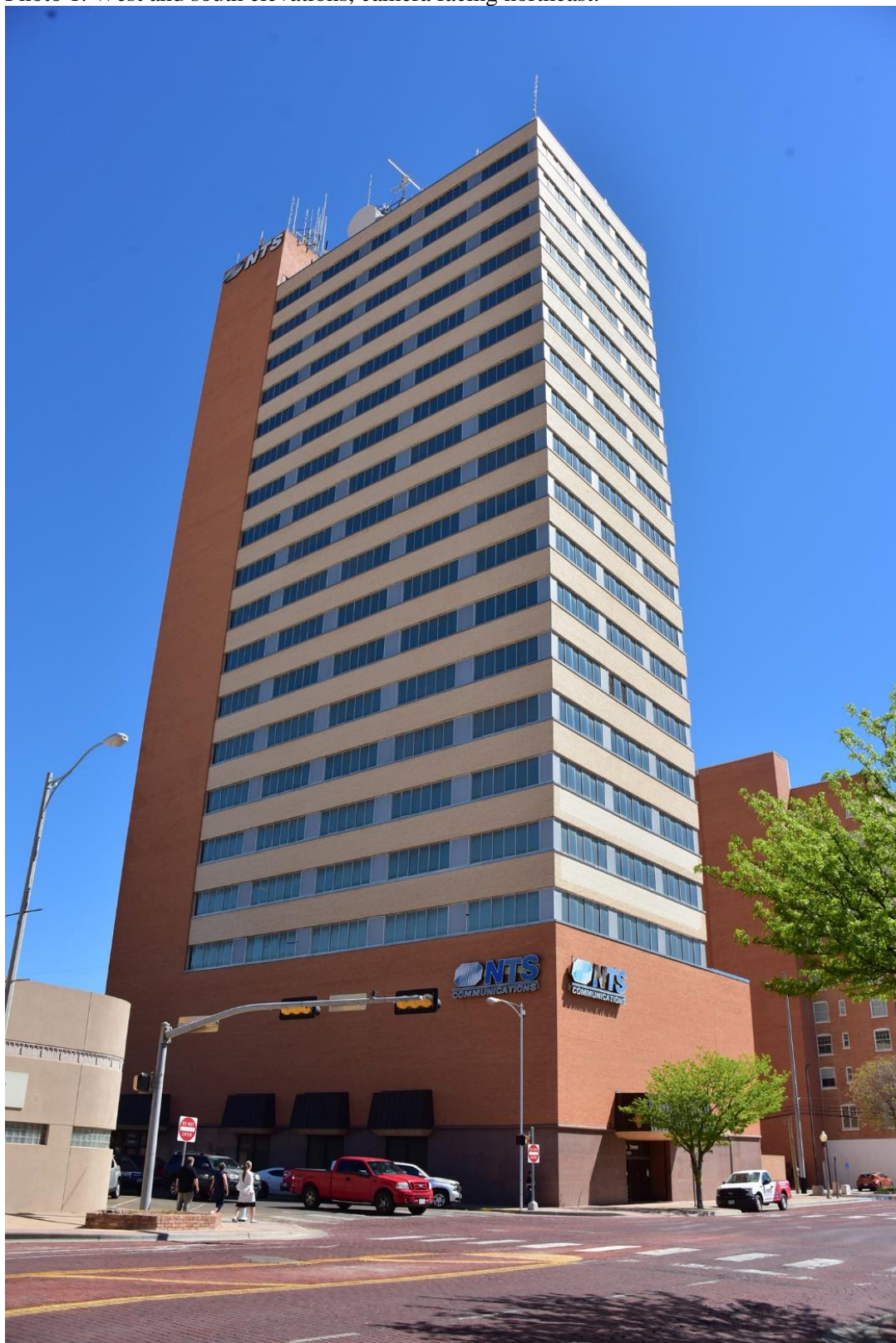
Photo 1. West and south elevations, camera facing northeast.
