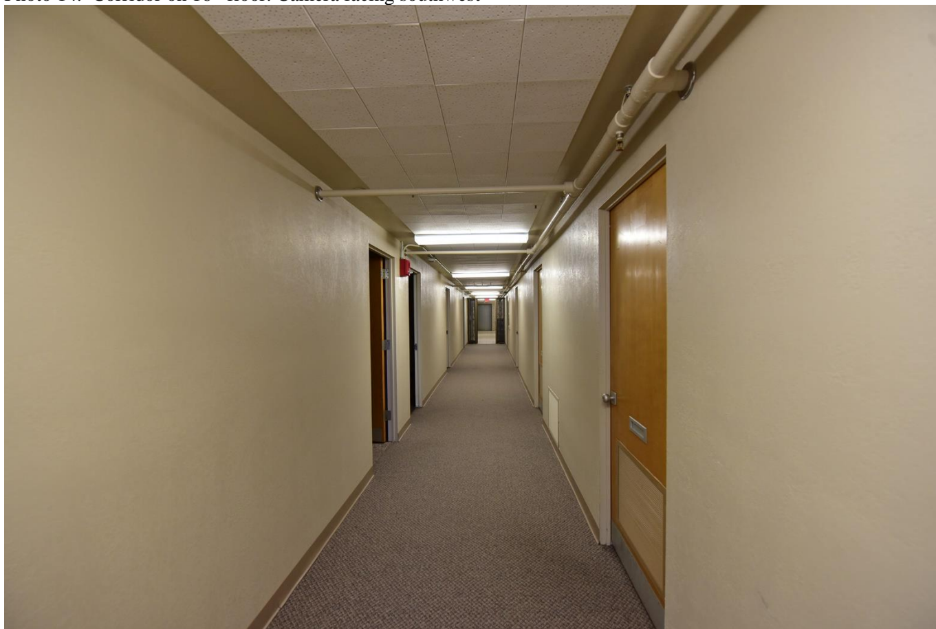
Photo 14. Corridor on 16 th floor. Camera facing southwest
