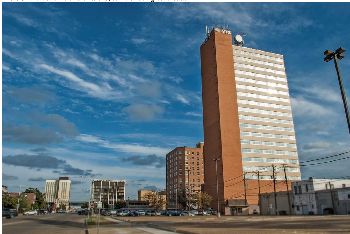
Photo 3. West and north elevations, camera facing southeast.
