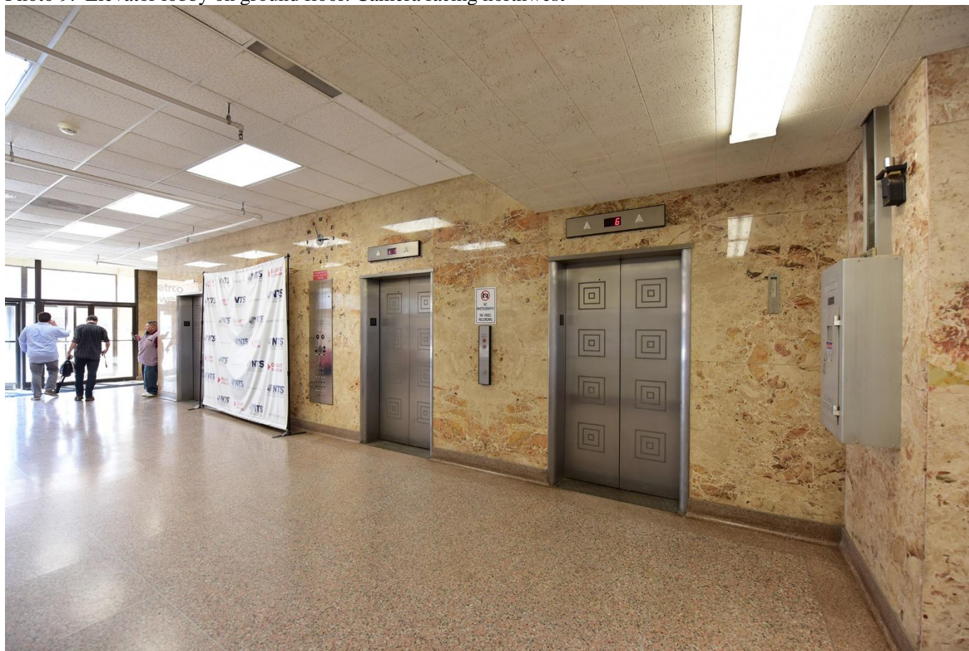
Photo 9. Elevator lobby on ground floor. Camera facing northwest
