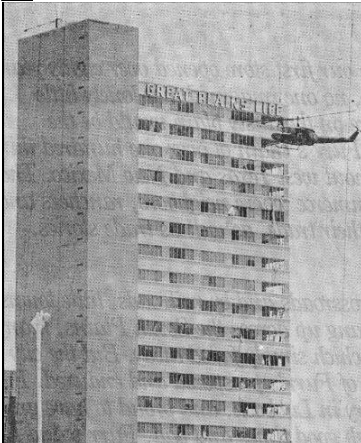
Figure 10. Great Plains Life Insurance Company Building following tornado damage in 1970. Source: https://www.lubbockonline.com/1970-lubbock-tornado/20-years-later/2012-02-03/fear-collapse-surrounded-landmark
