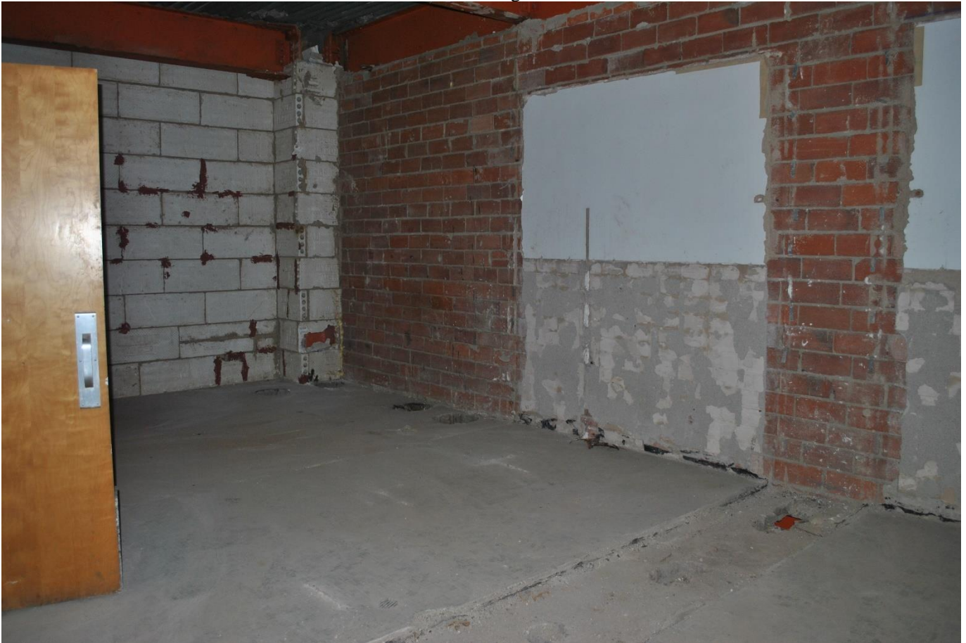
Photo 12. View of removed historic restroom. Camera facing west
