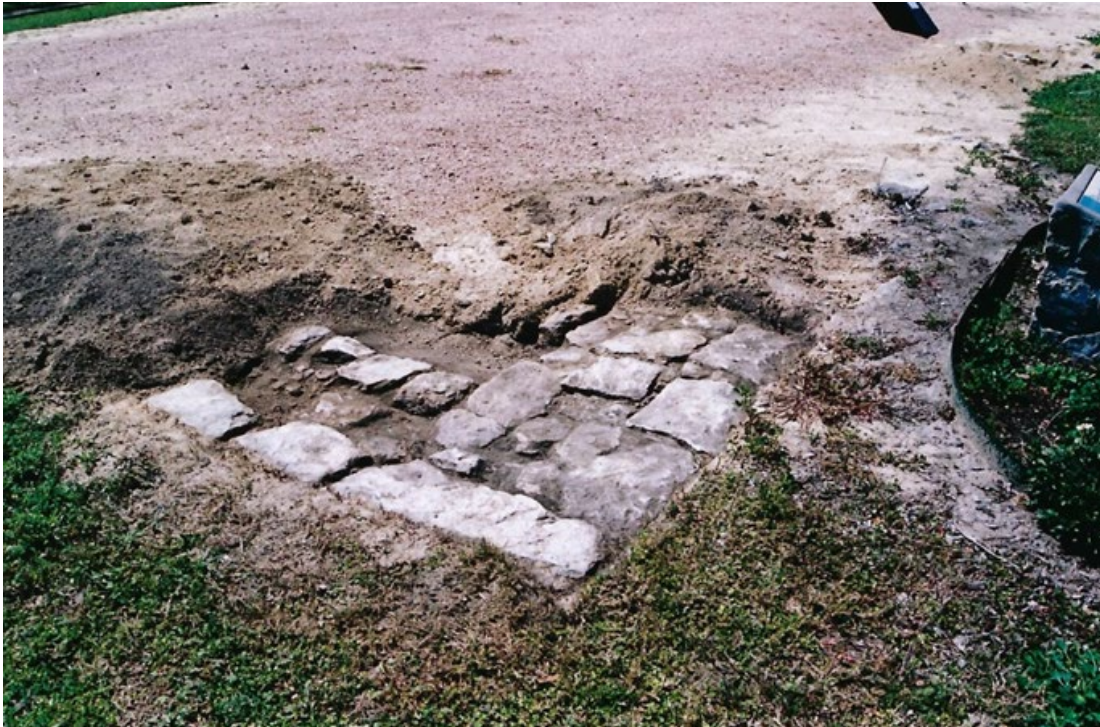
Photo 4: Photograph of the exposed limestone platform of the bell pole, constructed in 1882 (Contributing Resource 1F).
