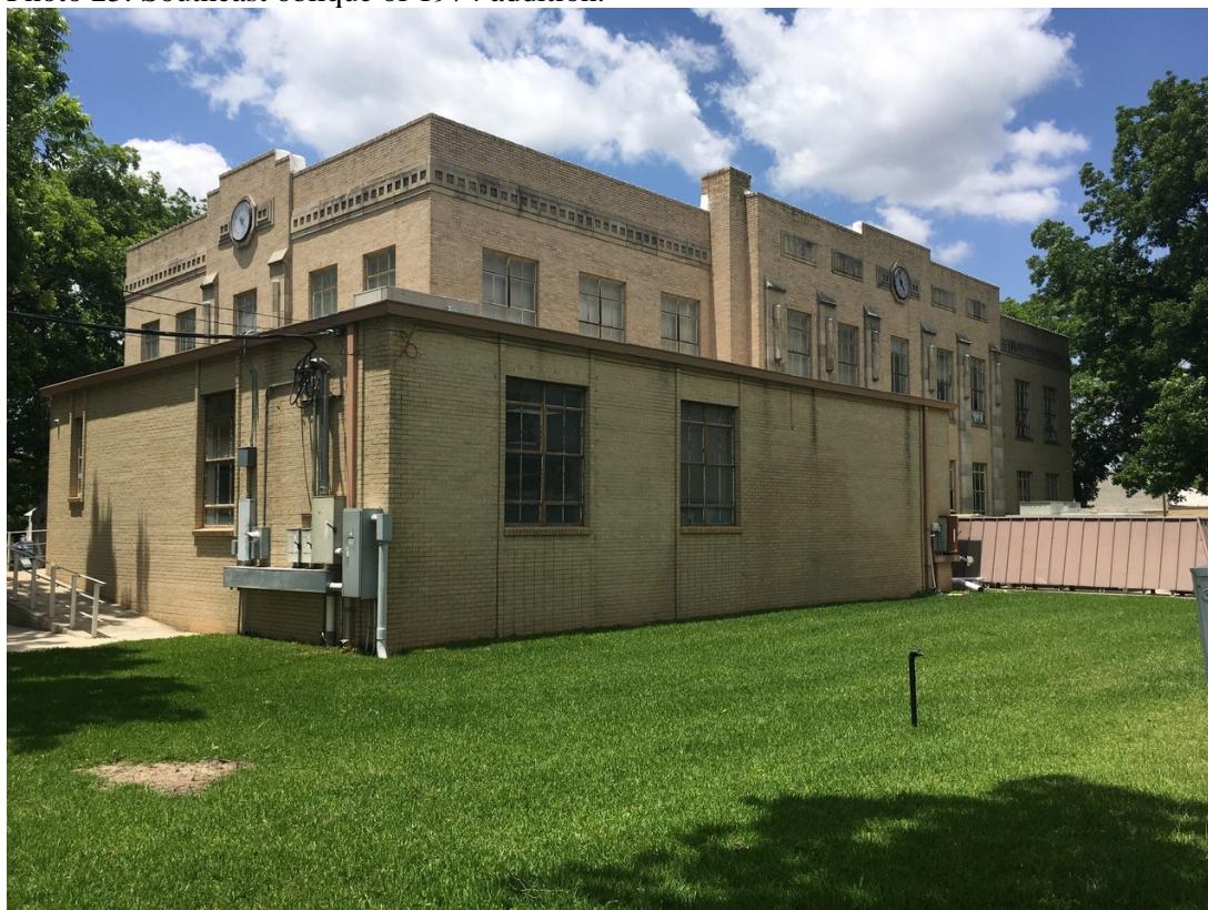
Photo 25: Southeast oblique of 1974 addition.
