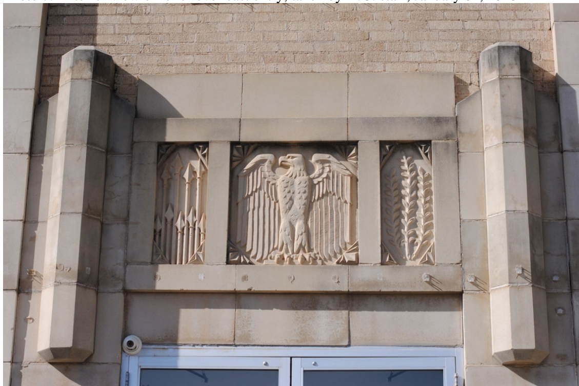
Photo 7: Exterior view of relief over east entry, taken by H.G. staff, January 04, 2018
