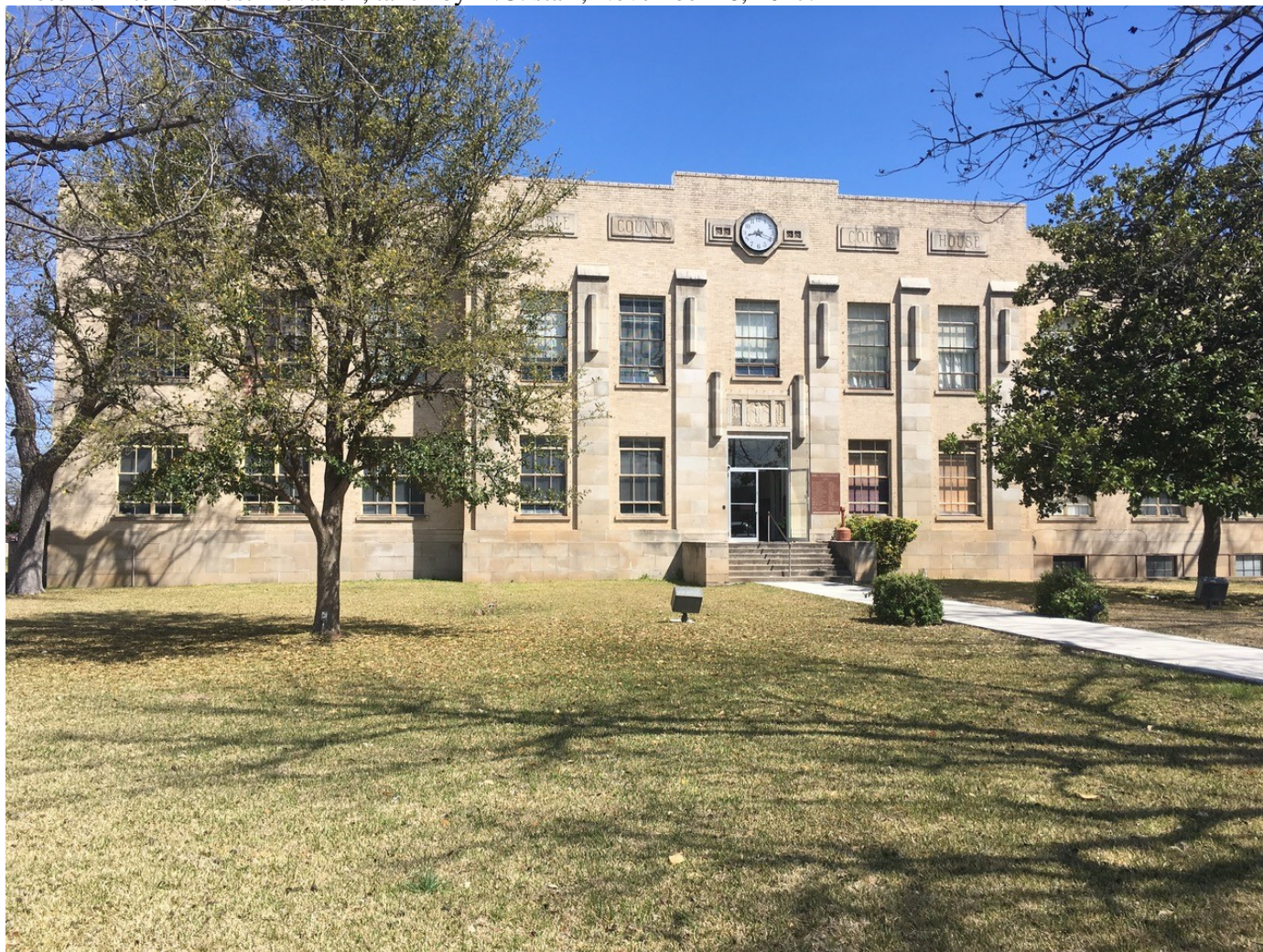
Photo 1: Exterior West Elevation, taken by H.G. staff, November 28, 2017.
