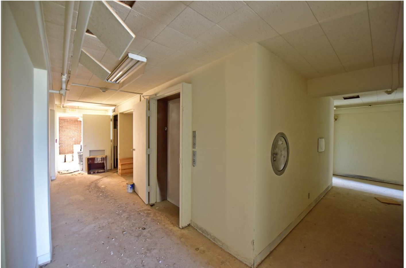
Photo 21. Second floor, corridor/elevators, view southwest.
