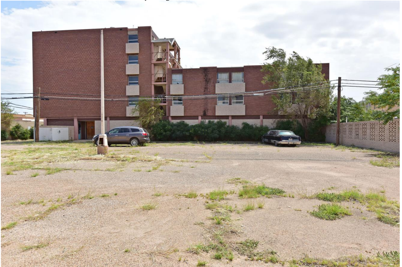
Photo 6. West elevations, view east across parking lot.
