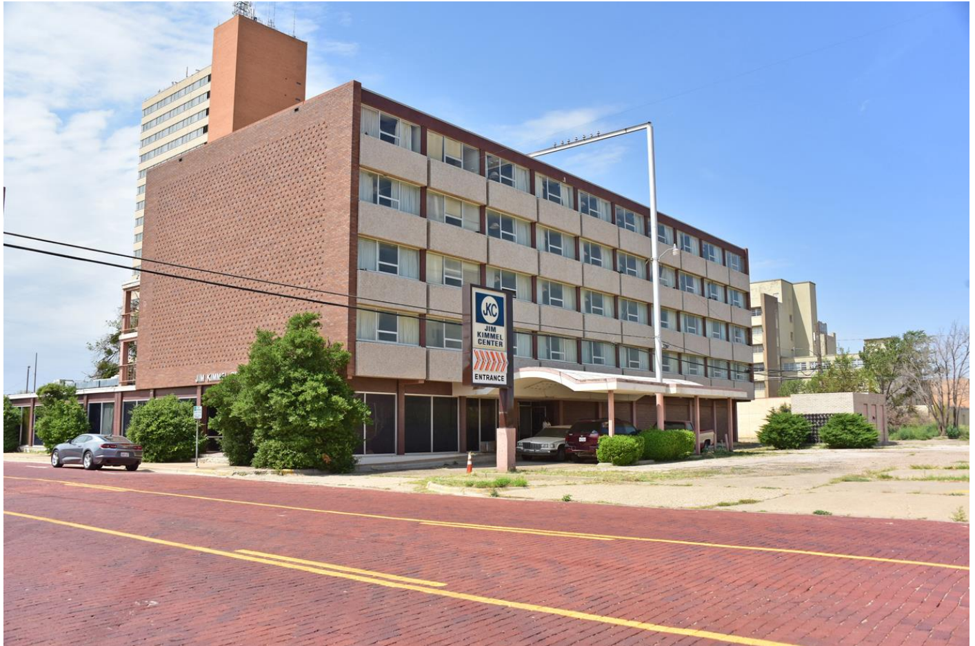
Photo 3. East and north elevations, view southwest.
