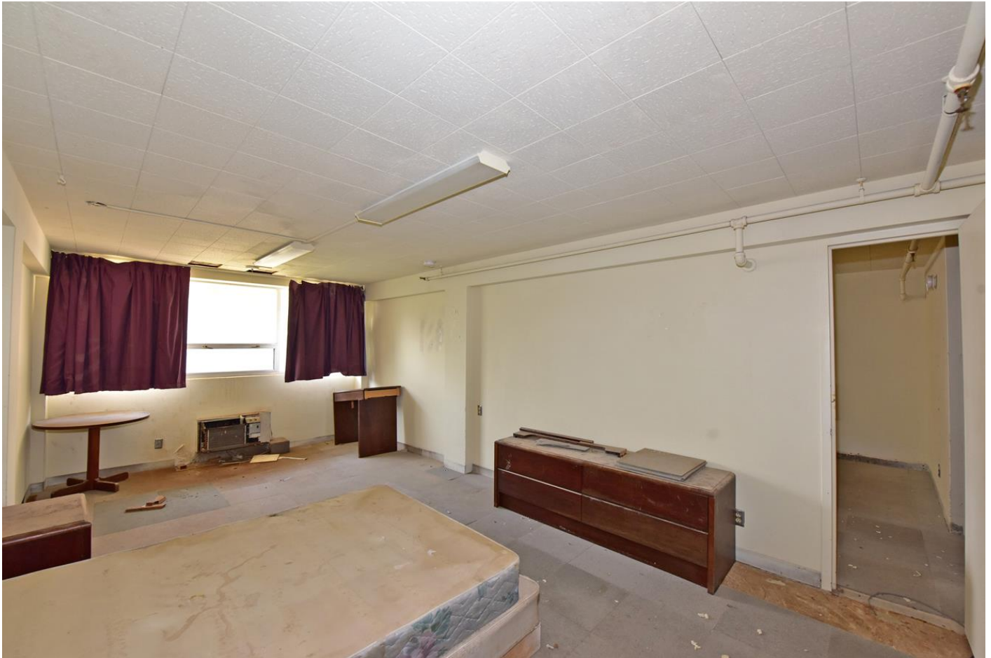
Photo 24. Second floor, Unit 212, view southwest.
