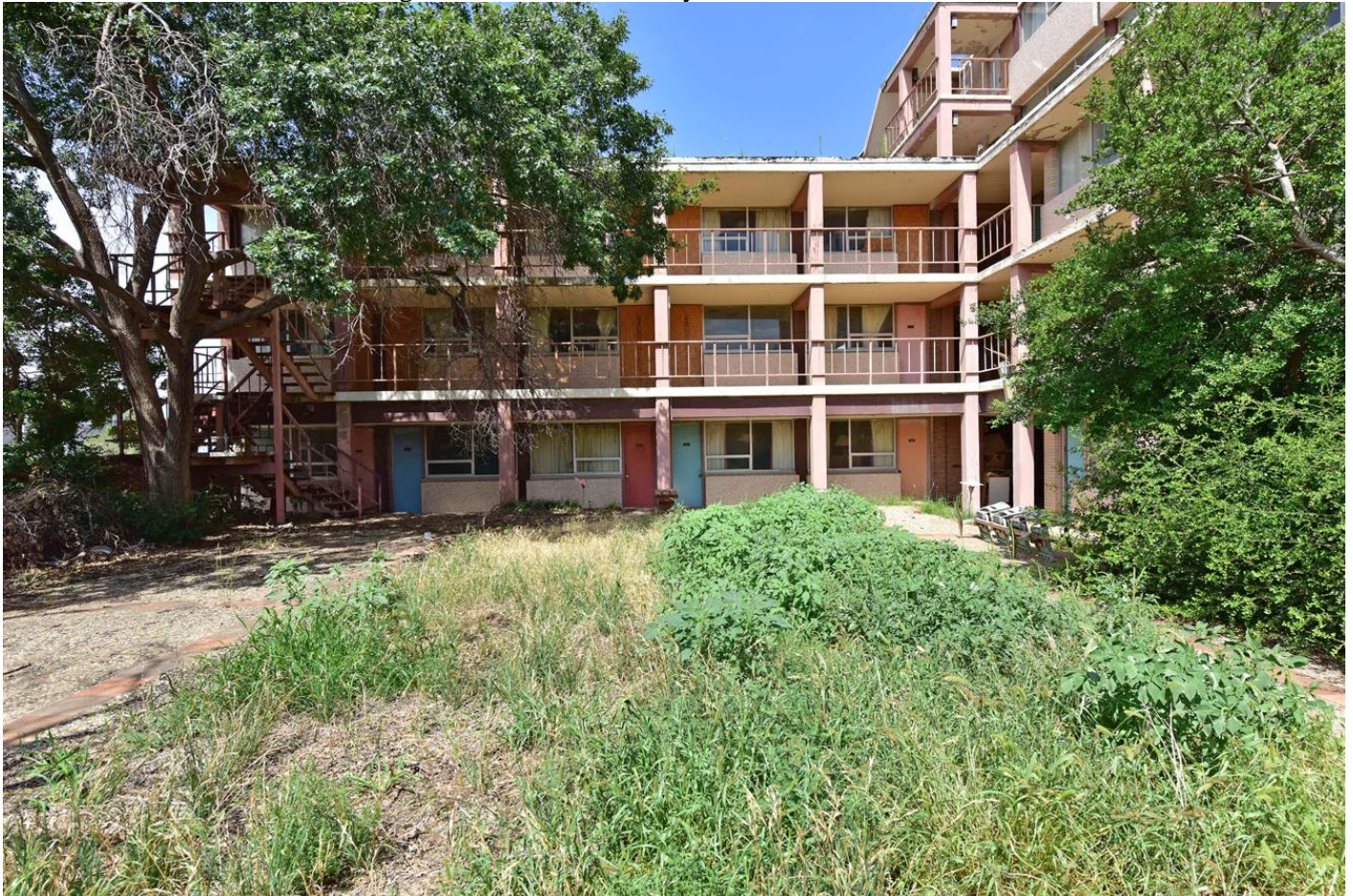
Photo 8. East elevation of west wing, view west across courtyard.
