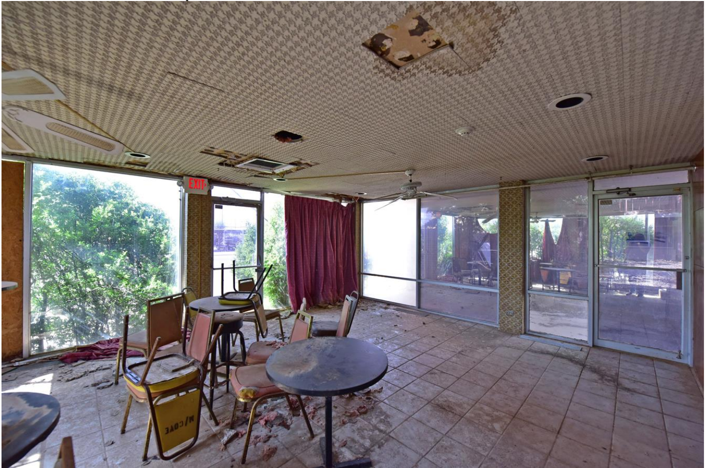
Photo 19. First floor, coffeeshop, view southwest.
