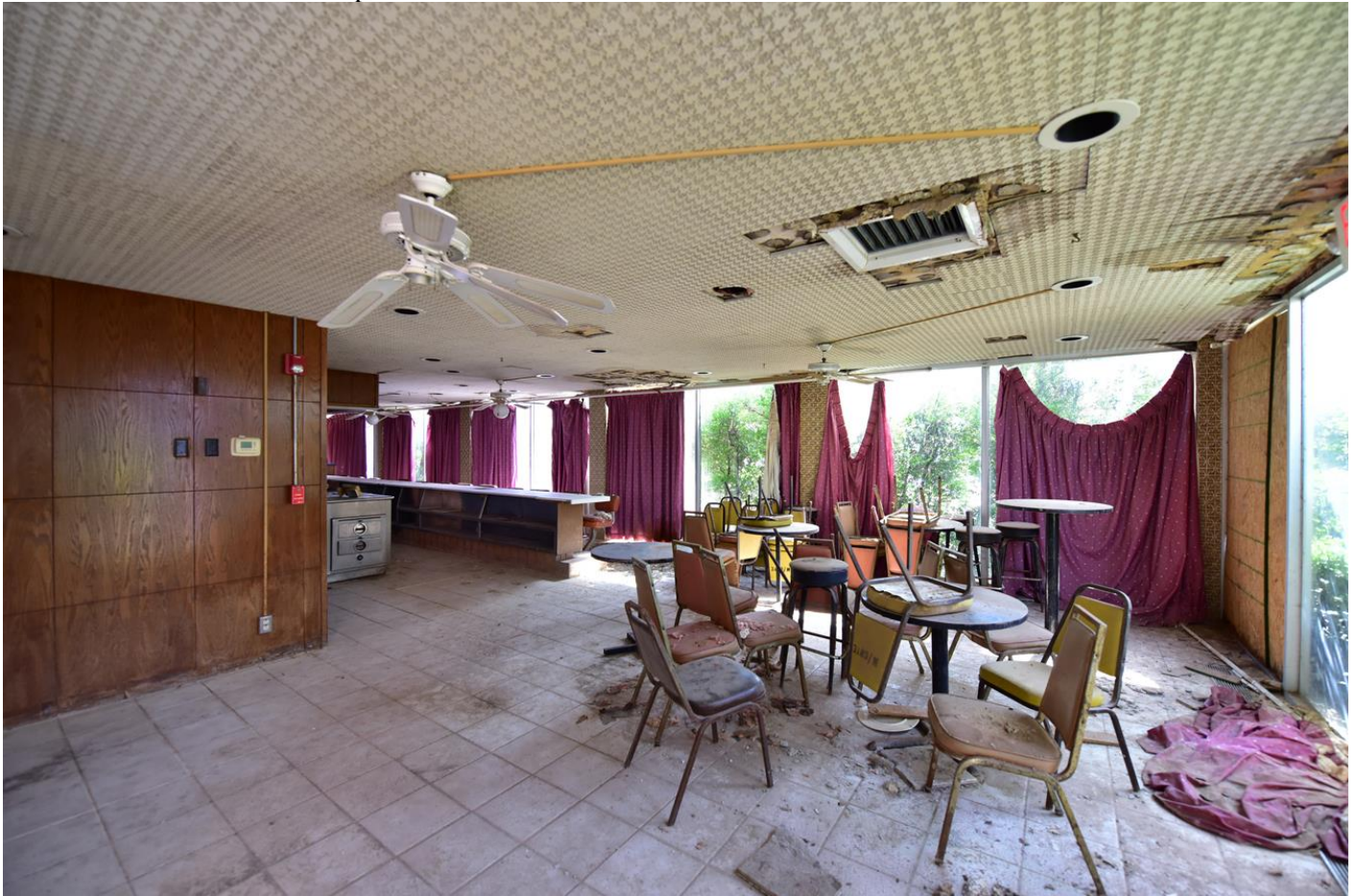
Photo 18. First floor, coffeeshop, view east-northeast.
