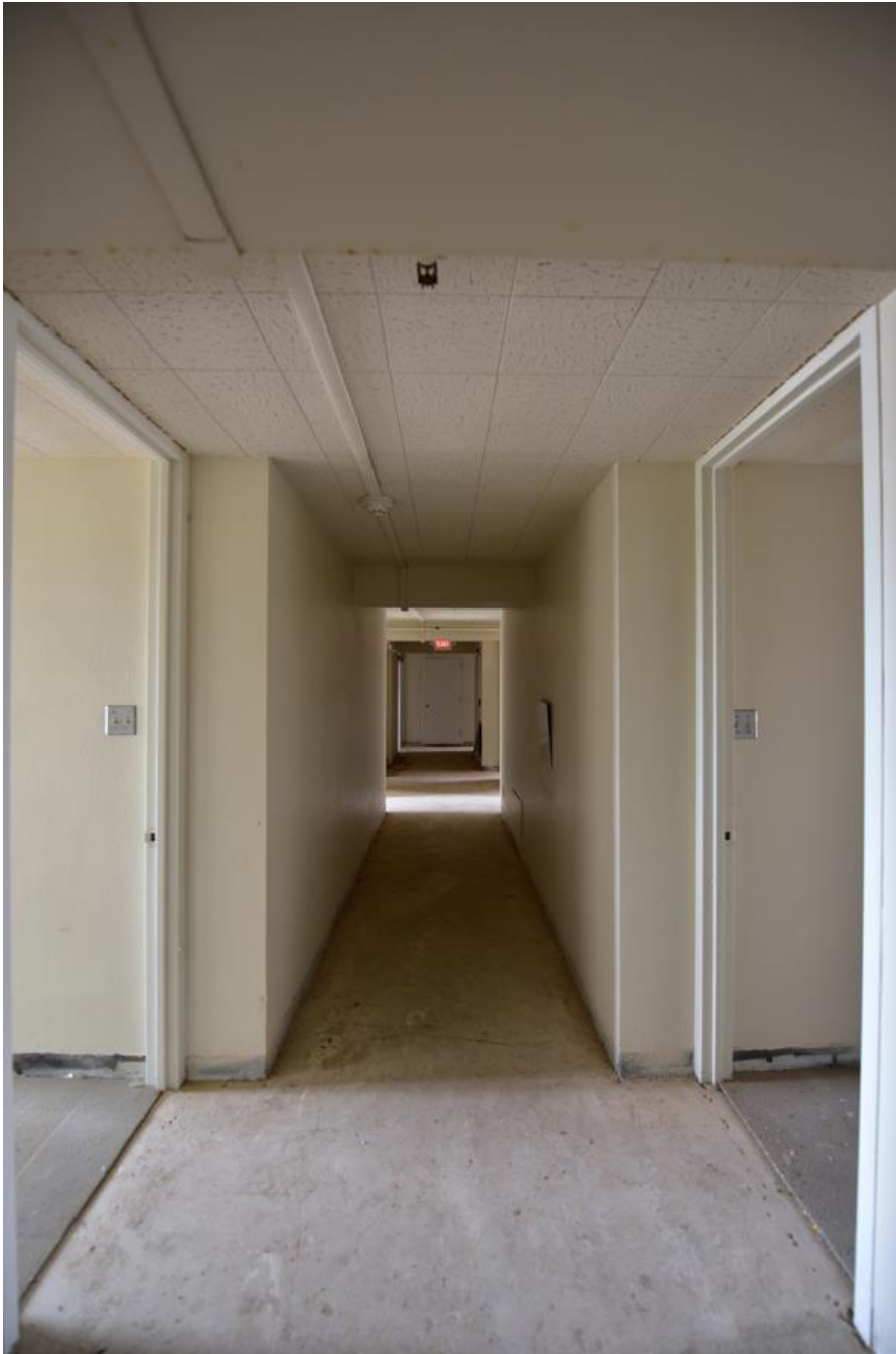
Photo 20. Fourth floor, main corridor, view east.
