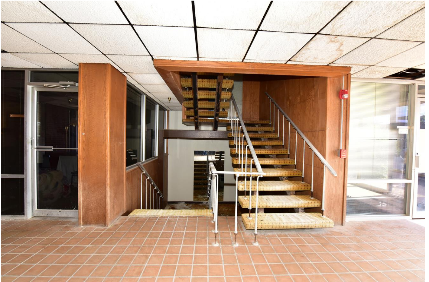
Photo 15. First floor, main stair, view north.
