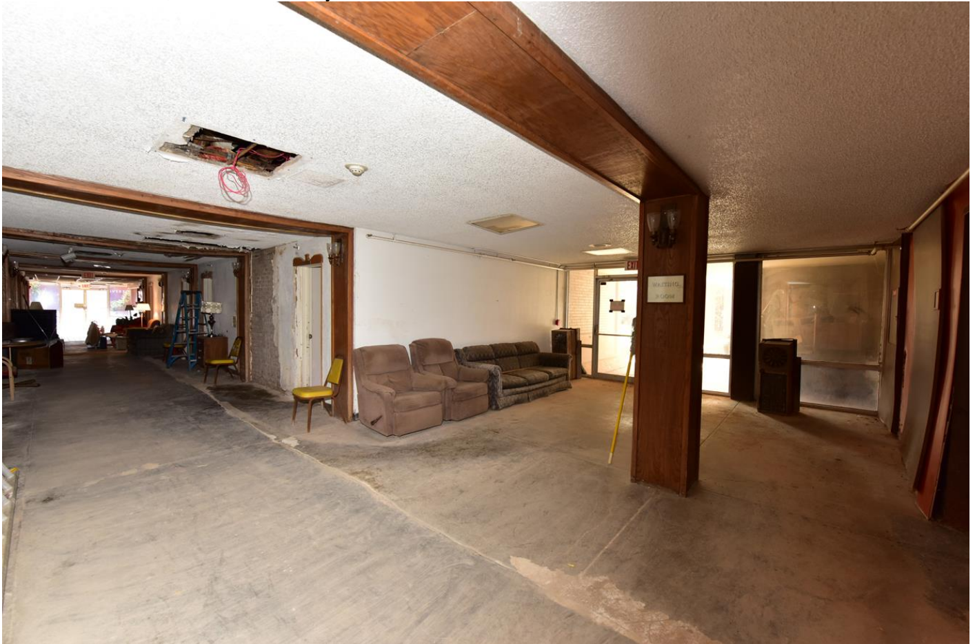
Photo 17. First floor, elevator/west lobby, view southeast.
