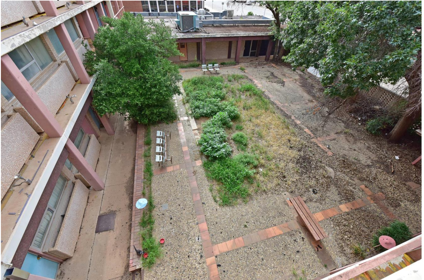
Photo 10. Courtyard, view east from west wing, third story balcony.
