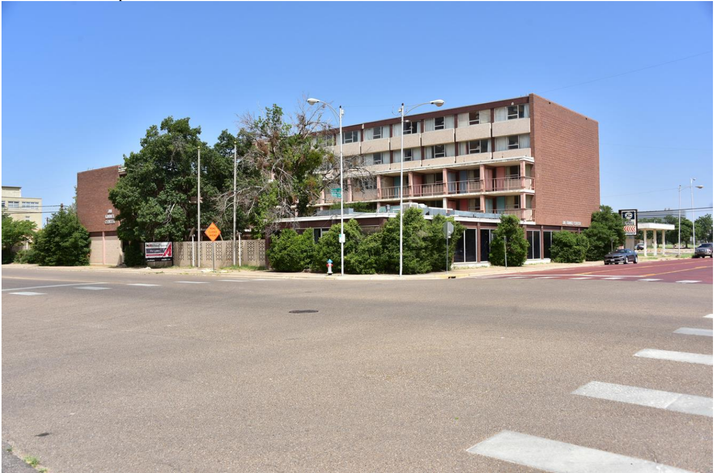
Photo 2. South and partial east elevations, view northwest.
