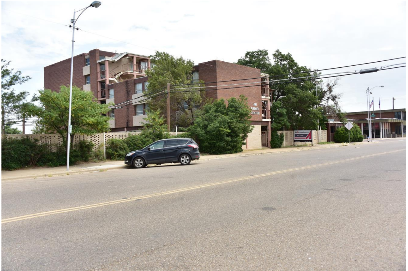
Photo 7. Partial west and south elevations, view northeast.
