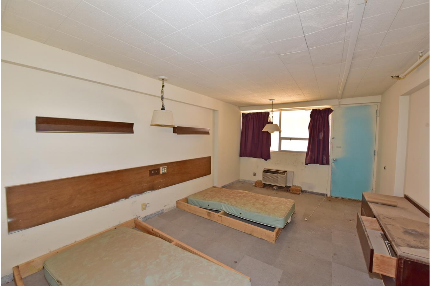
Photo 23. Second floor, Unit 216, view southeast.
