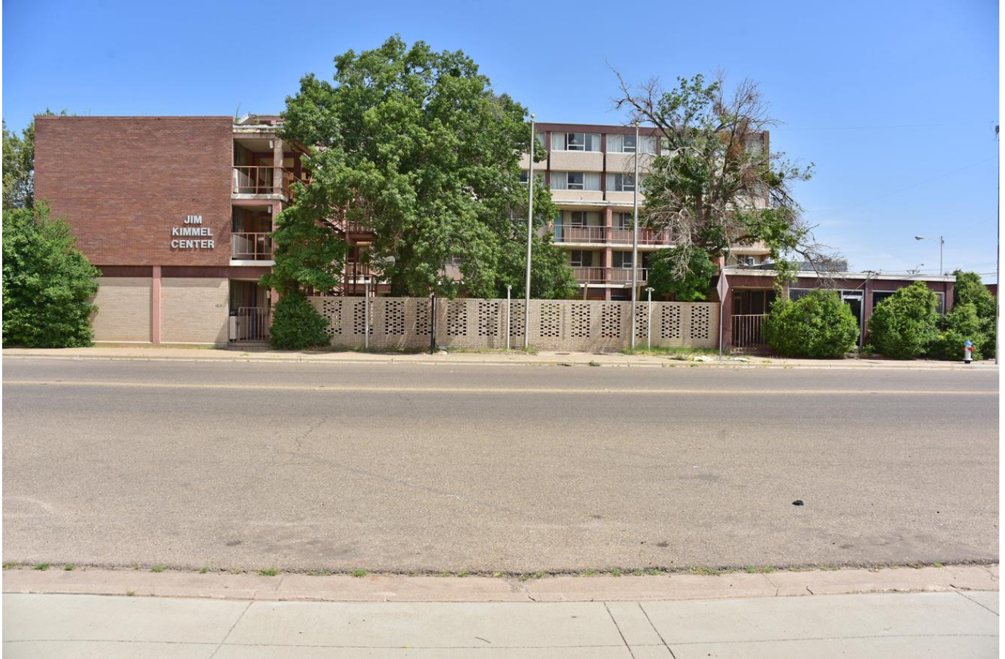
Photo 1. South elevations, view north.
