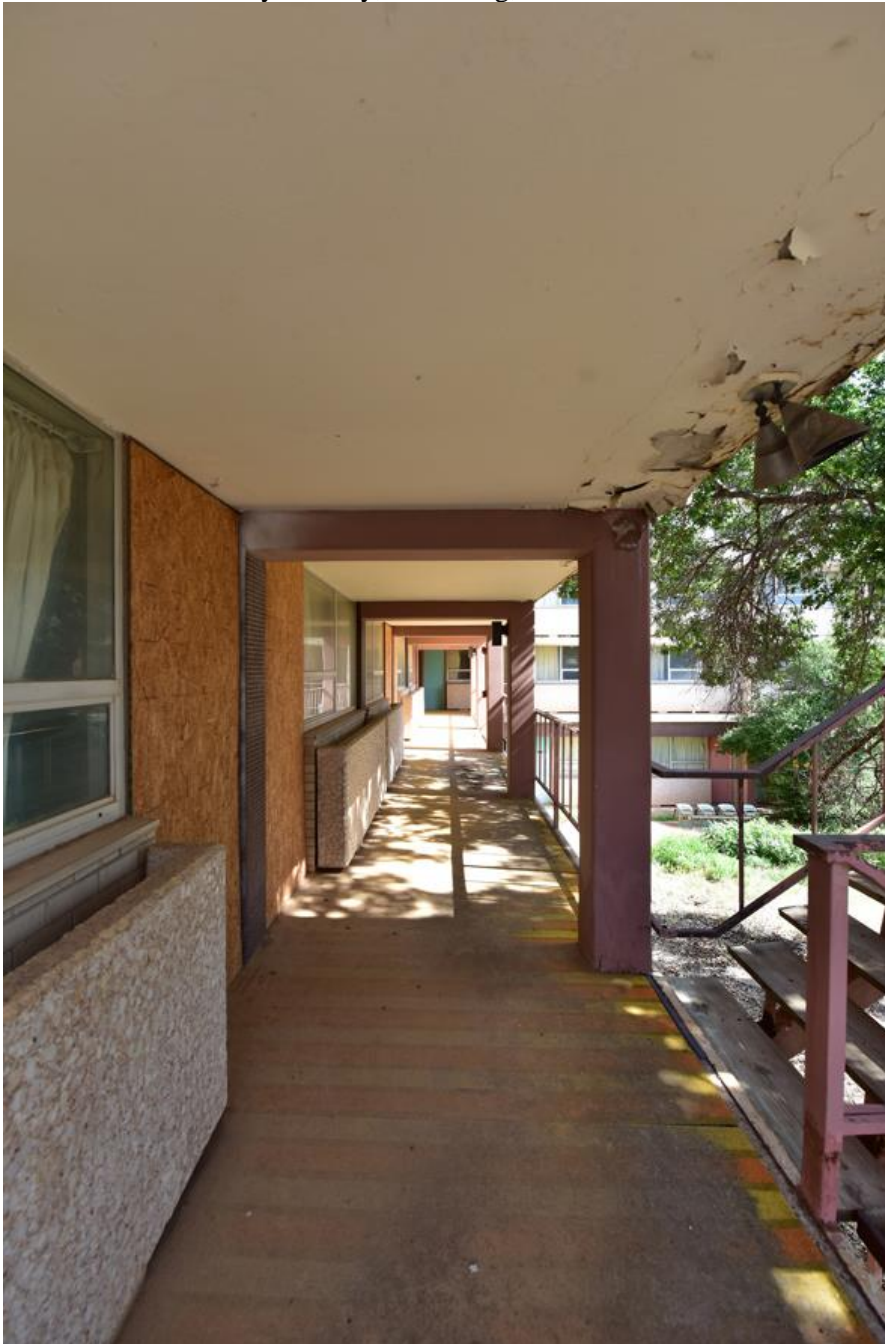
Photo 14. Second story balcony, west wing, view north.
