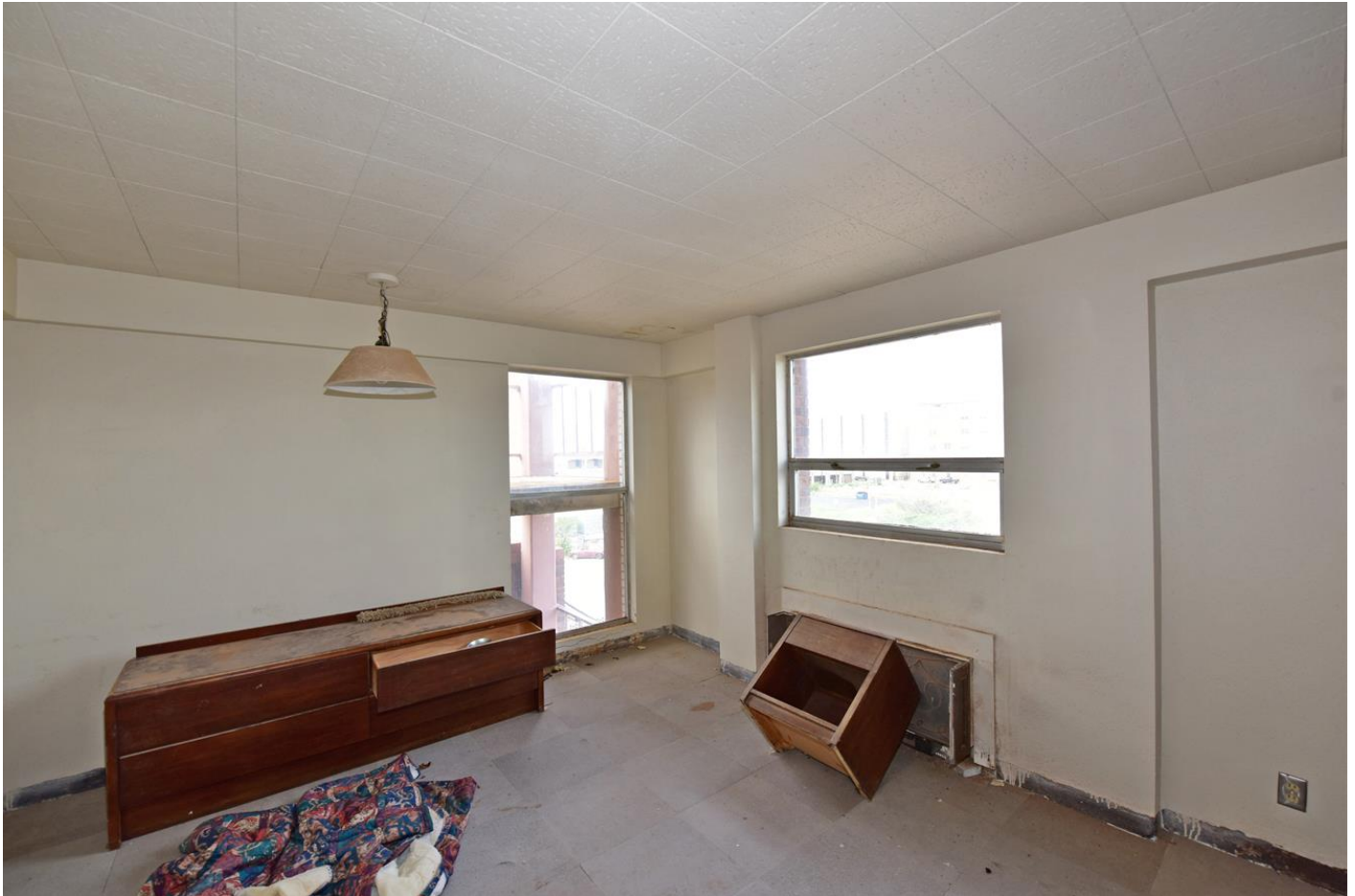
Photo 25. Fourth floor, Unit 420, view southwest.
