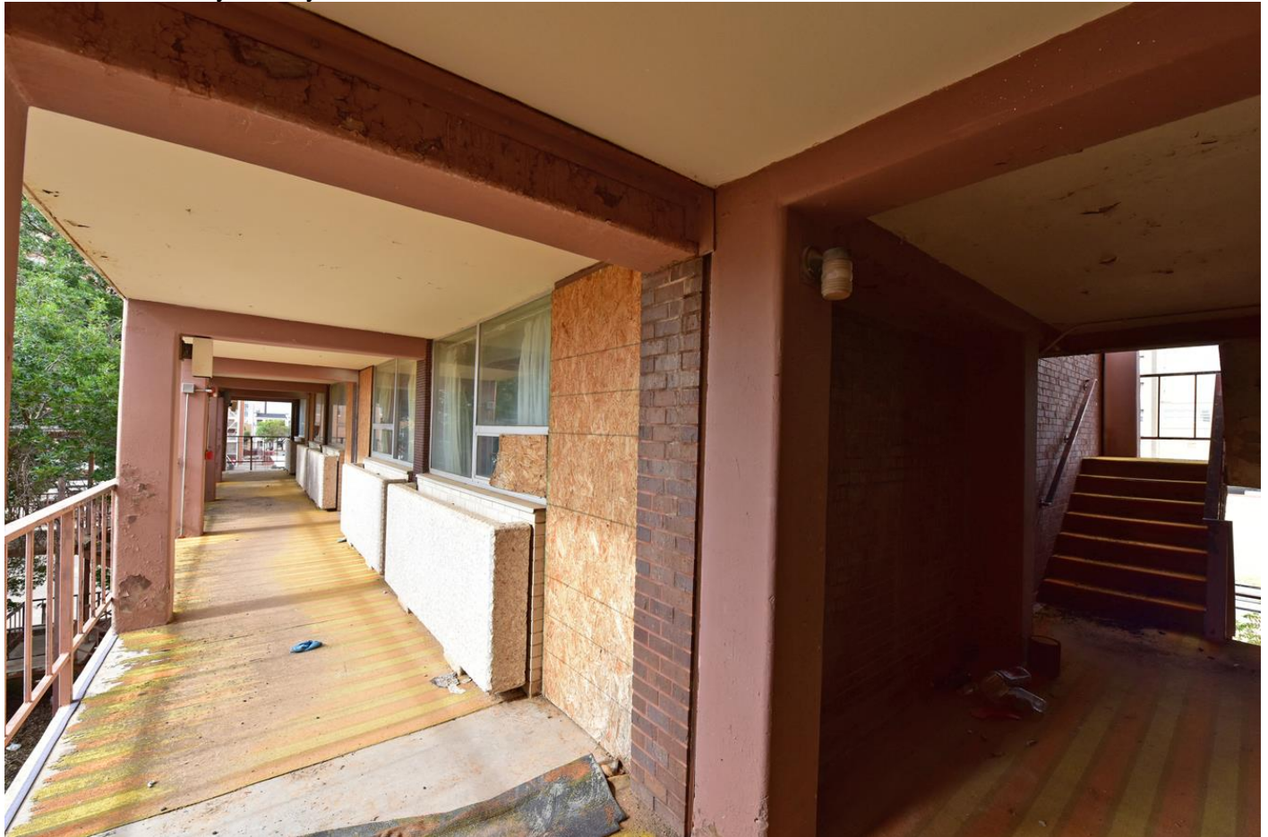
Photo 13. Third story balcony, view southwest.
