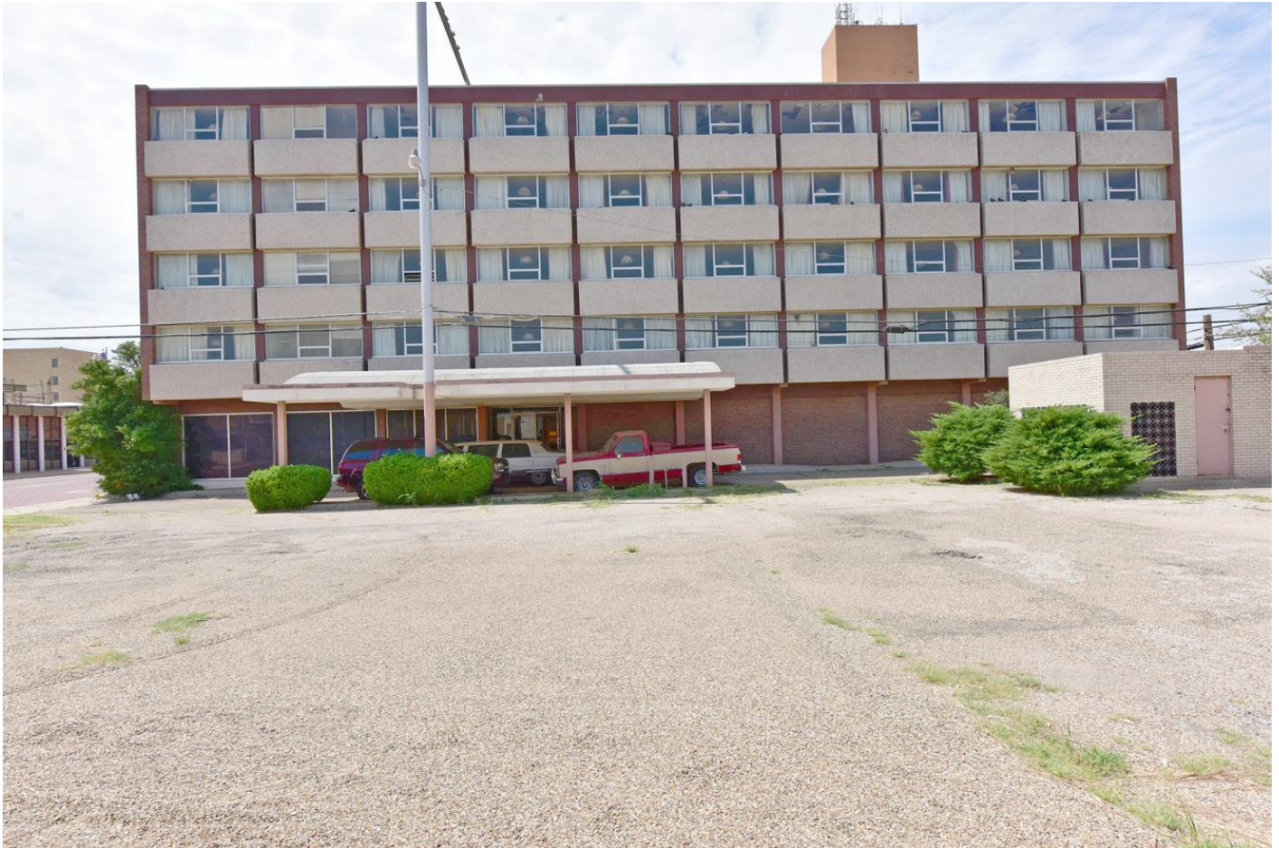
Photo 5. North elevation, view south.
