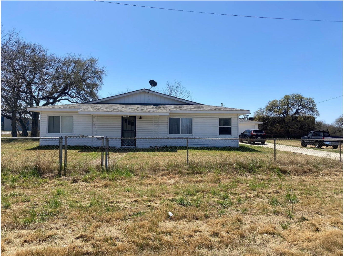
Photo 21: Primary (north) elevation of house. Camera facing south.
