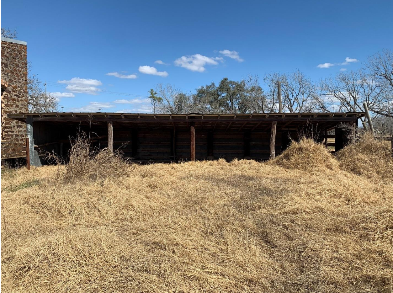
Photo 14: Southwest elevation of Shed A. Camera facing northeast.
