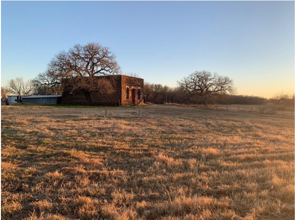
Photo 6: Primary (west) and north elevations of Heermann Store, camera facing south.
