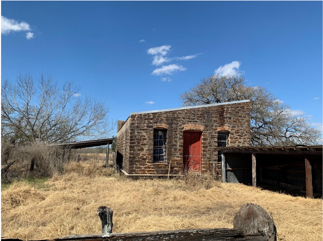
Photo 4: Rear (east) elevation of Heermann Store showing Sheds A and B, camera facing northwest.
