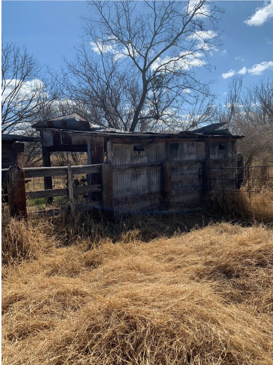
Photo 16: Northwest and northeast elevations of Shed B. Camera facing south.
