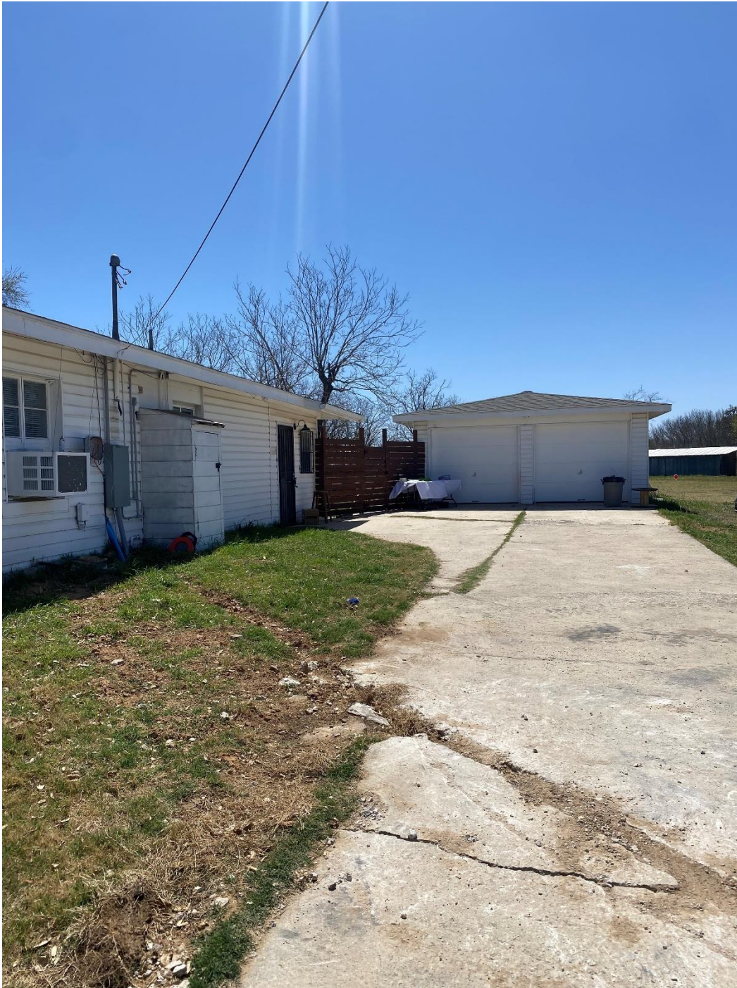
Photo 22: Primary (north) elevation of garage. Camera facing south.
