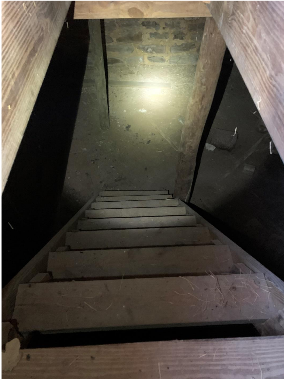
Photo 7: Heermann Store cellar.
