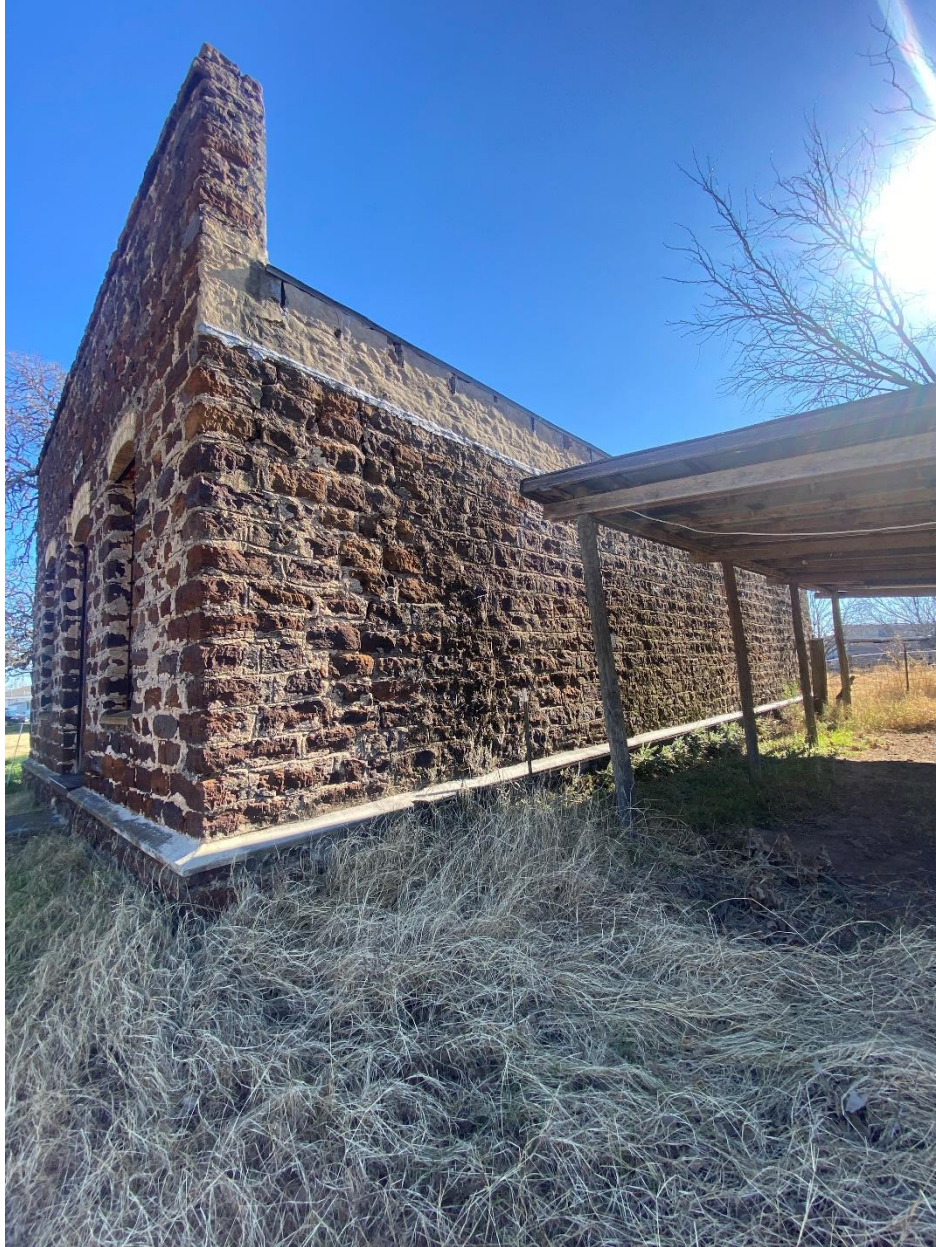
Photo 3: Primary (west) and south elevations of Heermann Store, camera facing east.
