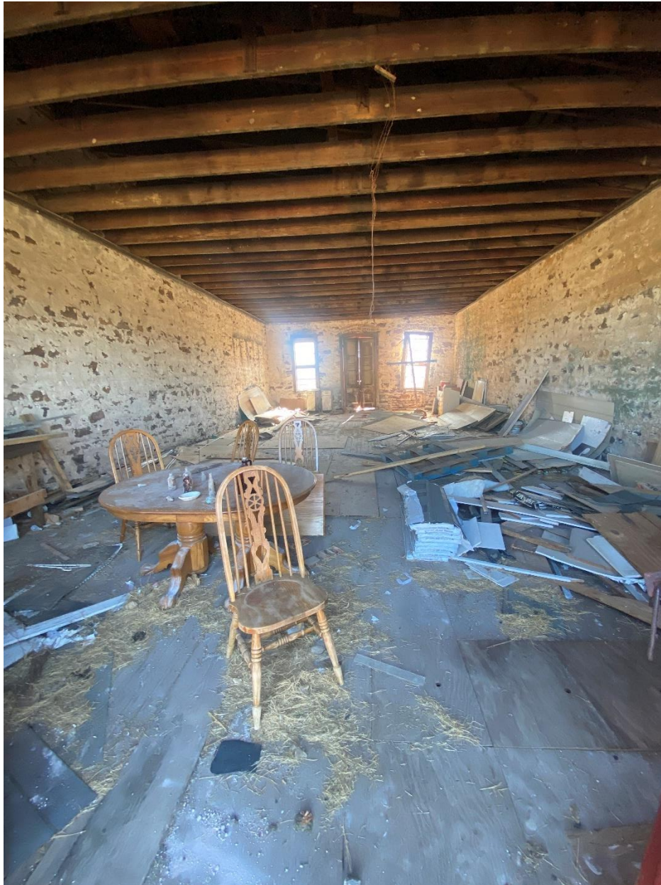
Photo 9: Heermann Store ground floor, camera facing southeast.
