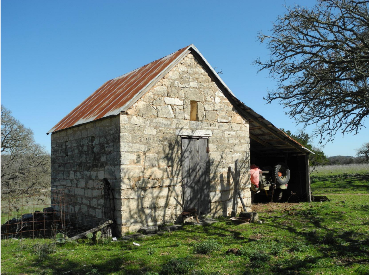
Photo 4: Contributing Building. Smokehouse (Resource 2f), limestone block and remnant with smoke vent, c. 1870, Feuge Farm. Photo by Terri Myers, March 2021, camera facing southeast.
