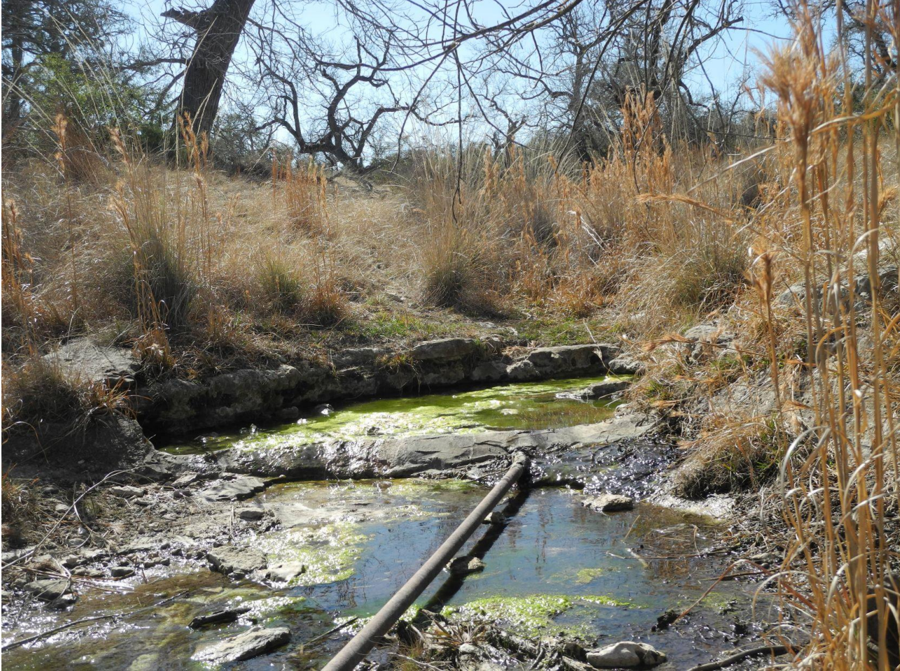
Photo 35: Contributing Structure. Developed Spring with stone-lined pools, metal pipe on Paul Stehling/Amandus Stehling pastures east of N Highway 87. Photo by Terri Myers, March 10, 2022.
