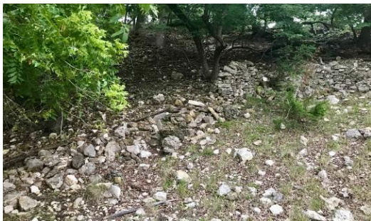
Stone Fence (12c) – This stacked limestone fence is located at the edge of some small trees near one of the ponds. The fence is two to three feet tall in sections, and has collapsed in other sections. Its total length is approximately 100 feet.
