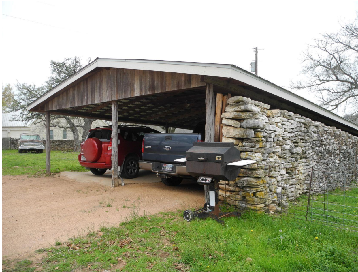
Photo 45: Noncontributing Building. Modern carport and stone wall, Amandus Stehling Farm. Photo by Terri Myers, March 25, 2021, camera facing northwest.
