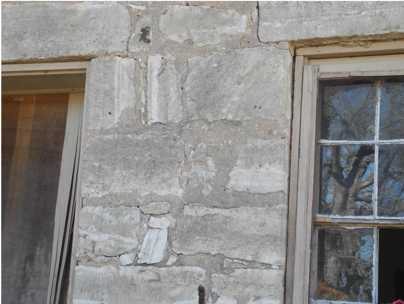
Photo 55: Materials and Methods. Stone remnants fitted to fill gaps in ad hoc fashion. Photo by Terri Myers, March 10, 2022.
