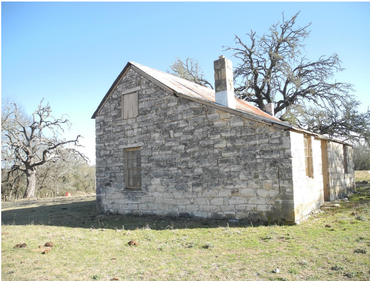
Photo 53: Materials and Methods. 1 ½ story Christoph Feuge Jr. House began as log house; c. 1870 lower logs replaced with stones, upper walls with shaped and remnant stone, chiseled corners. Shed-roofed addition of stone block/remnant. Photo by Terri Myers, March 25, 2021, camera facing southeast.
