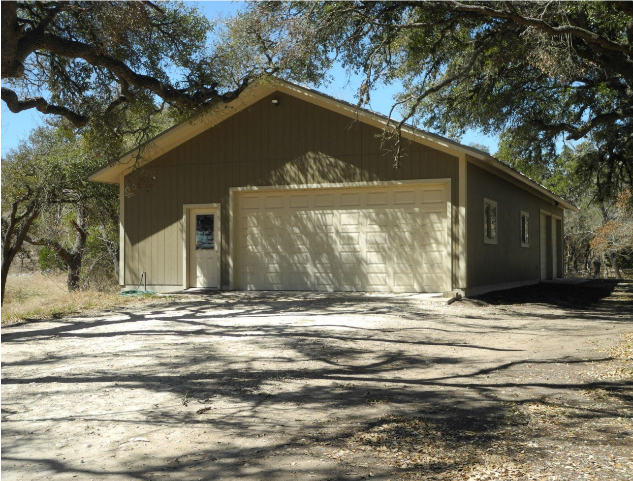
Photo 49: Noncontributing Building. Modern workshop (Resource 5b), Amandus Stehling Farm. Photo by Terri Myers, March 12, 2022, camera facing west.
