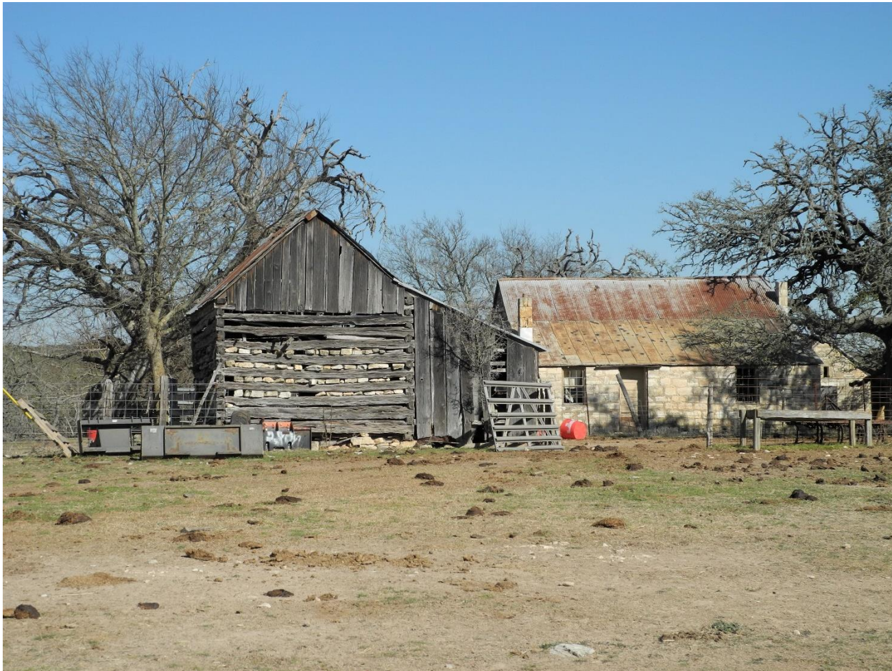
Photo 41: Contextual View. Early domestic and agricultural cluster (log barn c. 1860; limestone house c. 1870), on Feuge Farm. Photo by Terri Myers, March 10, 2022, camera facing south/southeast.
