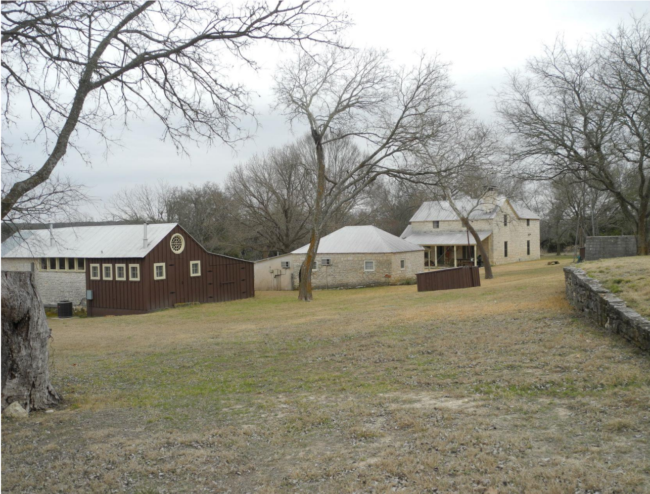
Photo 44: Contextual View. Building Cluster. Two stone barns; stone house (Resources 3c, 3b, & 3a), c. 1889, Joseph Stehling Sr./George Franz Stehling Farm. Photo by Terri Myers, March 11, 2022, camera facing west.
