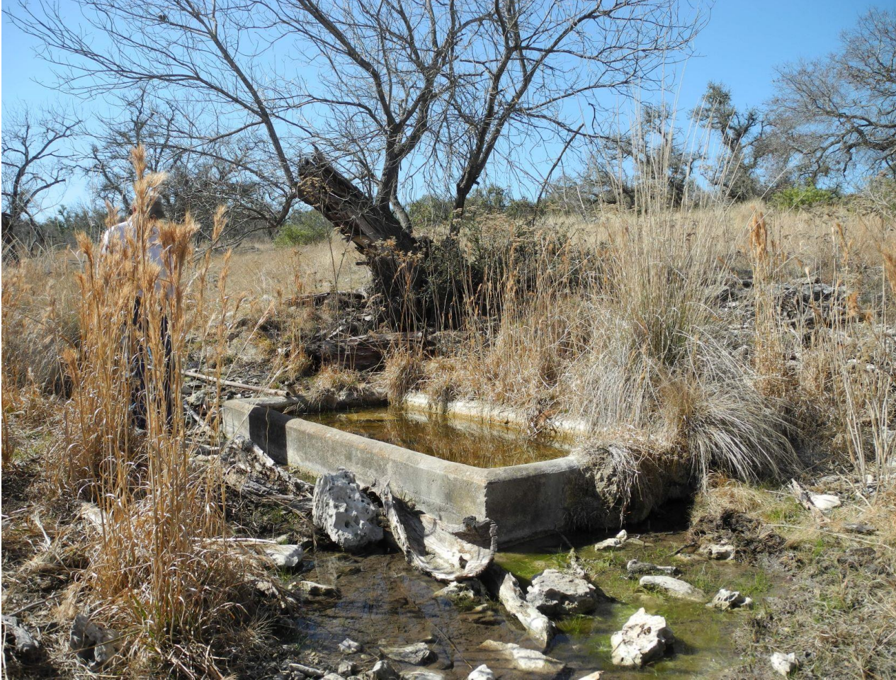
Photo 36: Livestock Trough concrete basin; water piped from developed spring, 1930s, Paul Stehling/Amandus Stehling pasture east of N Highway 87. Photo by Terri Myers, March 10, 2022.
