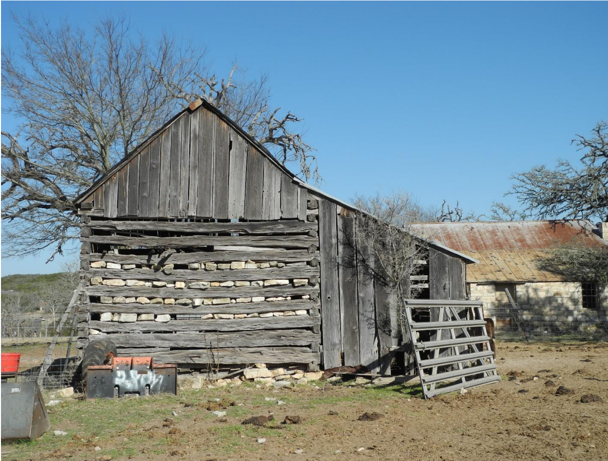
Photo 52: Materials and Methods. V-notched rough-hewn logs chinked with stones, c. 1860; type associated with German immigrant settlers in Texas Hill Country. Photo by Terri Myers, March 10, 2022, camera facing north.
