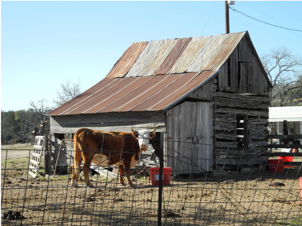
Photo 5: Log Barn (Resource 2d), V-notch timbers, c. 1860; frame shed addition c. 1900, Feuge Farm. Photo by Terri Myers, March 10, 2022, camera facing northwest.
