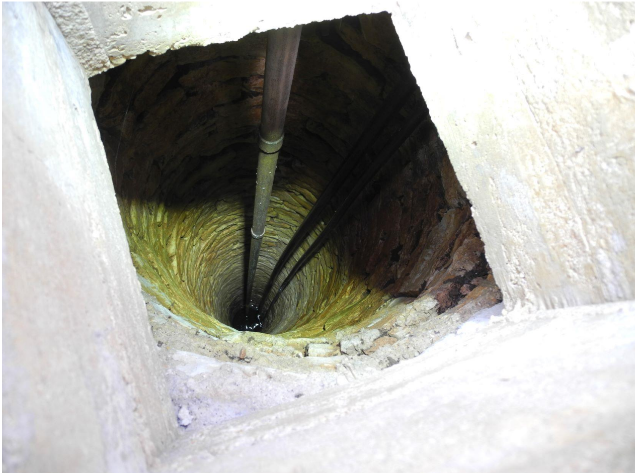
Photo 21:Contributing Structure. Hand-dug, stone-lined Well (Resource 6d), c. 1860, Amandus Stehling Farm. Photo by Terri Myers, March 2021.
