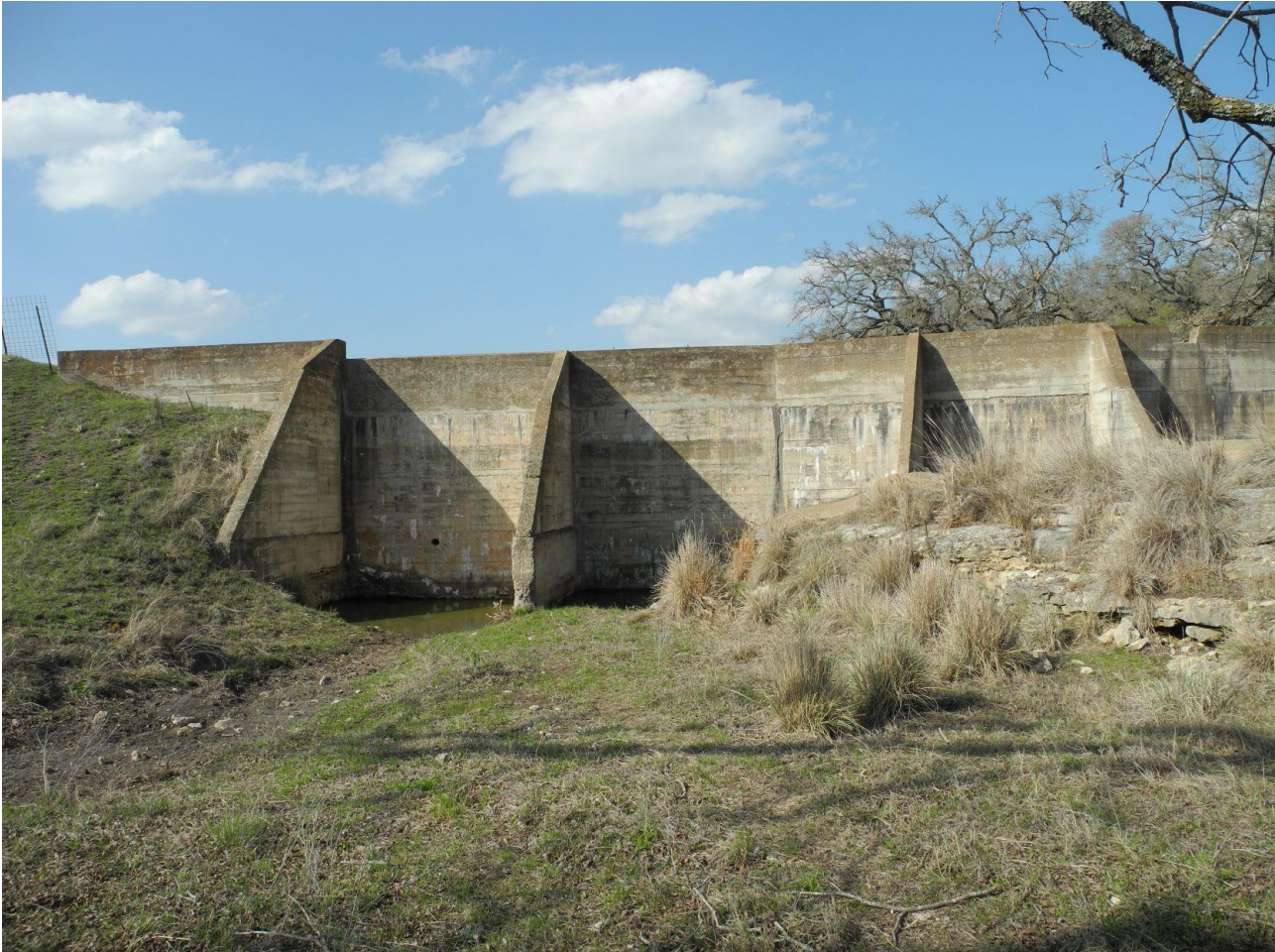
Photo 32: Contributing Structure. Concrete Dam (Resource 10a), c. 1937, hand-mixed and poured by Stehling brothers east of N Highway 87. Photo by Terri Myers, March 25, 2021, camera facing east.
