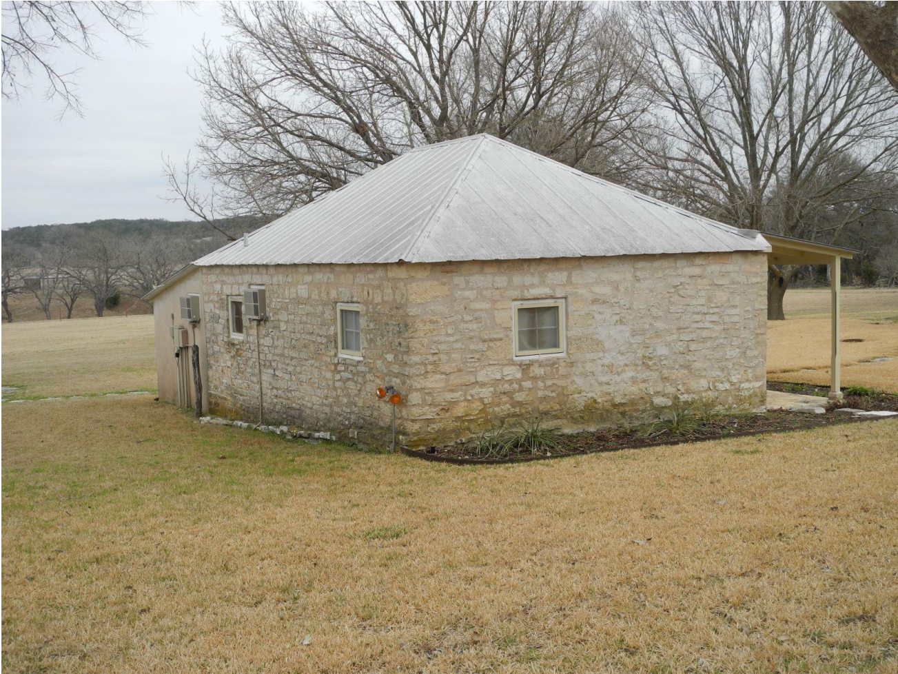
Photo 16: Contributing Building. Stone Barn converted to guest house (Resource 3b), c. 1890, on George Franz Stehling Farm. Photo by Terri Myers, March 11, 2022, camera facing southwest.
