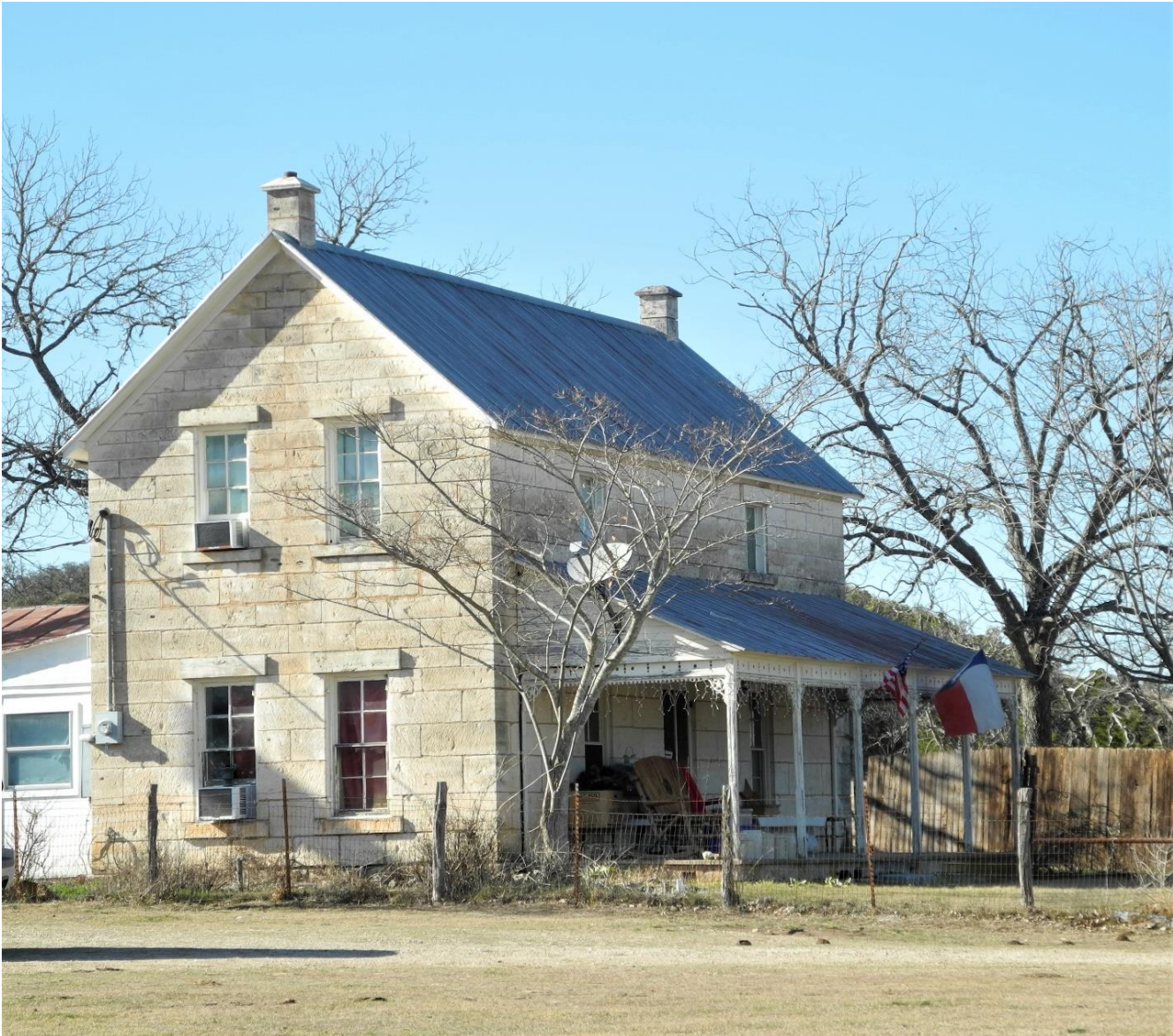
Photo 1: Contributing Building. Carl Feuge House, aka “1901 House,” (Resource 2a), quarried limestone house with Folk Victorian porch posts and trim. Photo by Terri Myers, March 10, 2022, camera facing northwest.
