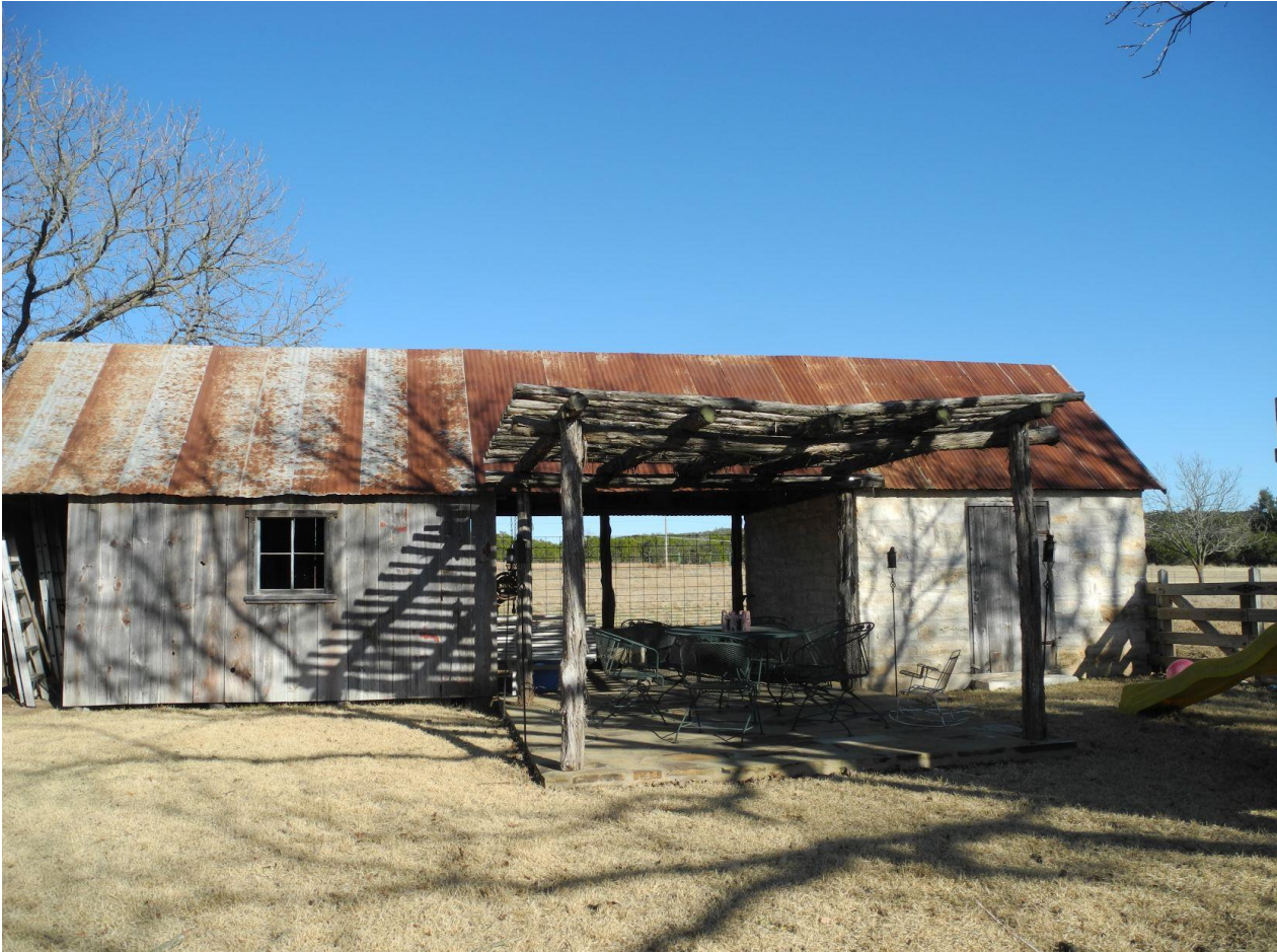
Photo 22: Contributing Building. "Dogtrot" Kitchen/Blacksmith Shop/Wash House (Resource 6c), c. 1881, Amandus Stehling Farm. Photo by Terri Myers, March 12, 2022, camera facing east.
