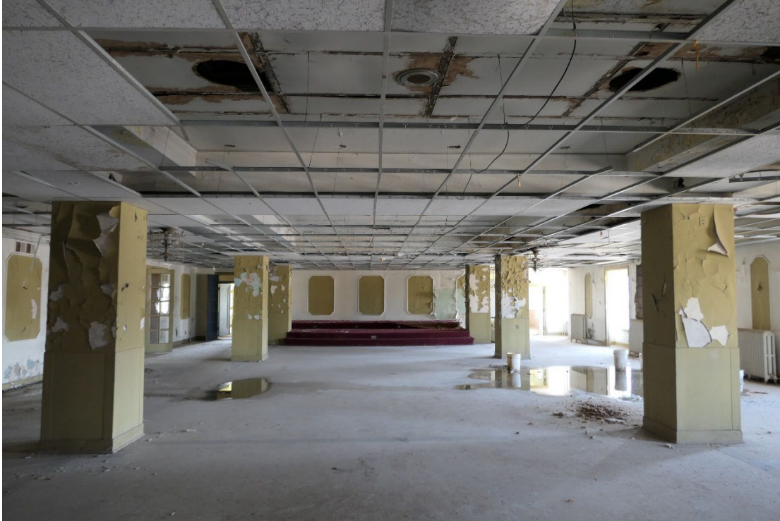
Photo 22: Second floor/mezzanine ballroom, looking east.
