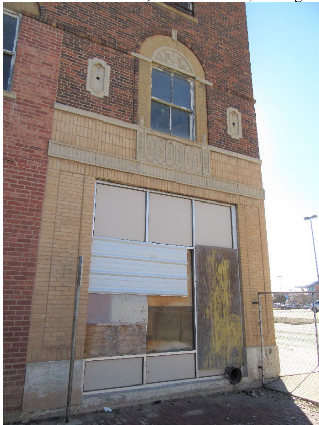
Photo 8: West elevation, south storefront, looking southeast.
