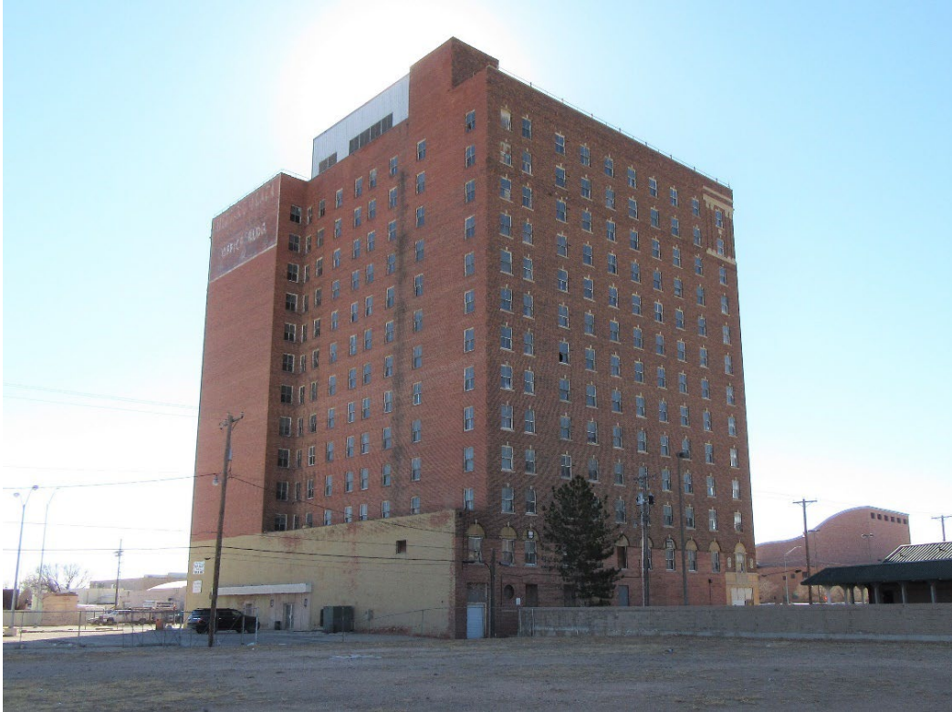
Photo 6: North and west elevations, looking southeast.
