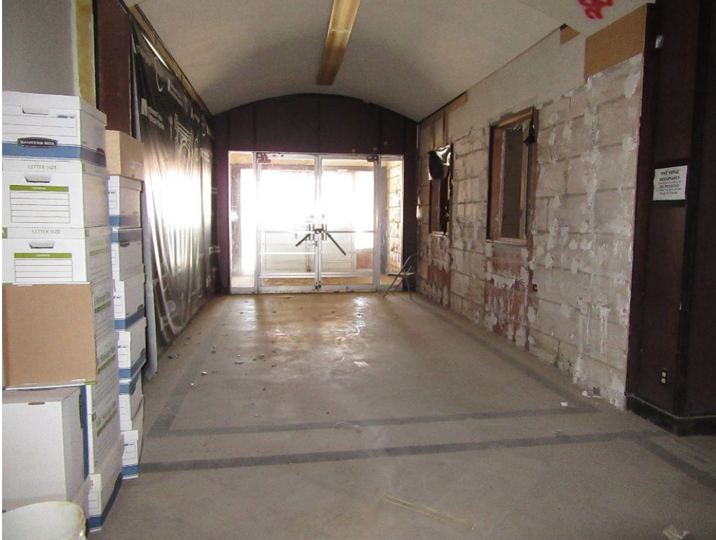
Photo 14: First floor, main (south) entrance, looking south.
