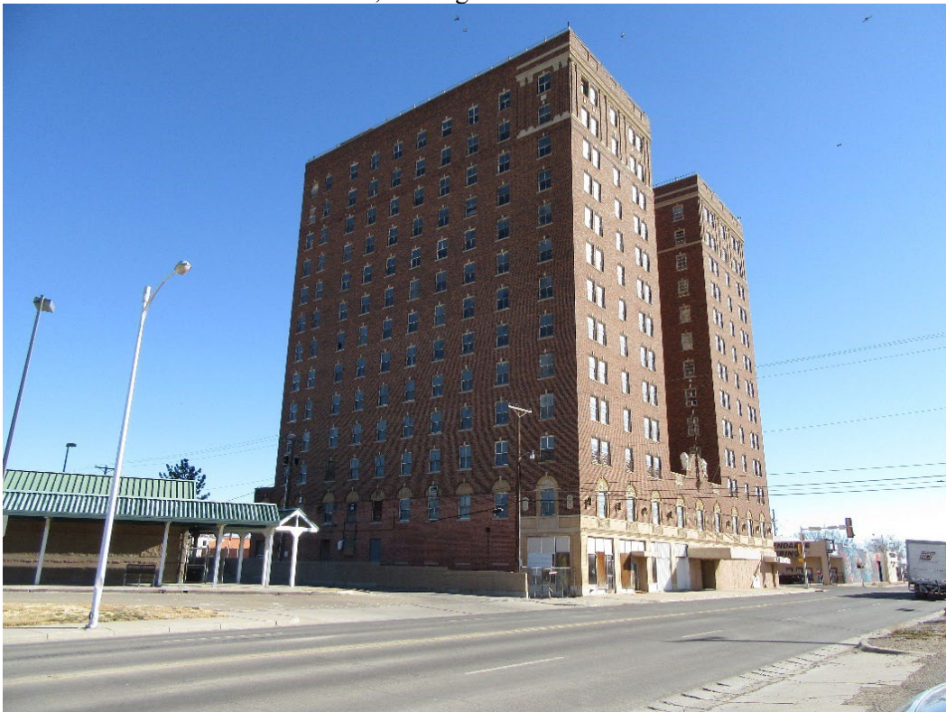
Photo 7: South and west elevations, looking northeast.
