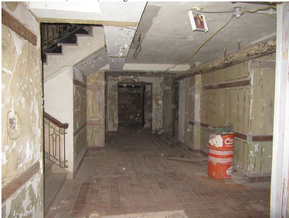
Photo 9: Basement, corridor, looking east.
