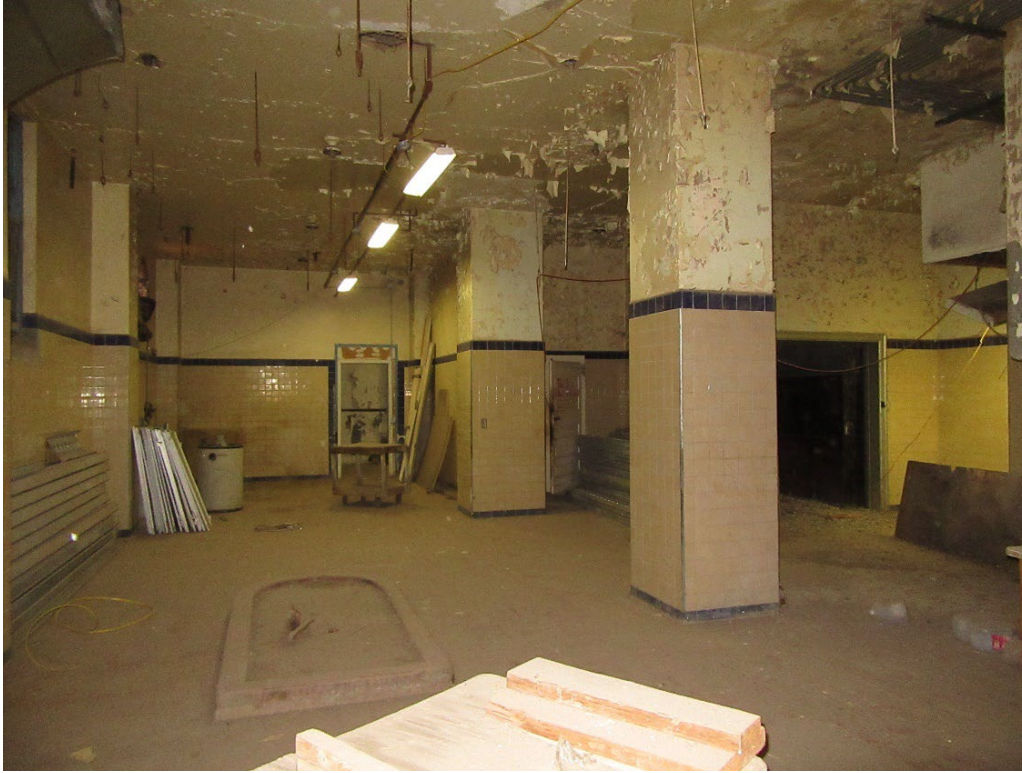
Photo 18: First floor, kitchen, looking north.
