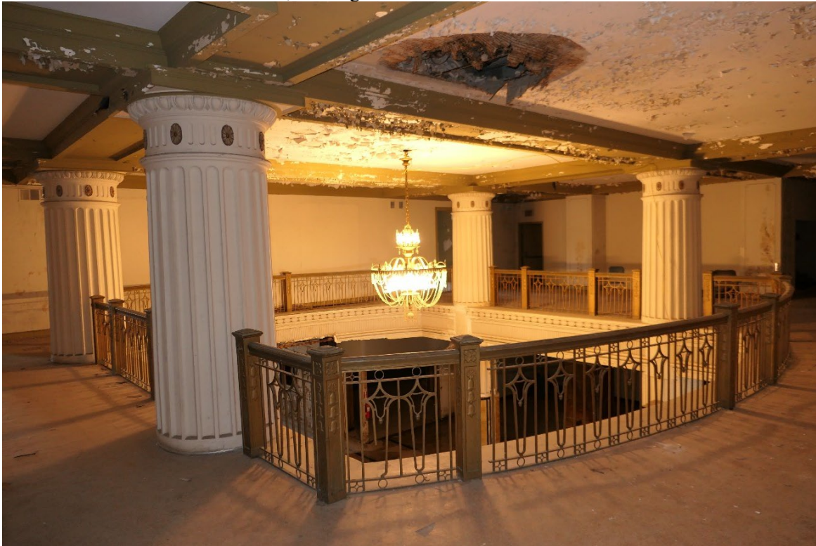
Photo 20: Second floor/mezzanine, looking northwest.
