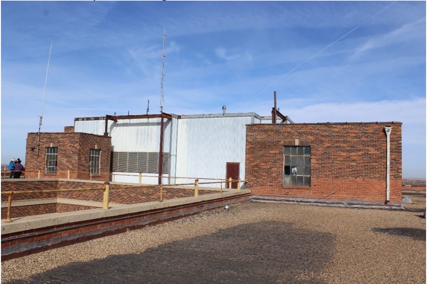
Photo 32: Main roof and penthouses, looking northwest.
