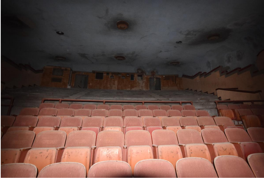
Photo 13. Interior, from front to rear of mezzanine, view facing east.
