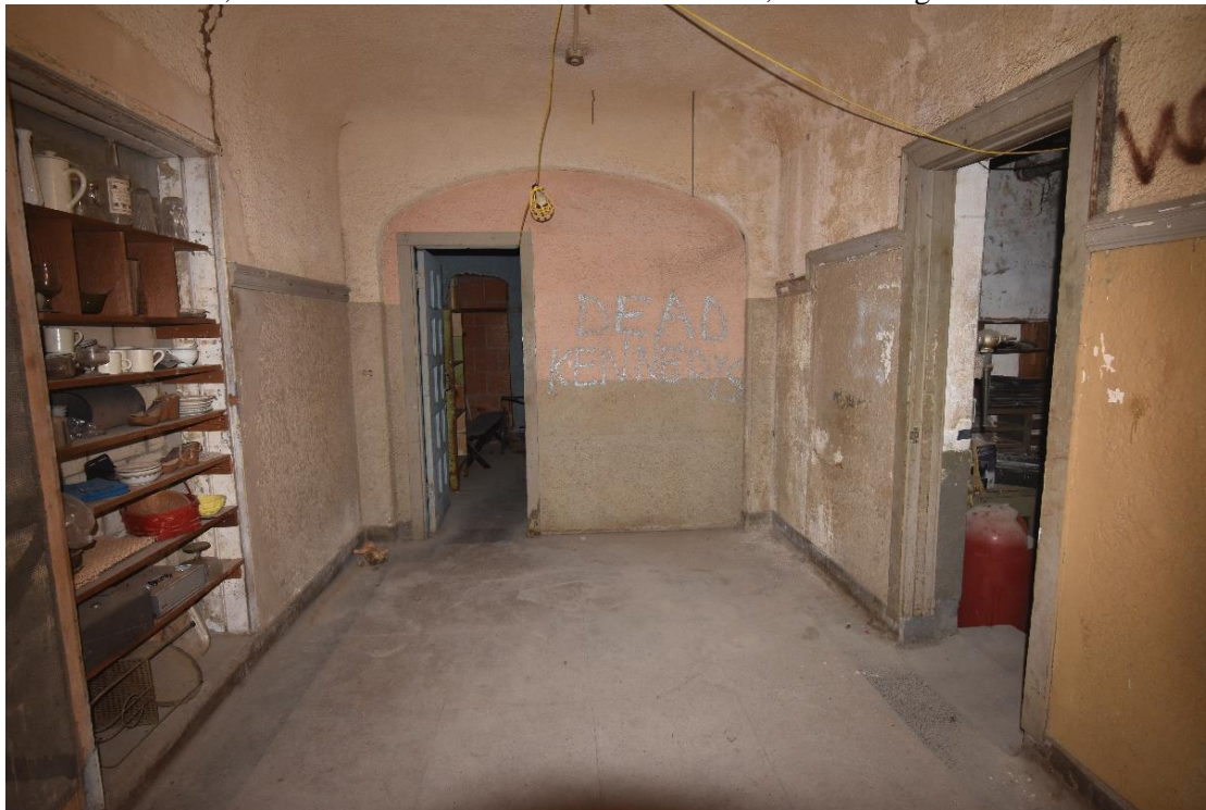
Photo 19. Interior, enclosed arched wall and built-in shelves, view facing west.
