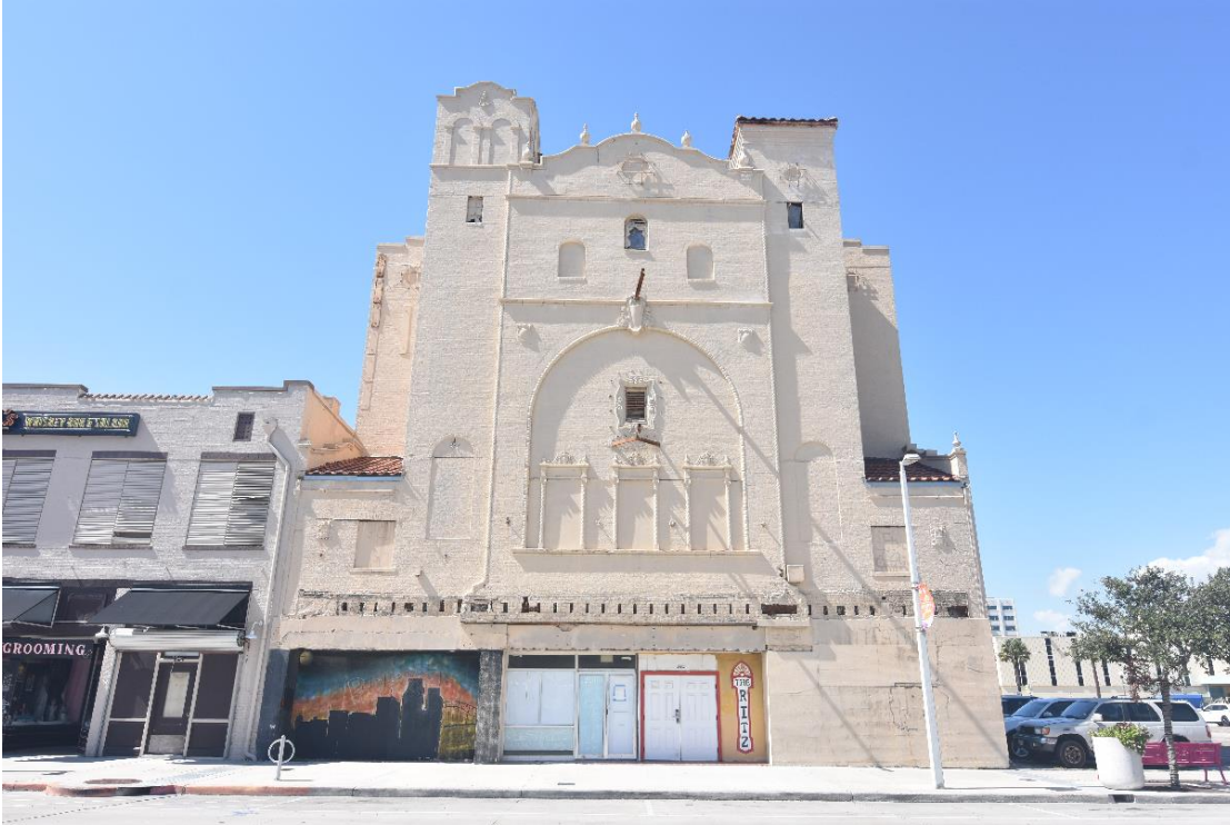
Photo 1. Front façade, view facing west.
