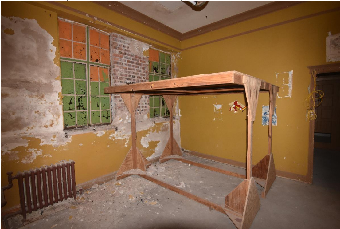
Photo 14. Interior, second floor office, view facing southeast.
