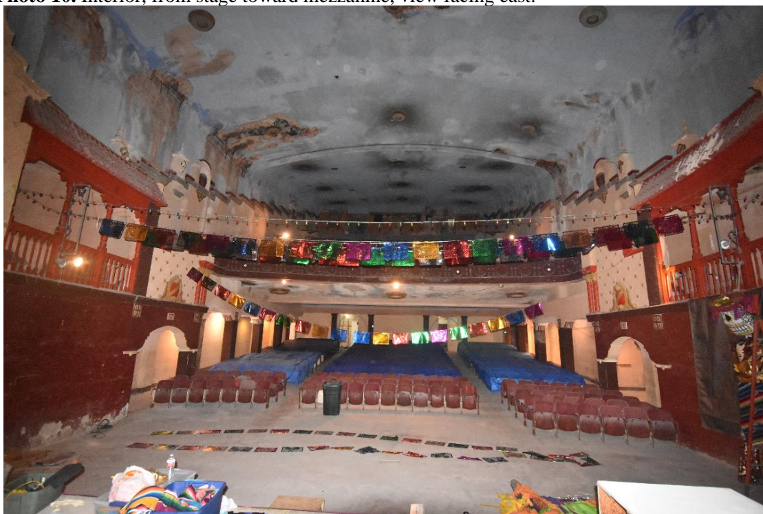
Photo 10. Interior, from stage toward mezzanine, view facing east.
