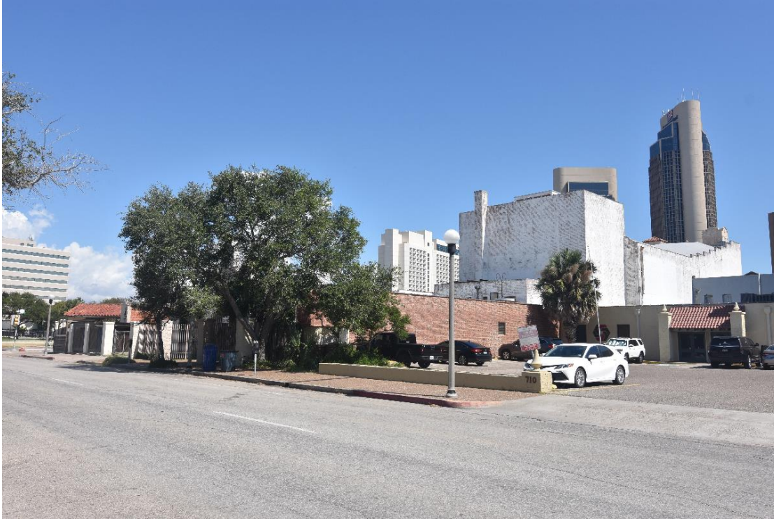
Photo 5. South façade, central lower portion obstructed by adjacent building, and west façade of the theater stage, view facing northeast.
