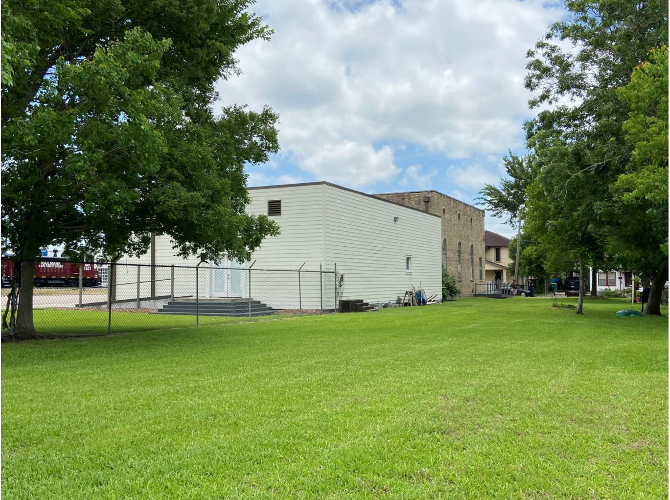
Photo 4. Oblique of north and west façades of community house (foreground) and synagogue (background). Camera facing southeast.
