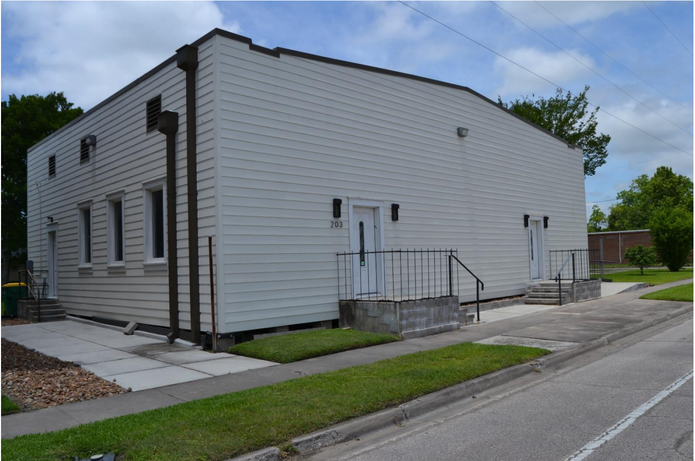
Photo 16. Oblique view of south and east façades of community house. Camera facing northwest.
