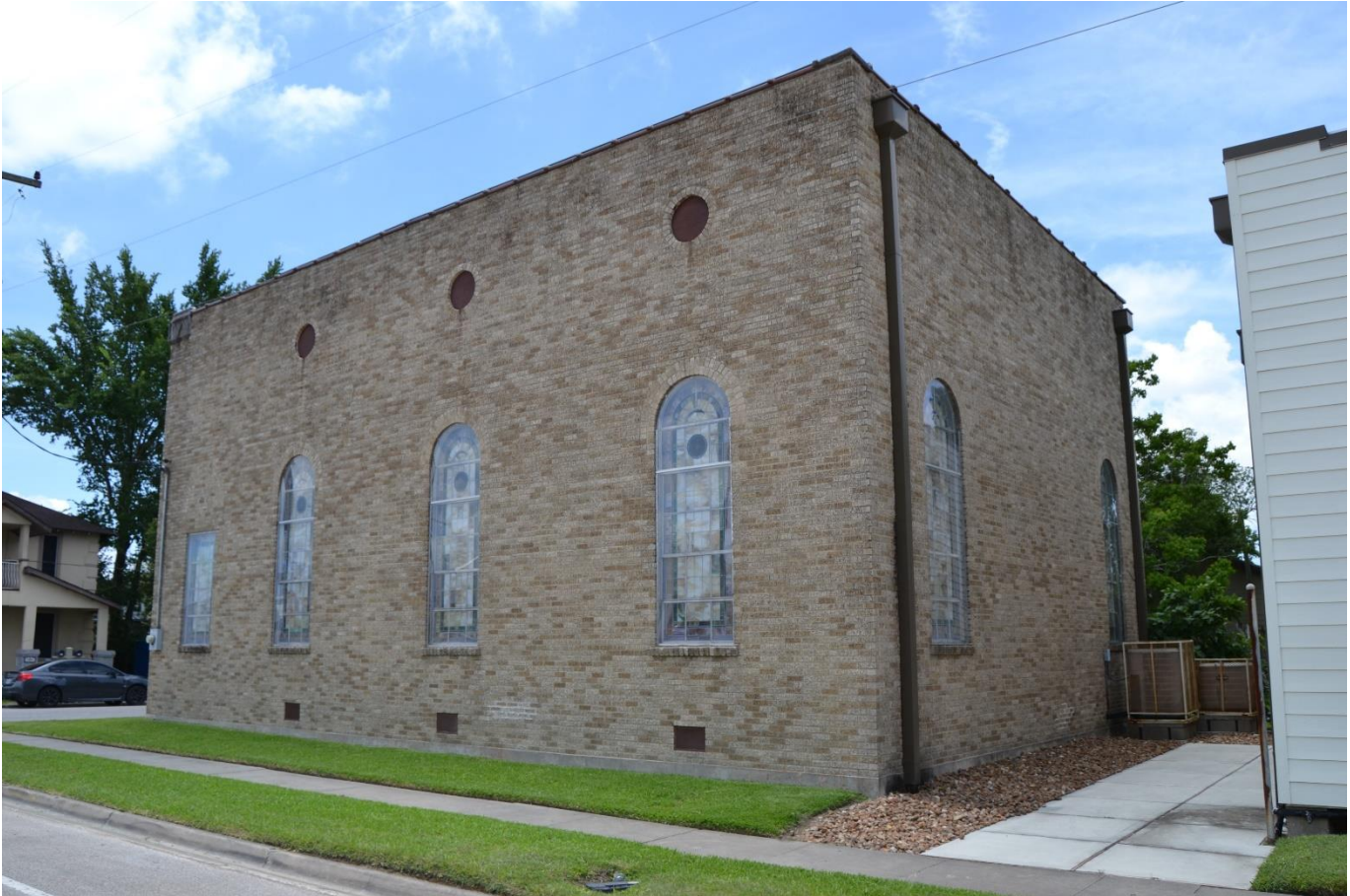
Photo 6. Oblique of east and north façades. Camera facing southwest.
