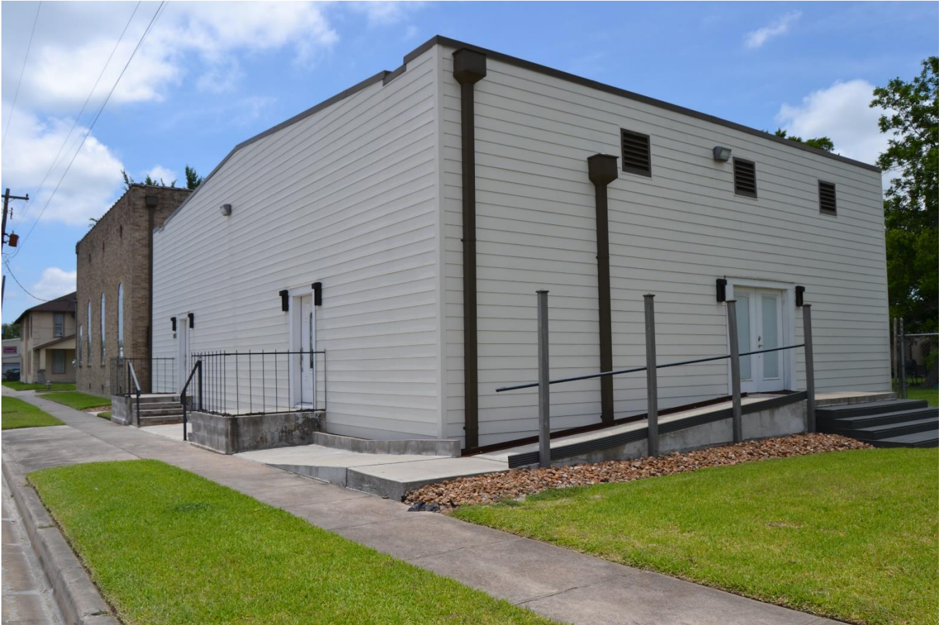
Photo 17. Oblique view of north and east façades of community house. Camera facing southwest.
