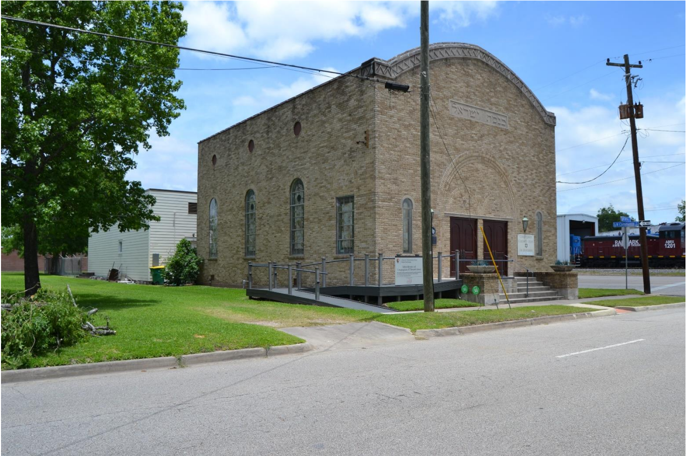
Photo 2. Oblique of west and south façades with railroad right-of-way to the east. Camera facing northeast.
