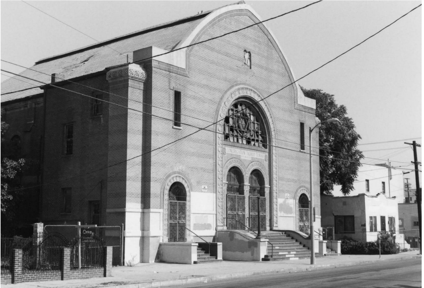
Figure 24. Congregation Talmud Torah of Los Angeles (Breed Street Shul). View from the Southeast, 2001. National Register of Historic Places form. Source: National Archives Catalog. https://catalog.archives.gov/id/123859047 .
