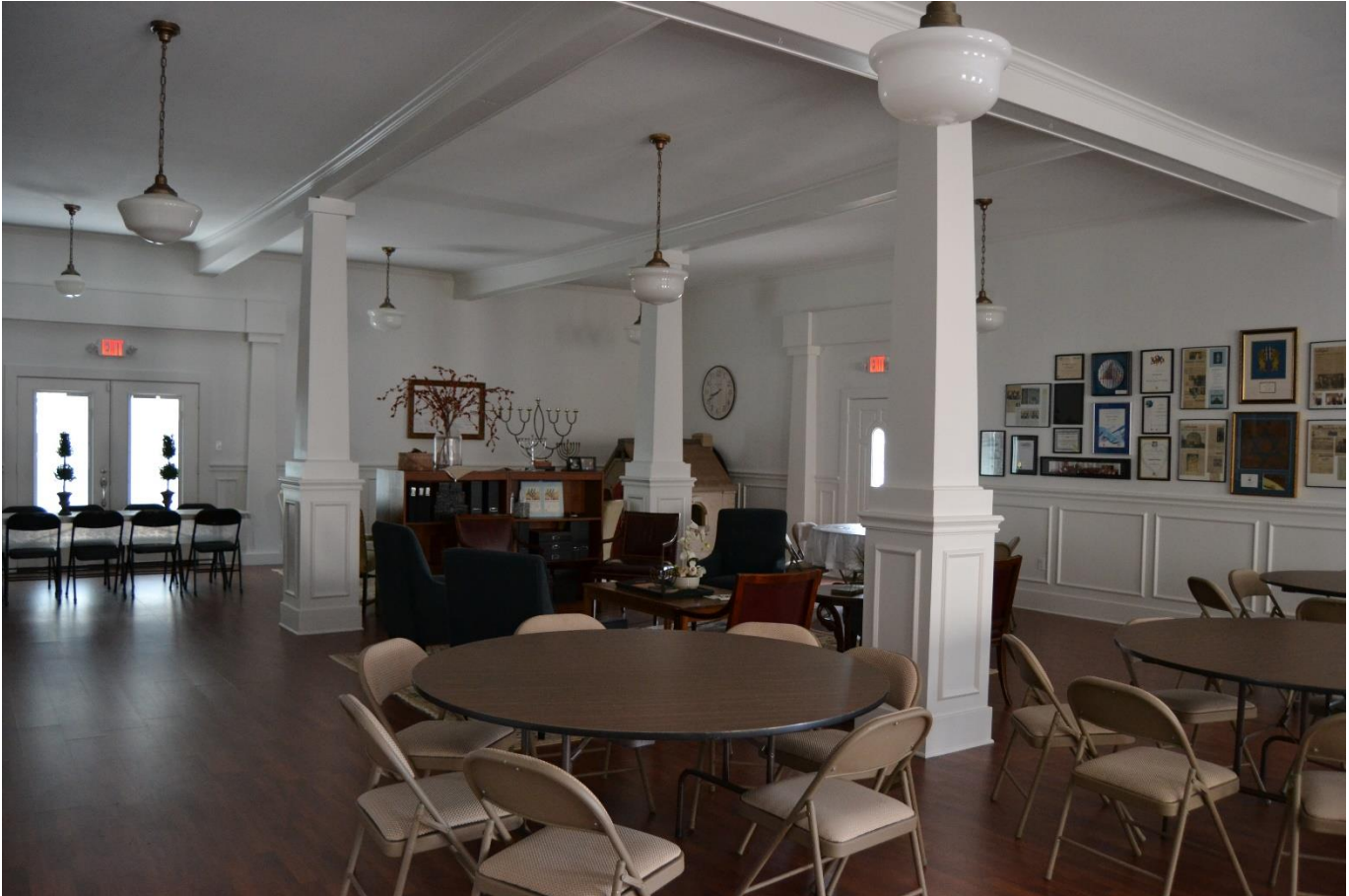
Photo 20. Interior view of community house showing the free-standing columns in the 1948 addition and other classically inspired wood trim. Camera facing northeast.
