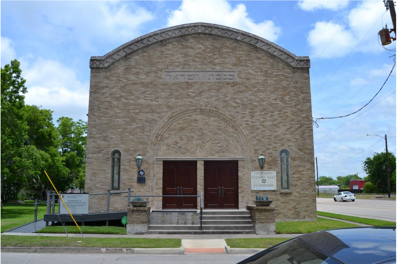
Photo 5. Front (south) façade of synagogue. Camera facing north.
