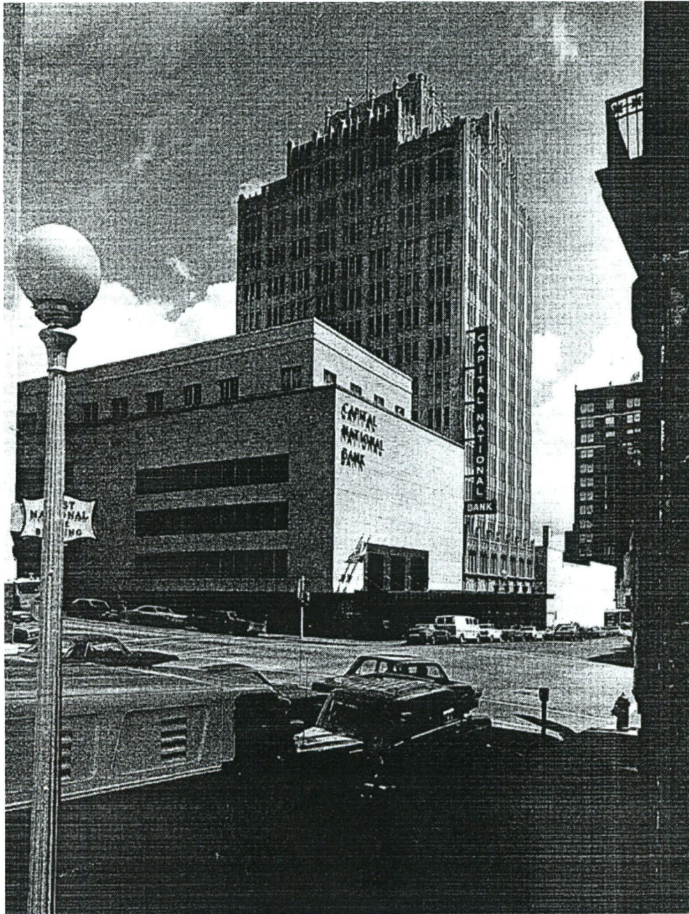
Figure 12. Capital National Bank alterations to Motoramp Garage, ca. 1951.
