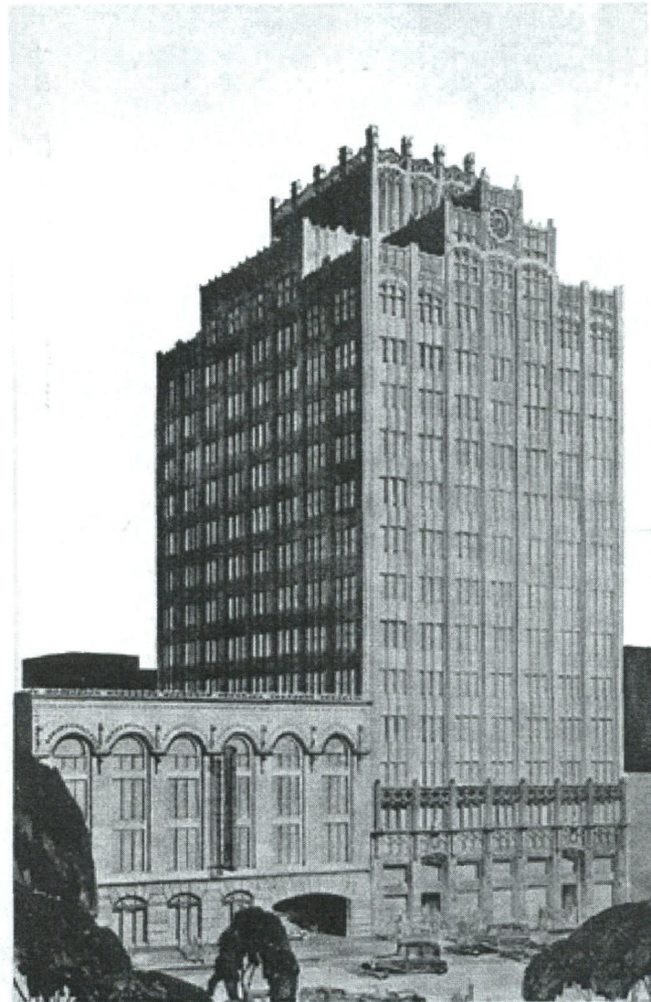
1206 THE NORWOOD BUILDING, AUSTIN, TEXAS (GIESECKE & HARRIS, ARCHITECTS)
