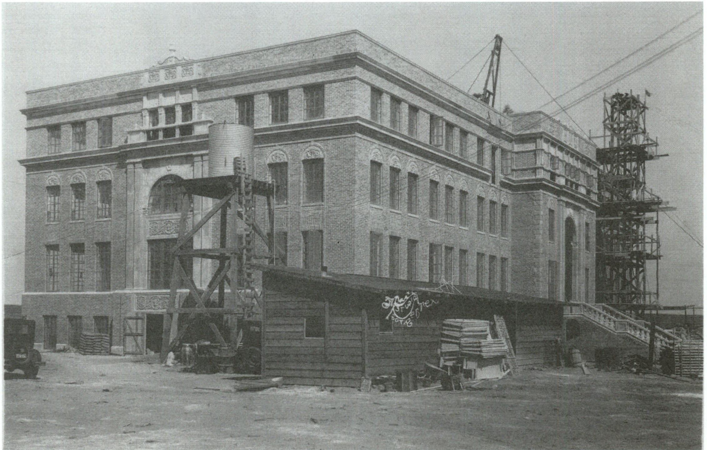
Figure 7: Hutchinson County Courthouse under construction in 1928. Photo courtesy of the Hutchinson County Historical Museum, Borger, Texas.
