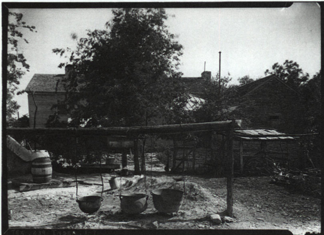
Figure 8: View of the rear yard of the main house, 1936. Historic American Buildings Survey, Harry L. Starnes, Photographer, April 23, 1936. REAR ELEVATION. HABS TEX,239-INDEP,1-7.
