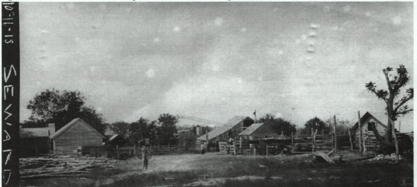
Figure 11: View of the service complex from the east, looking west, c. 1915.
