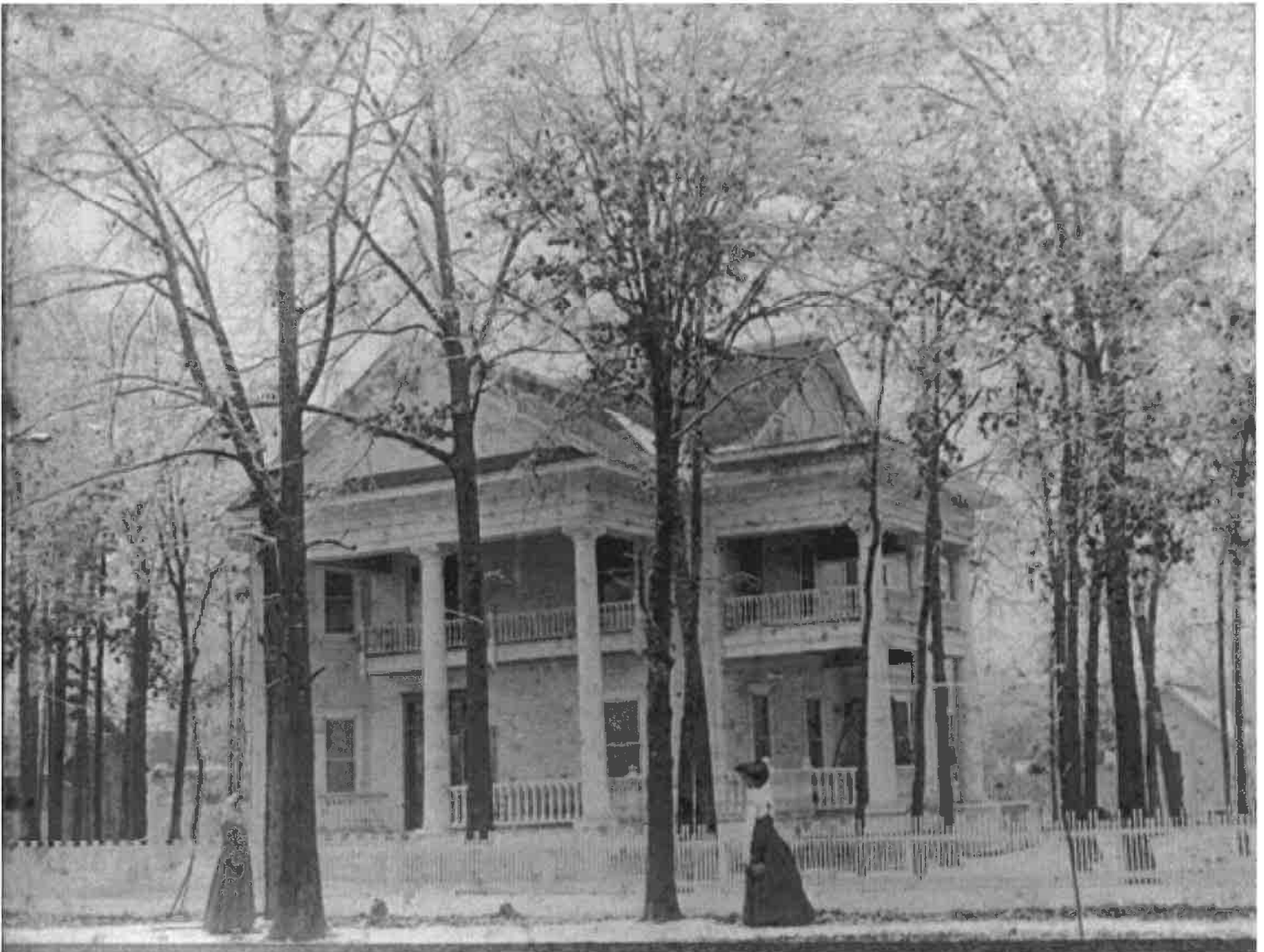
Figure 1: Historic Photo, c. 1903. West (left) and south (right) elevations.
