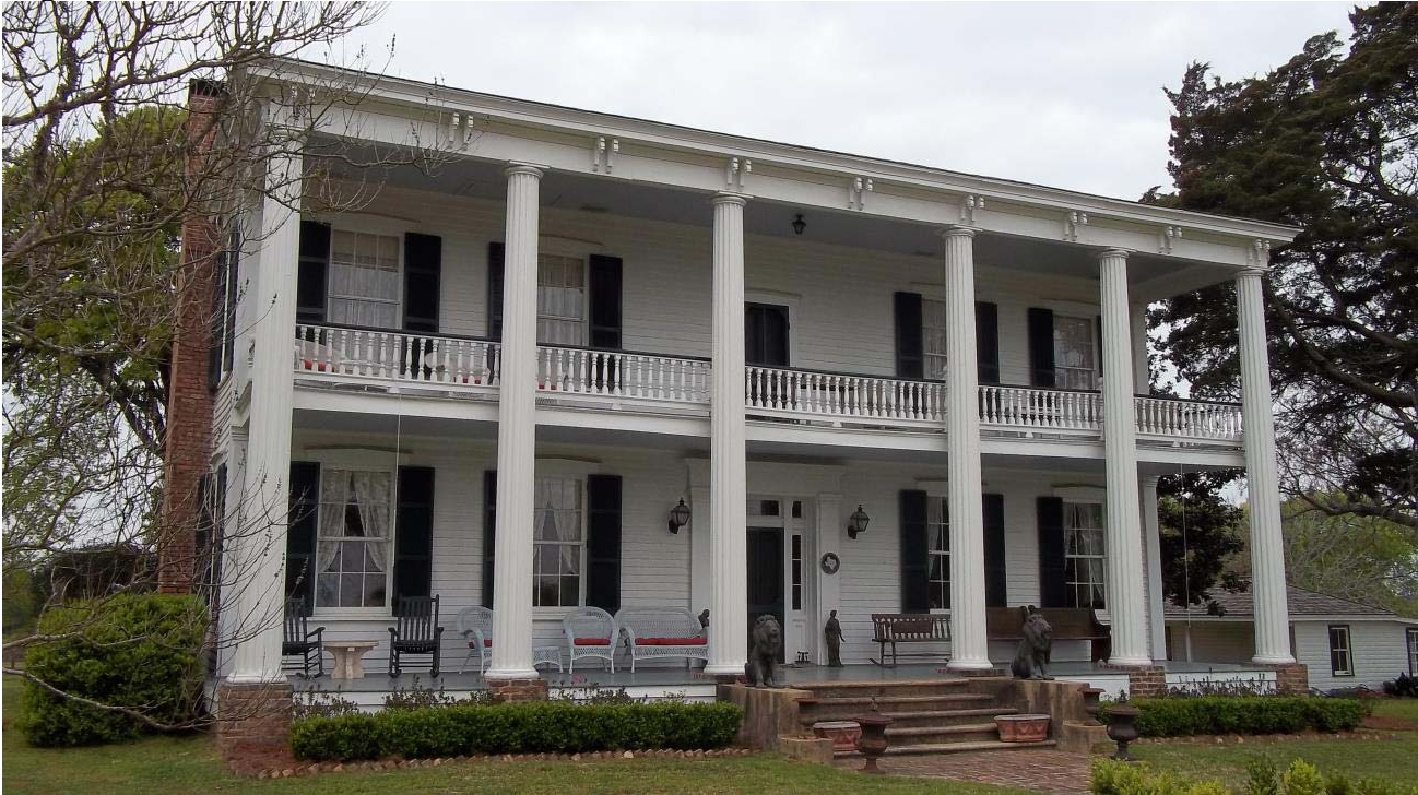
Figure 1: Southeast elevation of Monte Verdi Plantation House, current.
