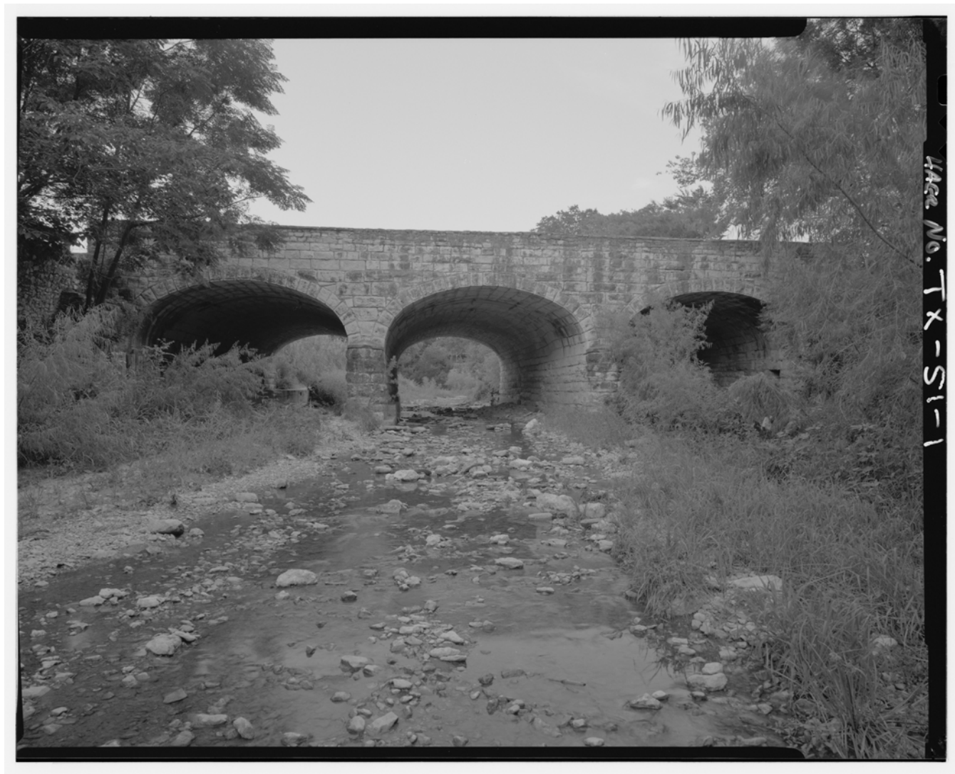
1996 HAER Photo 1 Elevation from south
