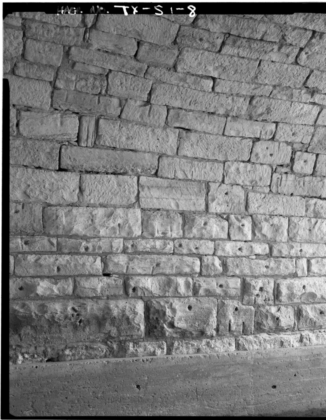
1996 HAER Photo 8 Underside of central arch, looking northwest
