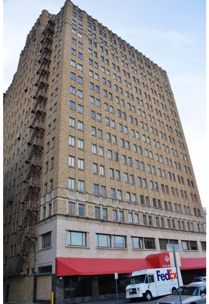
TX_Bexar County_Milam Building_0003.tif west elevation looking southeast
