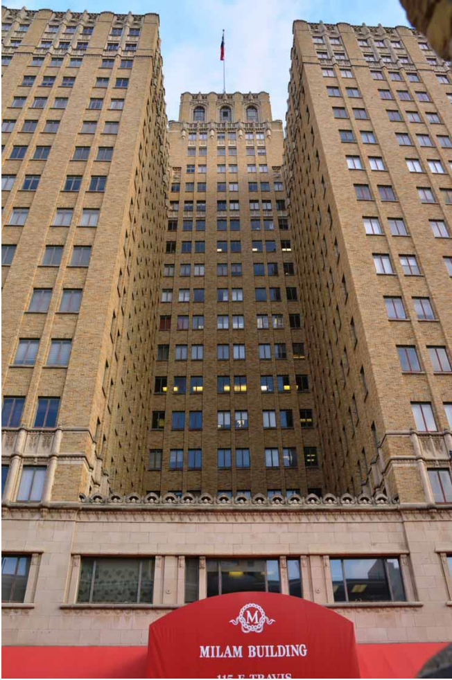
TX_Bexar County_Milam Building_0002.tif south elevation looking north
