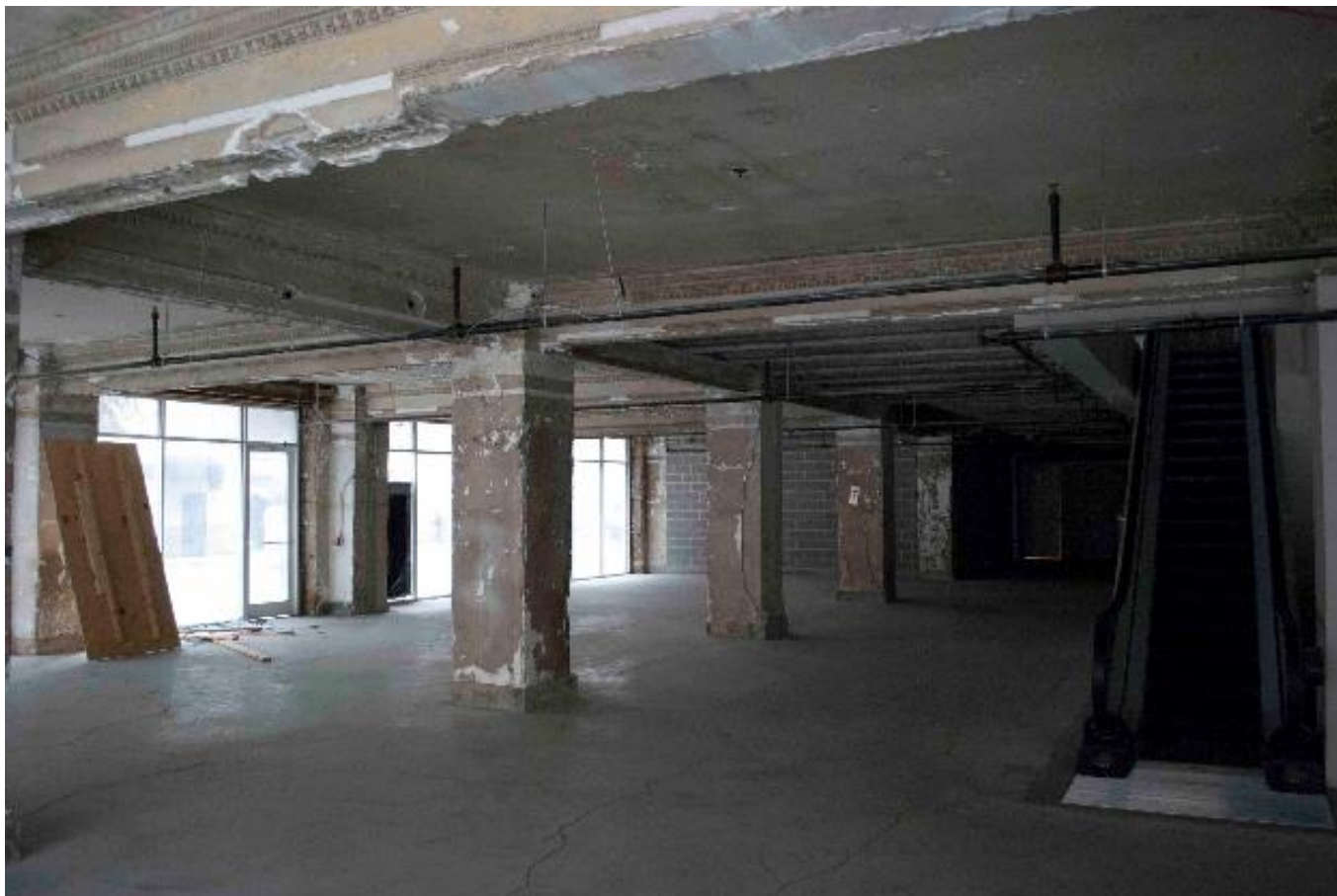
Photo #6 Interior, tenth floor, camera facing south, 2014.
