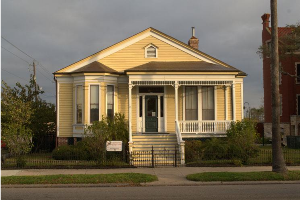
Photo 1: South elevation; camera facing north
