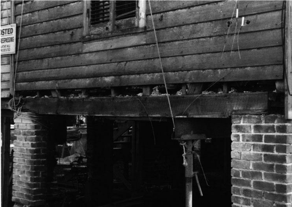
Figure 12: East elevation of rear addition breezeway of Quigg-Baulard Cottage; depicts pier and beam foundation and remains of exterior shutters and half wall; roof protected by tarps. Camera facing west.
