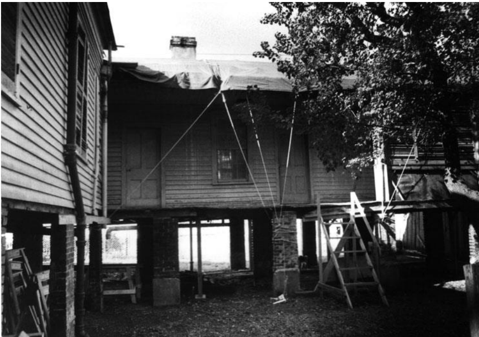
Figure 12: East elevation of rear addition breezeway of Quigg-Baulard Cottage; depicts pier and beam foundation and remains of exterior shutters and half wall; roof protected by tarps. Camera facing west.
