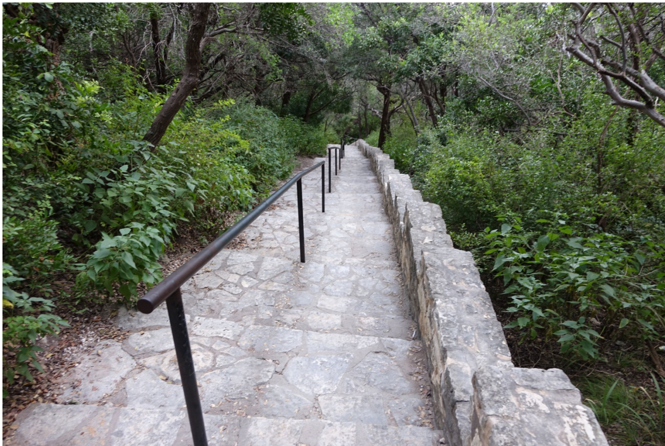
Photo 4 Staircase, looking down from summit Camera facing east
