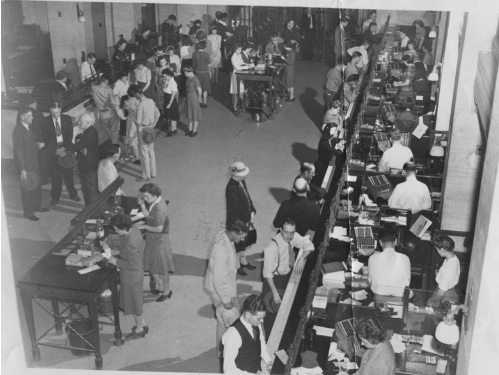
Figures 11 and 12: First National Bank of Port Arthur interior, c. 1943.
