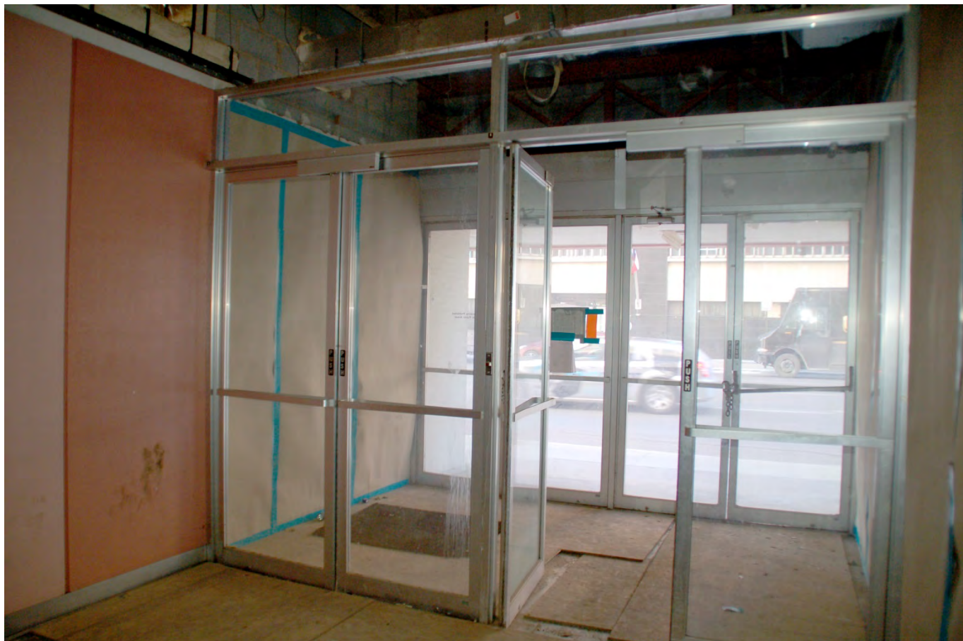
# 10 - Interior view, airlock vestibule, main building entrance, camera facing south
