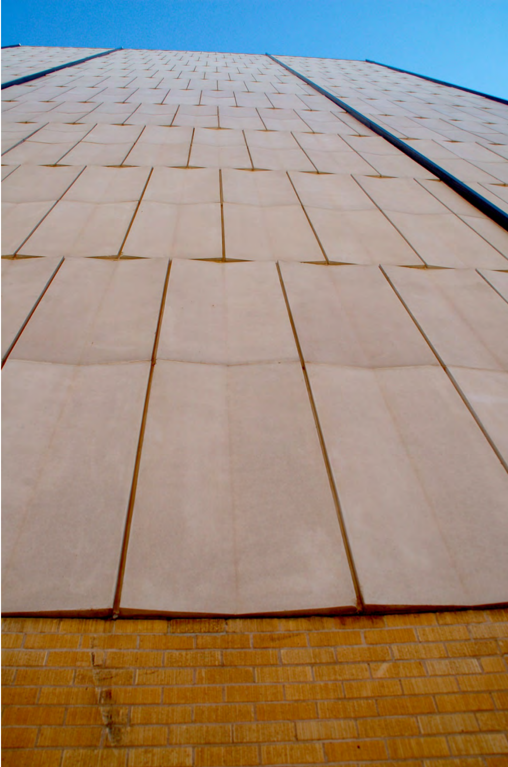
# 9 - Detail view, east elevation, cast stone panels, camera facing west
