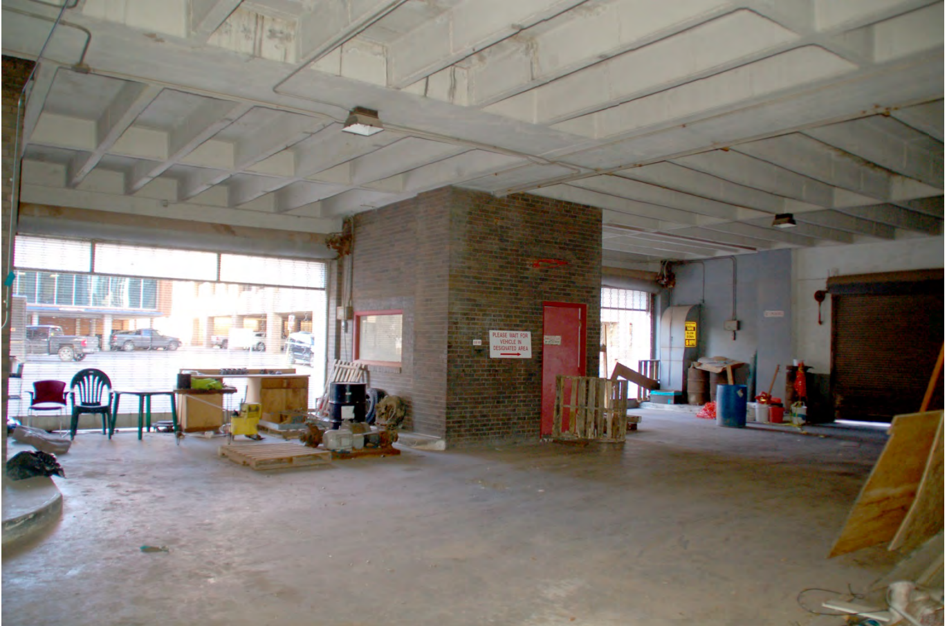
# 15 - Interior view, first-floor vehicular building entrance, camera facing southwest
