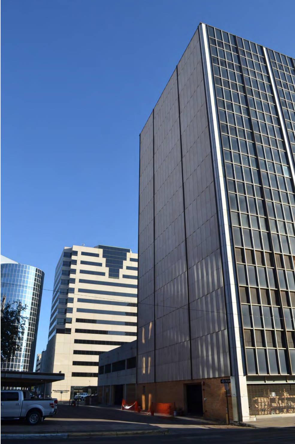
# 6 - Exterior view, west elevation, camera facing northeast
