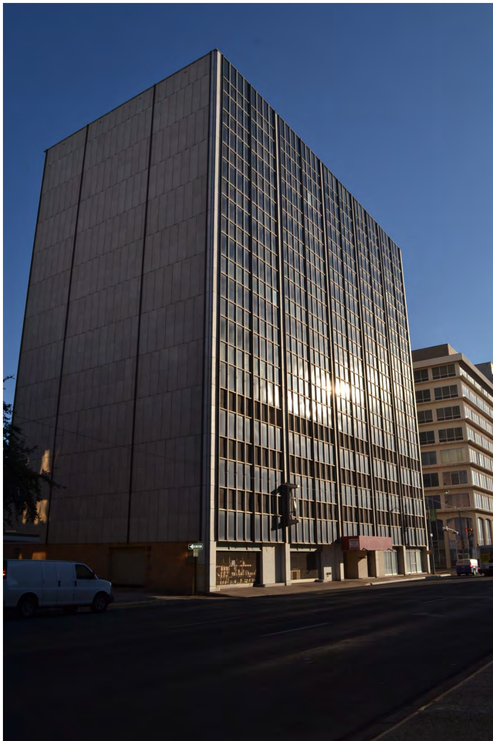
# 7 - Exterior view, south and west elevations, camera facing northeast
