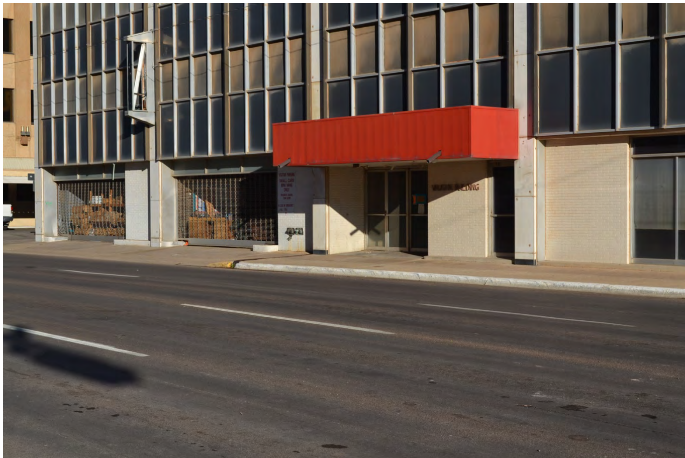
# 8 - Detail view, south elevation, main building pedestrian and garage entrances, camera facing northwest
