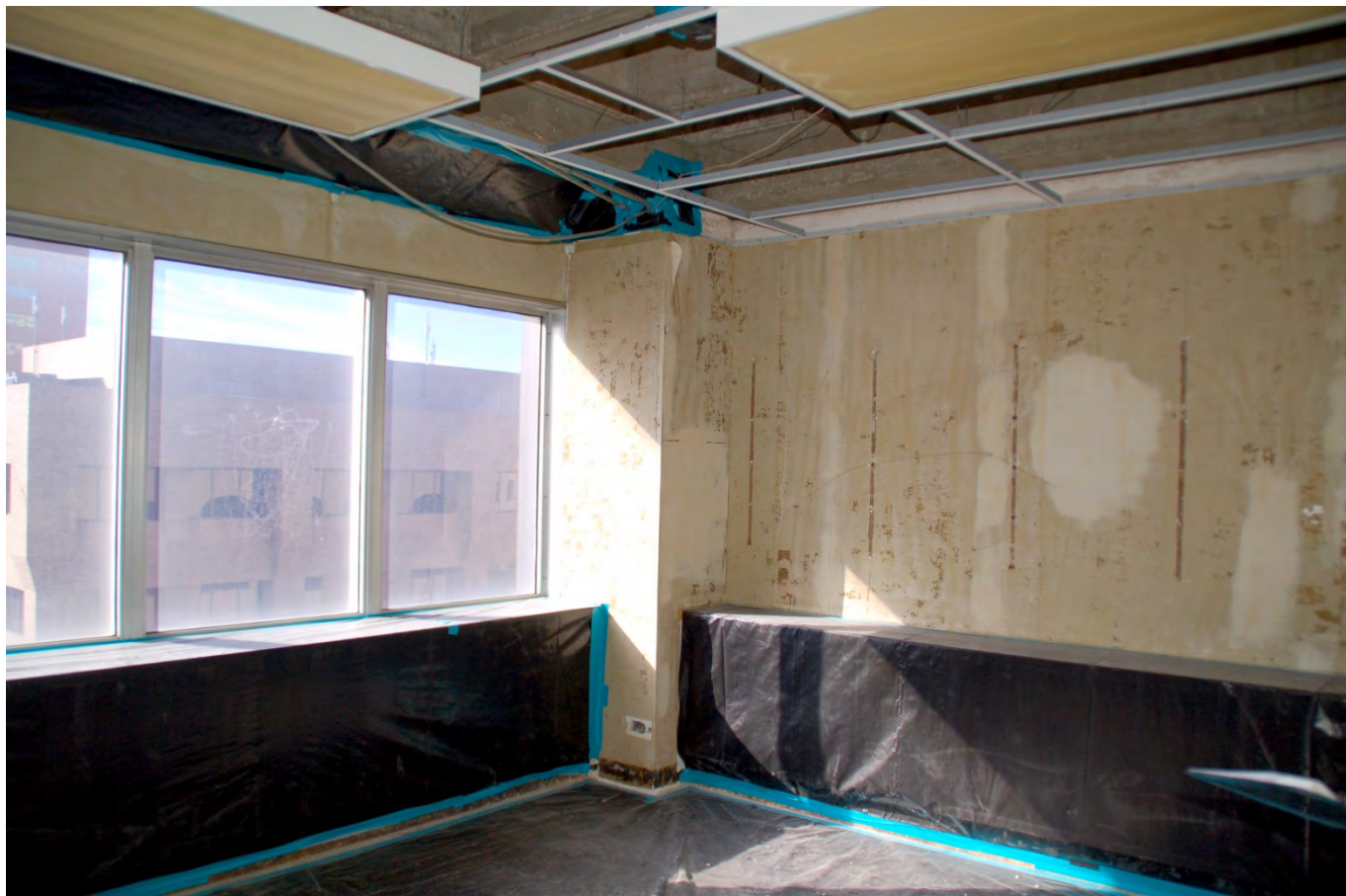
# 18 - Interior view, typical upper-floor tenant space (sixth floor), camera facing southwest
