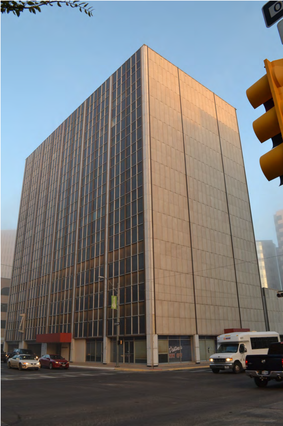
# 2 - Exterior view, south and east elevations, camera facing northwest
