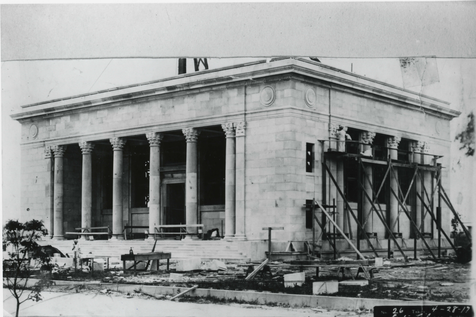
Mrs. Delora Gates, wife of the late John W. Gates, donated to the City of Port Arthur a library building costing approximately $75,000.00, in 1917.
